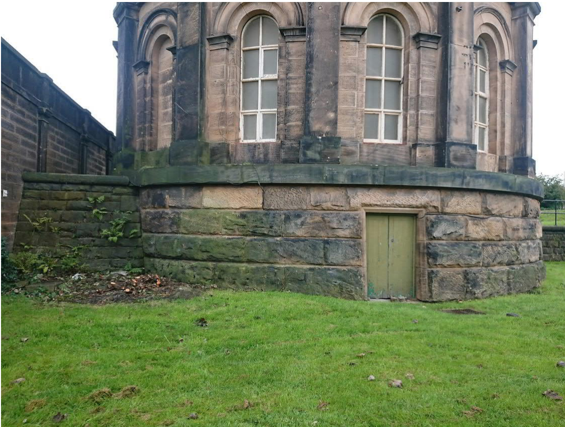
Figure 4: View of the eastern door and existing retaining wall
