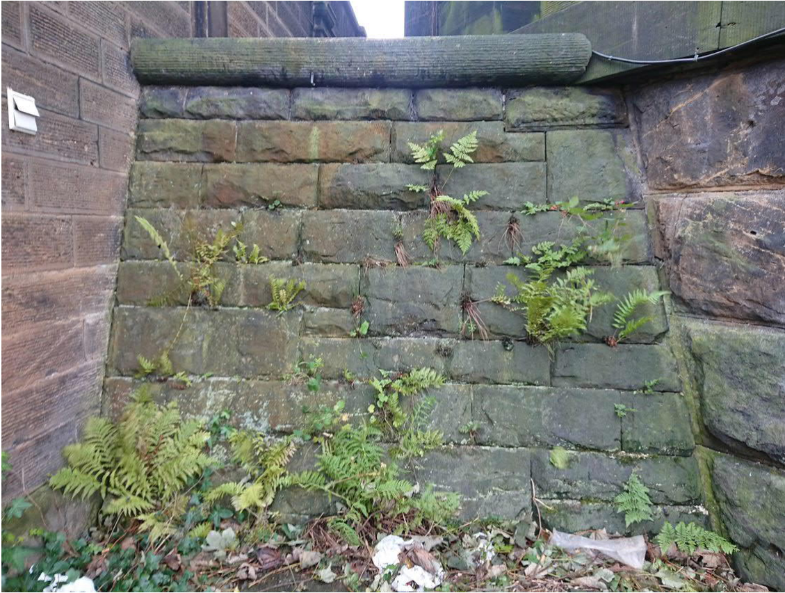
Figure 3: Existing retaining wall as viewed from the eastern side
