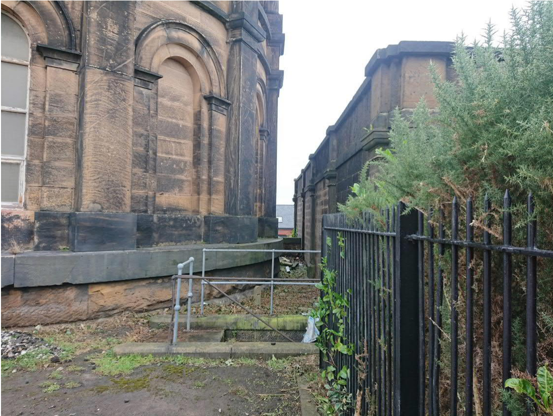
Figure 2: View from the west showing the existing steps and retaining wall
