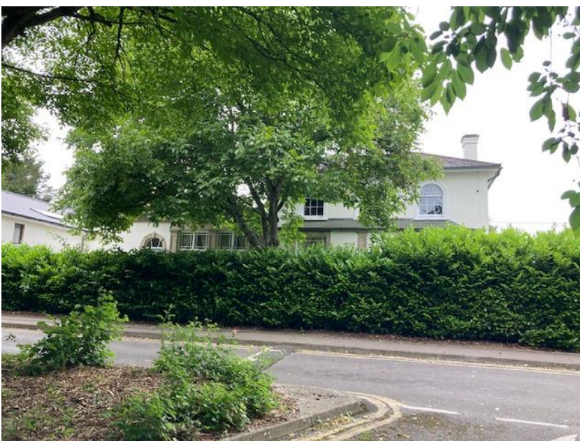
Photo 5.1: Holgate House viewed from within the northern boundary of the site
