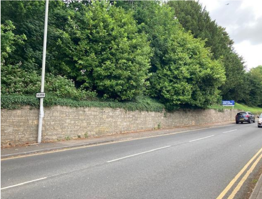
Photo 5.4: View from Number 30 looking towards the site, viewed from the north-west
