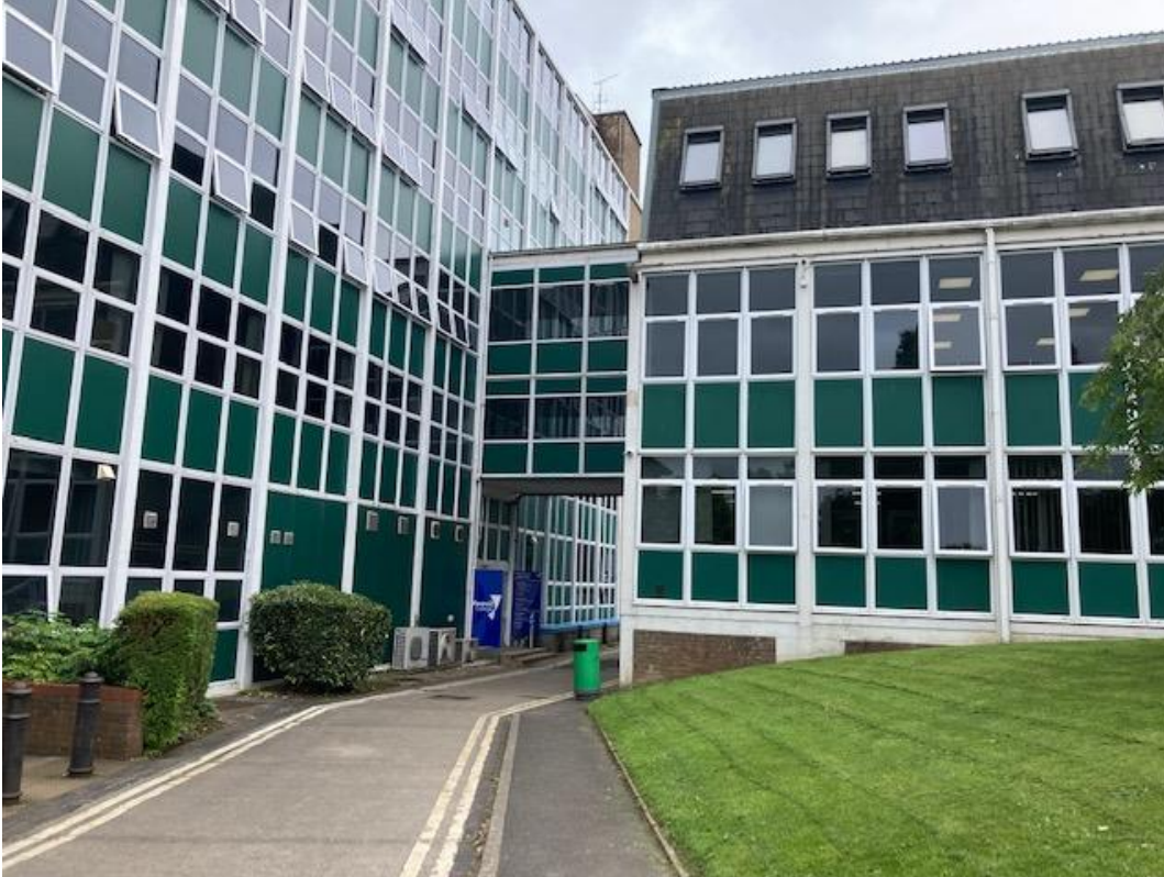
Photo 4.5: Kingston Building (FEAM block), looking west
