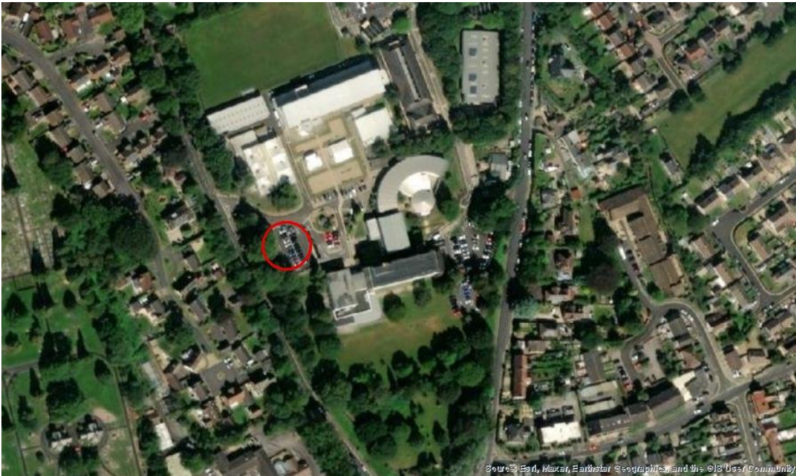
Photo 5.7: Aerial imagery showing the car park where Hollands House was formerly located
