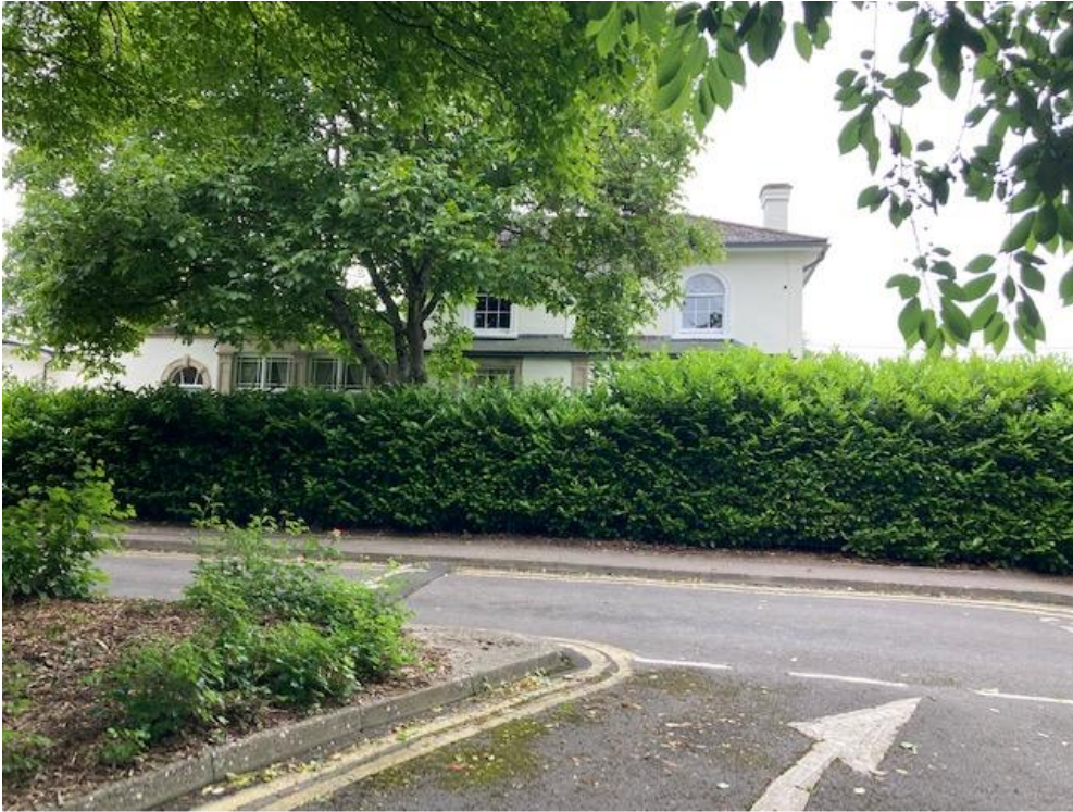
Photo 4.2: Holgate House, viewed from the site looking north
