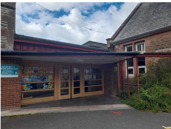
Figure 4.21: New main student entrance, facing west
