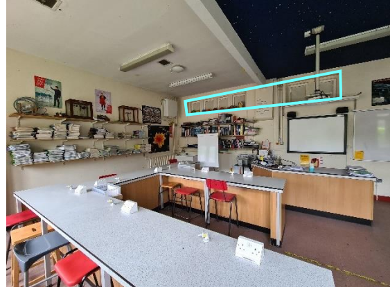
Figure 5.55: Former windows in the 1935-7 Science Building
