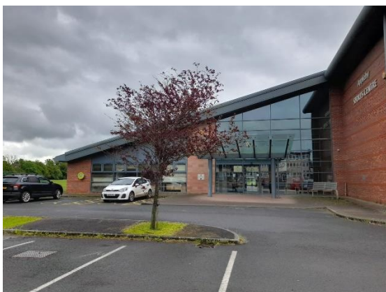
Figure 4.26: Sports Centre entrance, facing south
