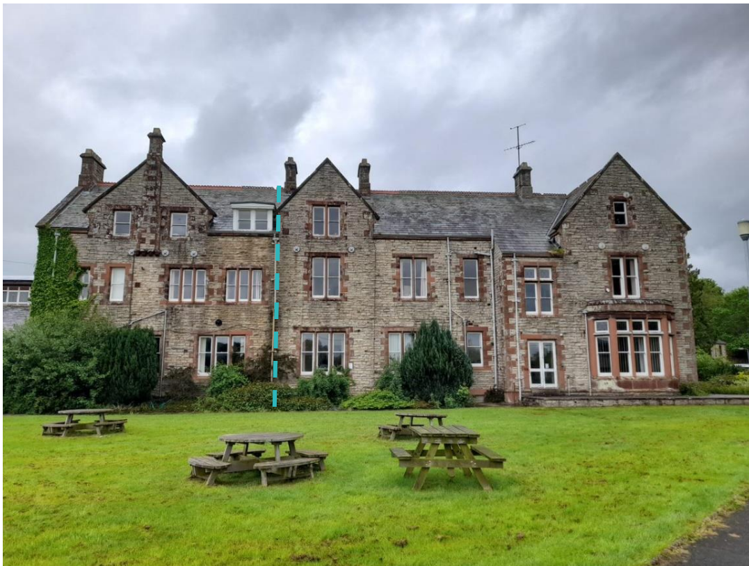
Figure 5.7: Southern elevation of the Original School Building. The blue line denotes the stylistic shift on this façade.
