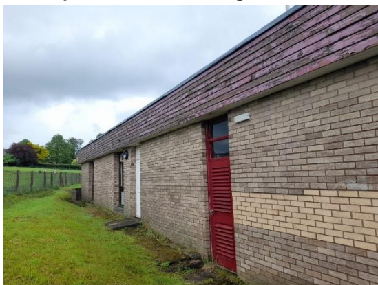
Figure 5.90: Former Intake and Development Centre, facing north
