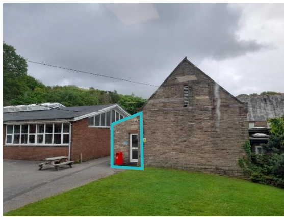
Figure 5.53: 1935-7 Science Building western elevation, facing east with the modern extension highlighted
