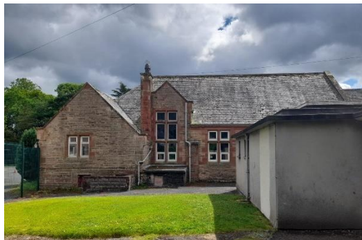
Figure 5.48: 1927 Science Building, facing south
