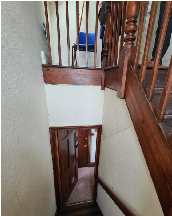
Figure 5.33: Second floor staircase, facing east
