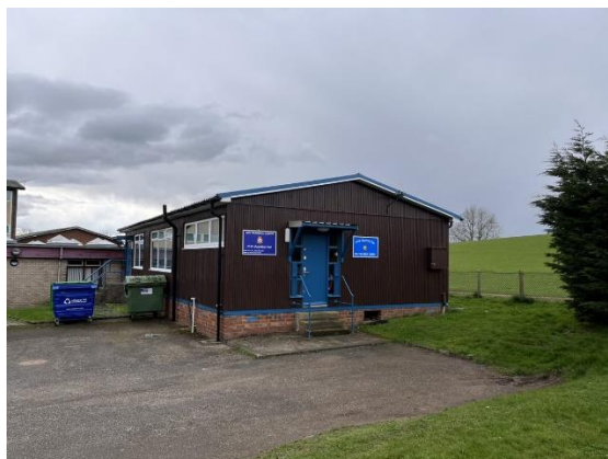
Figure 4.22: ATC hut, facing south.
