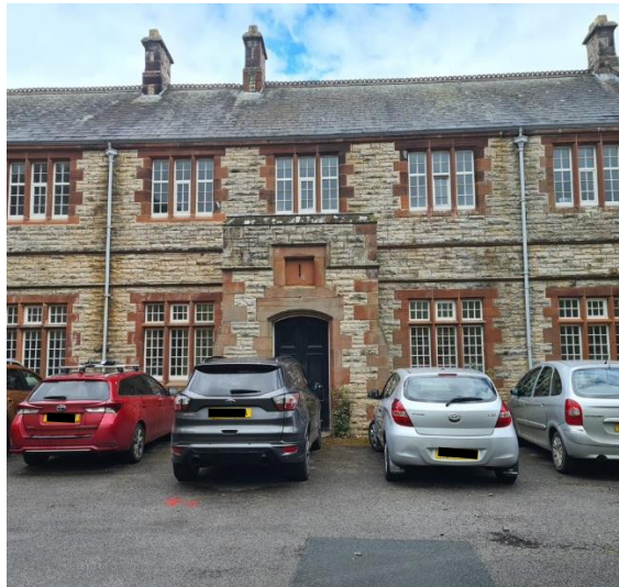
Figure 5.5: Former school main entrance
