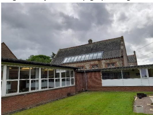
Figure 5.72: Science classrooms (left) and single storey corridor (right), facing south
