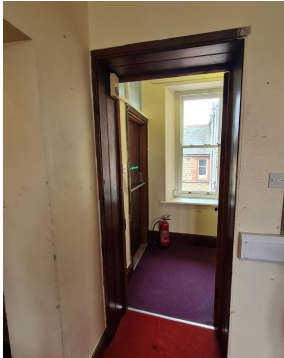
Figure 5.34: Fire door access to stairs, facing north
