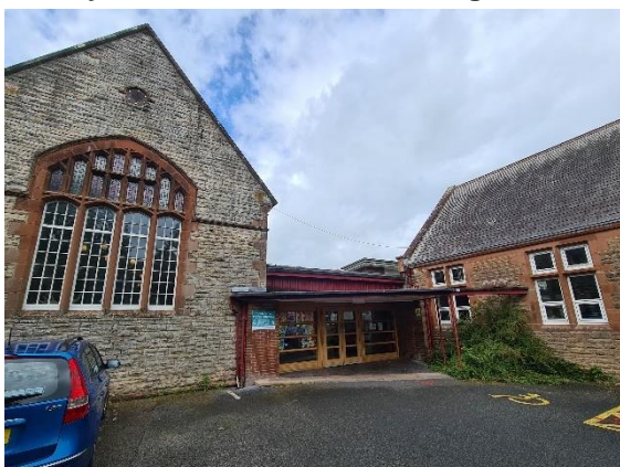
Figure 5.70: Modern entrance between the Library and 1927 Science Building
