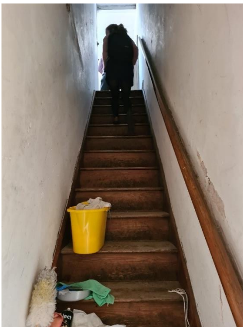
Figure 5.23: Second floor staircase
