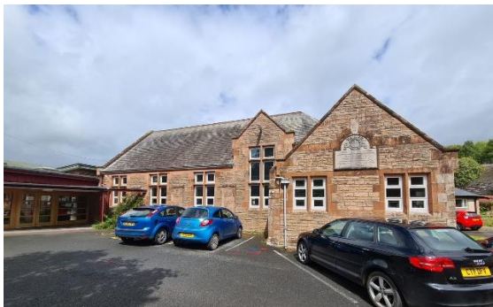
Figure 5.47: 1927 Science Building, facing north
