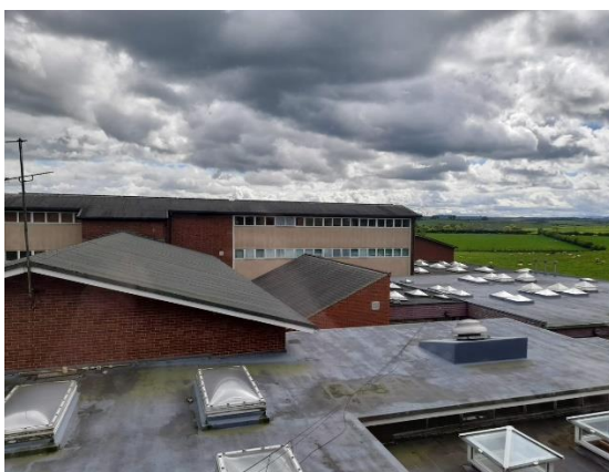
Figure 5.77: Rear of the 1962 block, facing south
