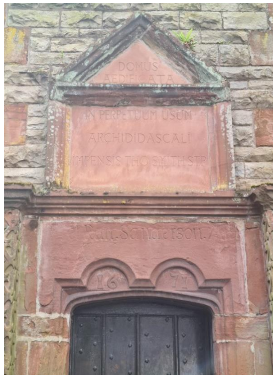
Figure 4.5: Plaques above the door from the former Headmaster’s House
