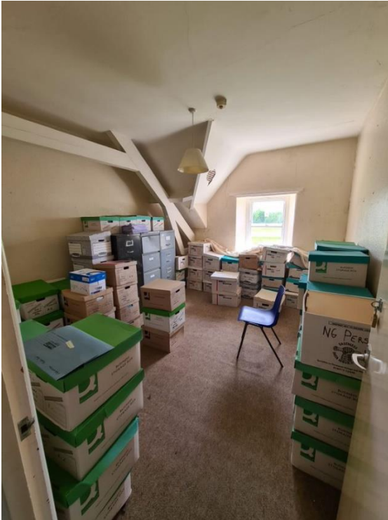
Figure 4.28: Second floor room now used for storage within the former Boarding House within the Original School Building
