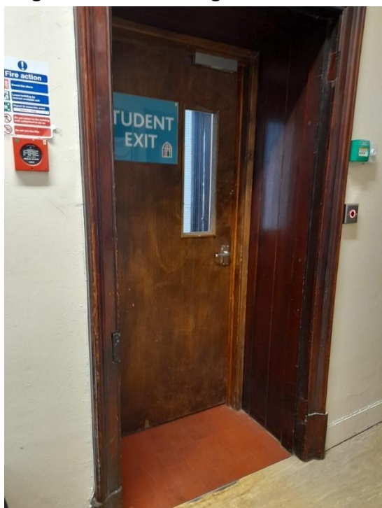
Figure 5.26: Access into porch from Original School Building corridor
