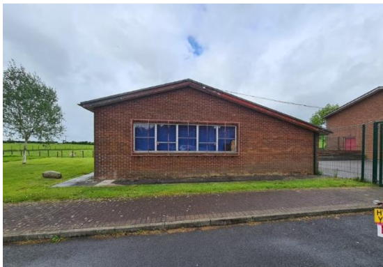
Figure 5.75: Music block, facing west
