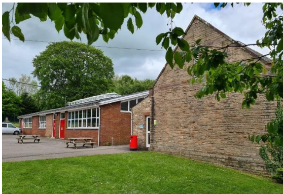
Figure 5.74: DT block visible beyond the 1935-7 Science Building
