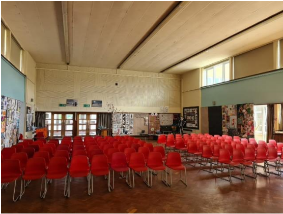
Figure 5.65: Main Assembly Hall facing south
