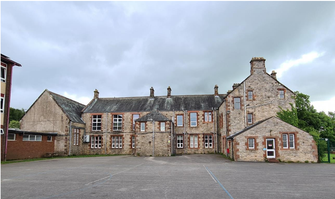
Figure 5.8: Western elevation of the Original School Building
