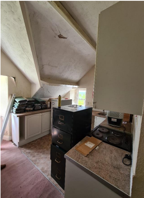
Figure 5.35: Former second floor flat kitchen, facing south-west
