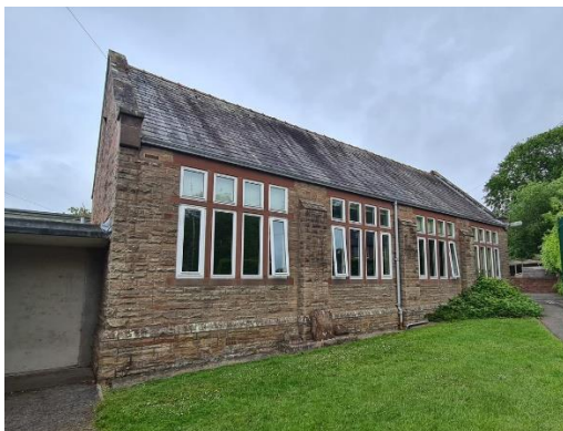
Figure 4.9: 1935-7 Science Building, from the east
