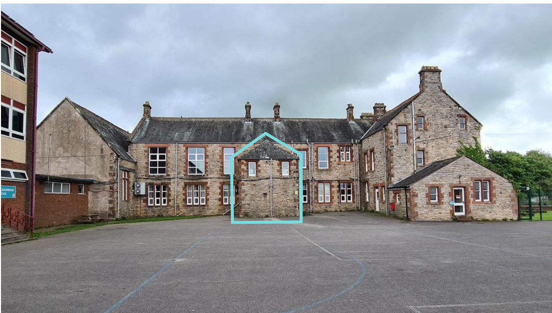
Figure 4.7: Appleby Grammar School from the west. The central protruding bay (outlined in blue) accommodates the main staircase.
