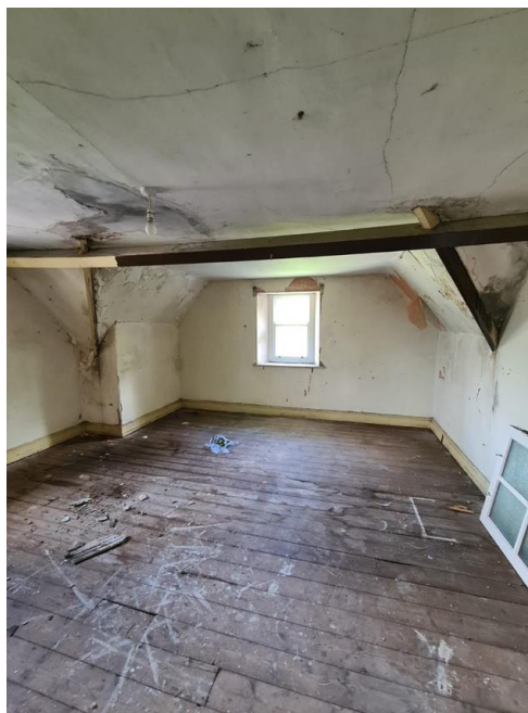
Figure 5.24: Former second floor bedroom, now disused, facing south.
