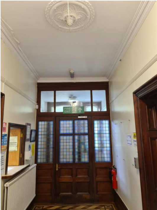
Figure 5.10: Front door screen, facing east
