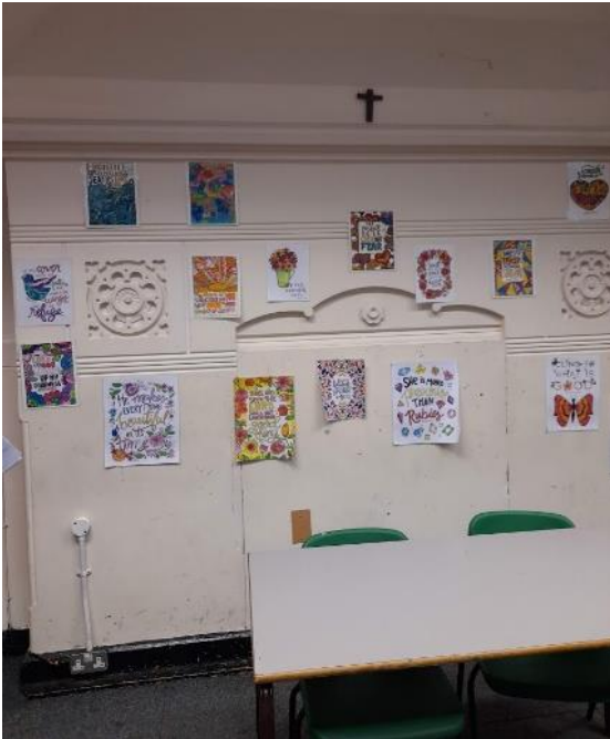
Figure 5.49: Infilled fireplace in room 94 (EFAA).
