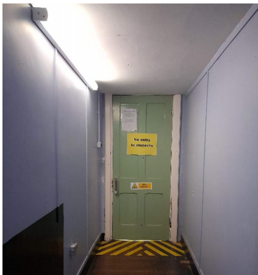
Figure 5.109: Corridor through the eaves (EFAA).
