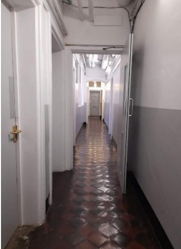
Figure 5.56: North-western corridor, facing south-east (EFAA).
