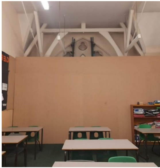
Figure 5.112: Boards at the end of classroom 205 (EFAA).
