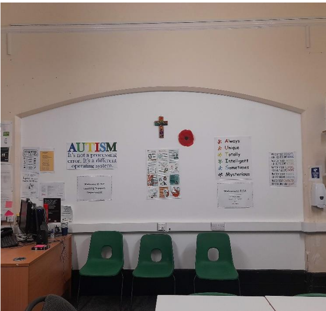
Figure 5.81: The now-infilled archway that formerly joined Room 118 on Figure 5.76 (EFAA).
