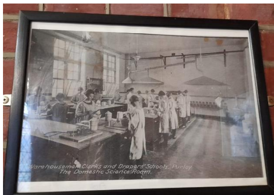
Figure 4.18: Domestic Science Classroom, c. 1930 located within EFAC
