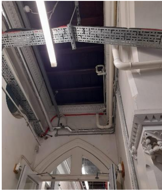
Figure 5.41: Ceiling of corridor (EFAA).
