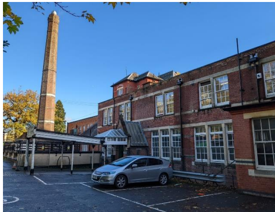
Figure 5.13: North-western elevation of EFAA, facing north to the chimney.
