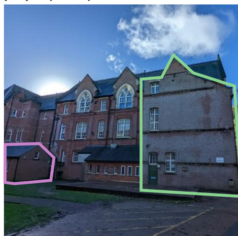
Figure 5.17: North-western elevation of the 1903 wing, with the stair tower outlined in green and the chapel in purple (EFAA)
