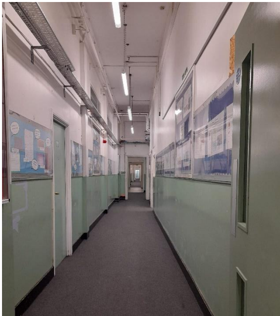
Figure 5.86: Corridor, facing south-west (EFAA).
