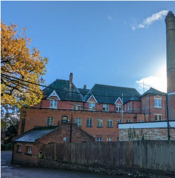
Figure 5.10: Northern end of the north-western elevation of EFAA
