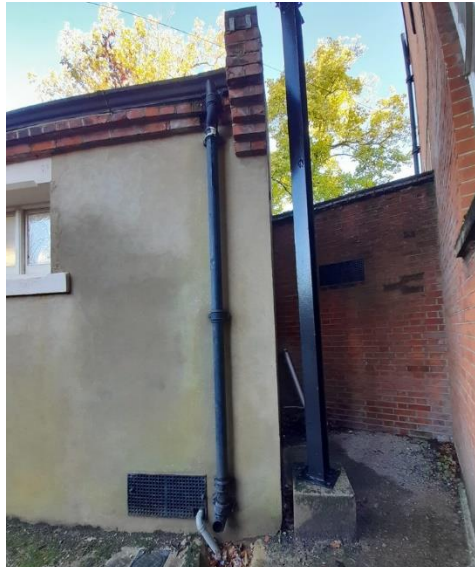
Figure 5.11: Corridor connecting to small rectangular toilet block (EFAA)
