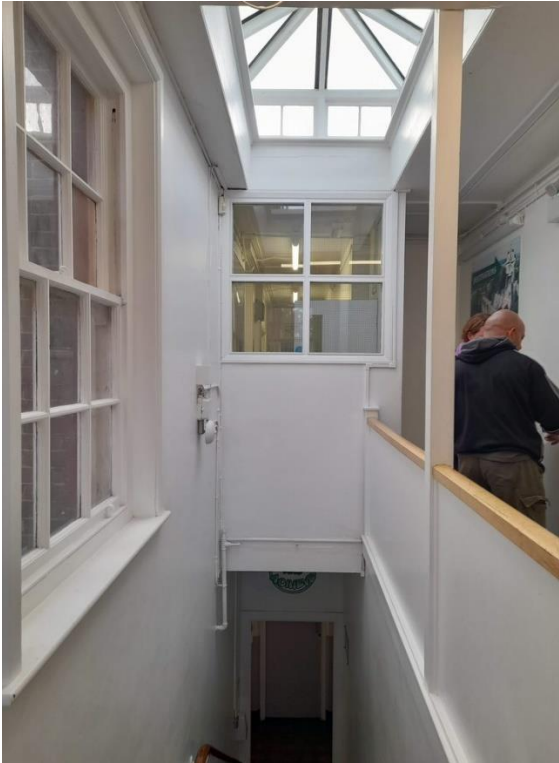
Figure 5.83: Stairwell up to the Sixth Form Centre (EFAA).
