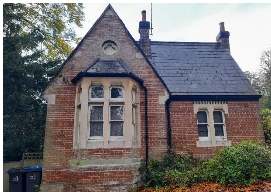
Figure 4.6: Lodge, facing west
