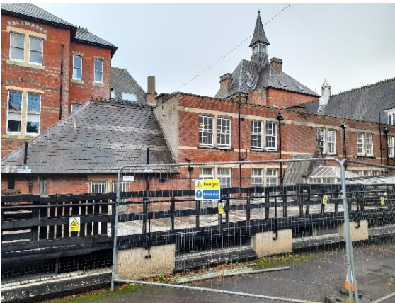
Figure 5.12: North-western elevation of EFAA, facing south-east.
