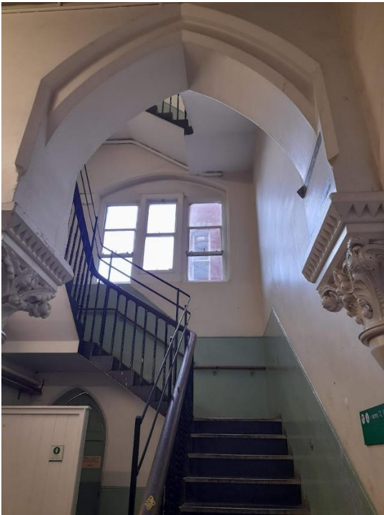
Figure 5.42: Central, wider staircase (EFAA).
