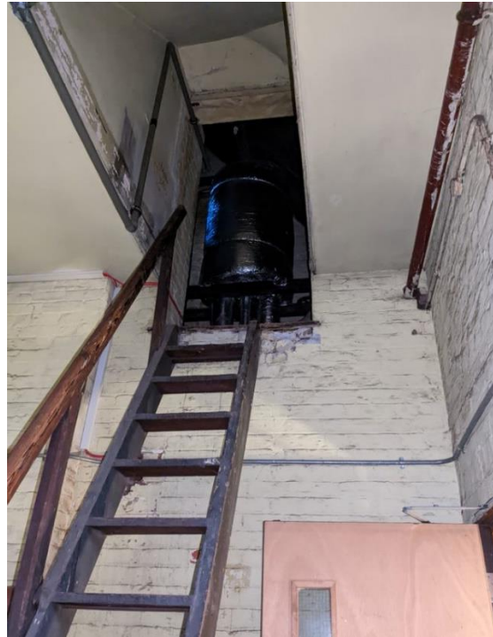
Figure 5.128: Ladder to bell tower (EFAA).
