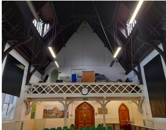
Figure 5.36: Main Hall, facing south-east (EFAA).
