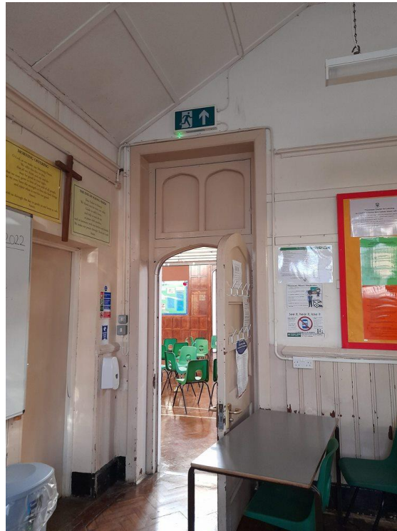
Figure 5.141: Door from classroom back to hall (EFAB).
