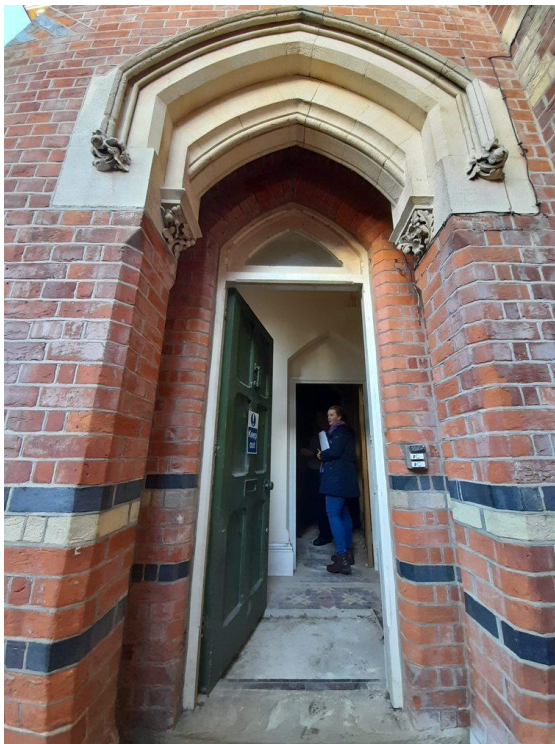
Figure 5.172: Main entrance to the House.
