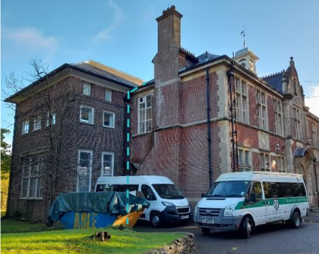
Figure 5.145: North-western elevation of EFAC. The turquoise line denotes the original extent of the block (right) and the extension (left).
