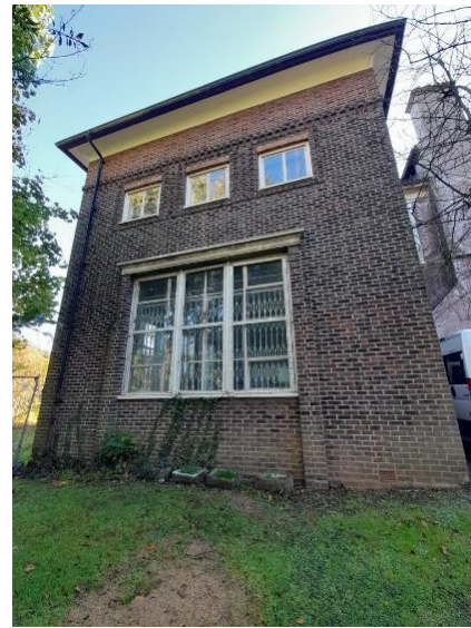
Figure 5.149: North-western elevation of EFAC.
