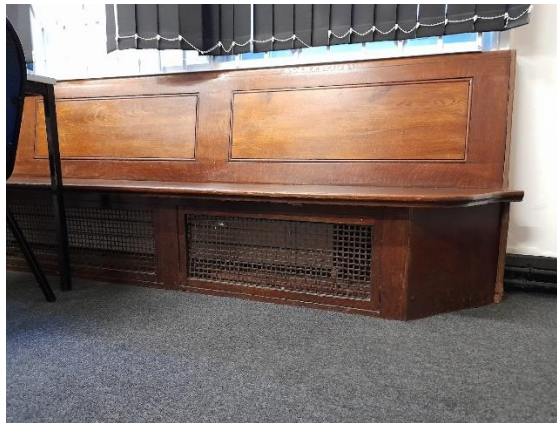
Figure 5.68: Fitted bench seating over the library radiators (EFAA).
