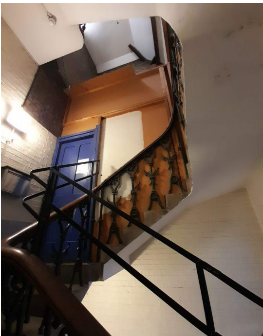
Figure 5.125: Staircase to third floor with partition (EFAA).
