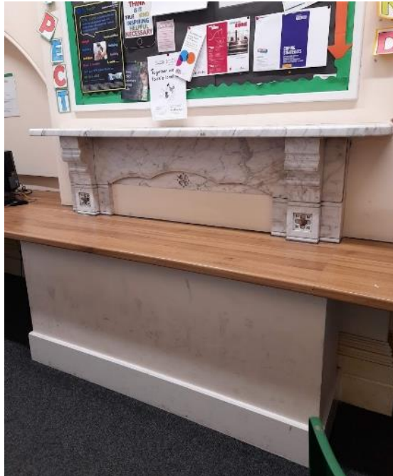
Figure 5.50: Infilled fireplace bisected by modern desk in room 97 (EFAA).
