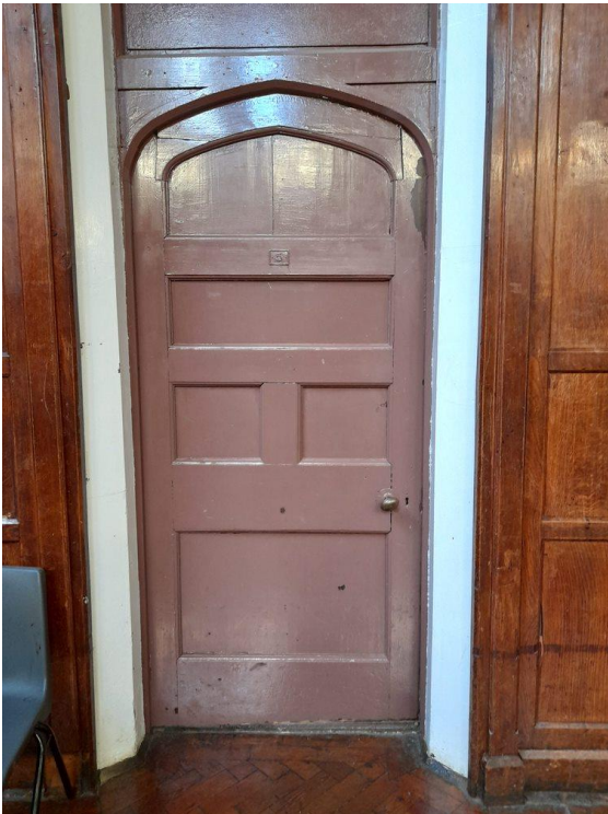
Figure 5.140: Door from the hall to classroom (EFAB).
