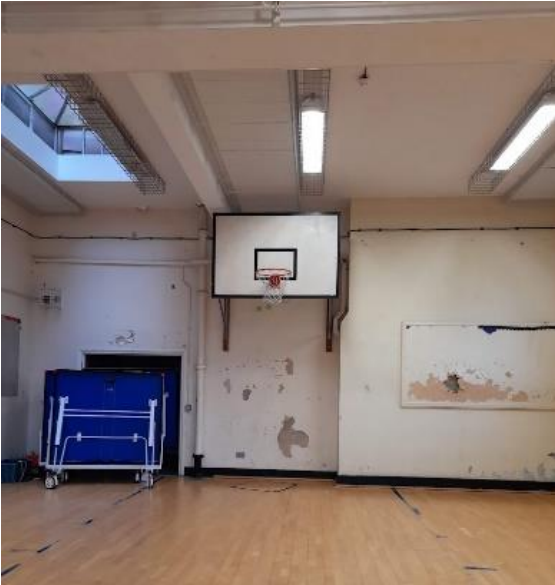
Figure 5.61: Gym, facing south-west (EFAA).
