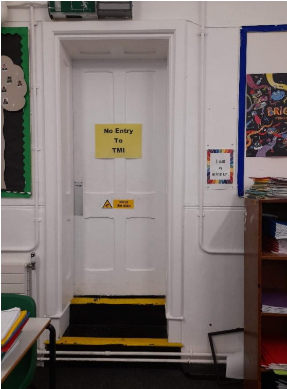
Figure 5.116: Door to the corridor through the eaves (EFAA).
