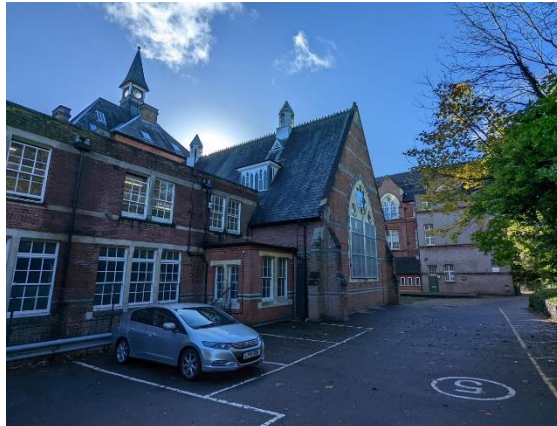
Figure 5.15: North-western elevation of EFAA, facing south.
