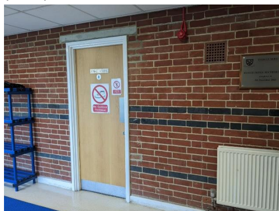
Figure 5.171: Internal view of the area with the pitched roof shown on Figure 5.168 (EFAE).
