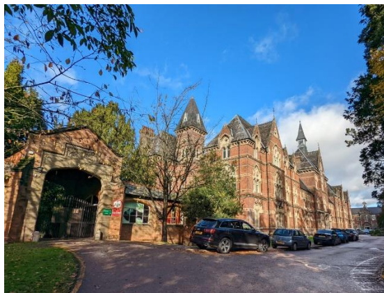
Figure 5.6: Southern end of the eastern elevation of EFAA, where it adjoins EFAB
