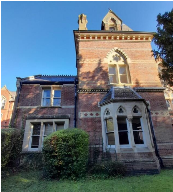
Figure 5.174: The south-western elevation of the House. The lower bay on the left is a later extension.
