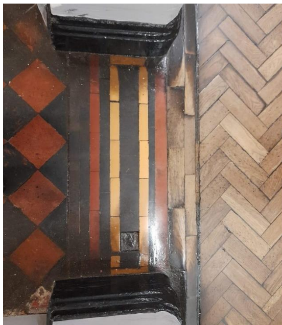
Figure 5.52: Encaustic tiles and parquet flooring (EFAA).
