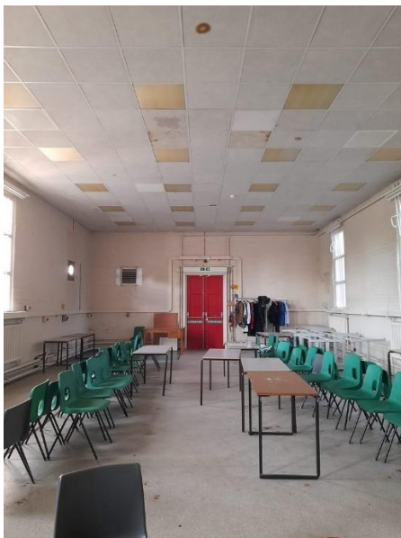
Figure 5.161: Room 2 in EFAD as labelled on Figure 5.160.
