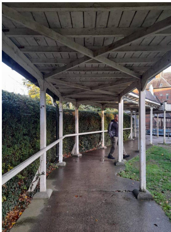
Figure 4.16: Covered walkway that formerly connected to the Sanitorium
