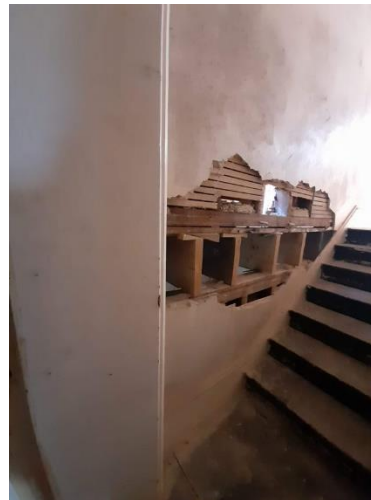
Figure 5.181: Area of missing plaster within the House.
