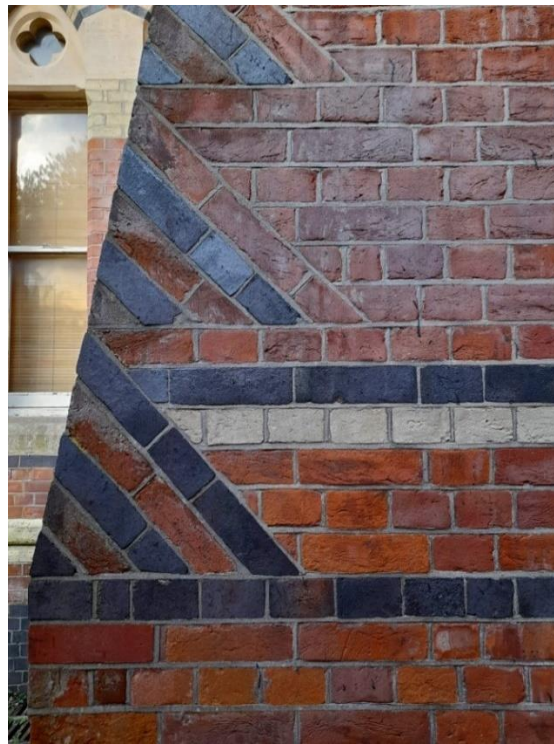
Figure 5.173: Buttress with polychromatic brickwork on the exterior of the House.
