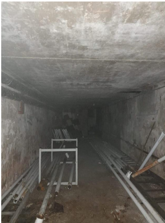
Figure 4.23: Interior of the air raid shelter
