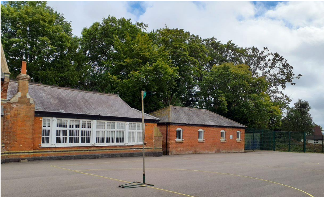
Figure 5.159: The north-western elevations of EFAD and EFAF.
