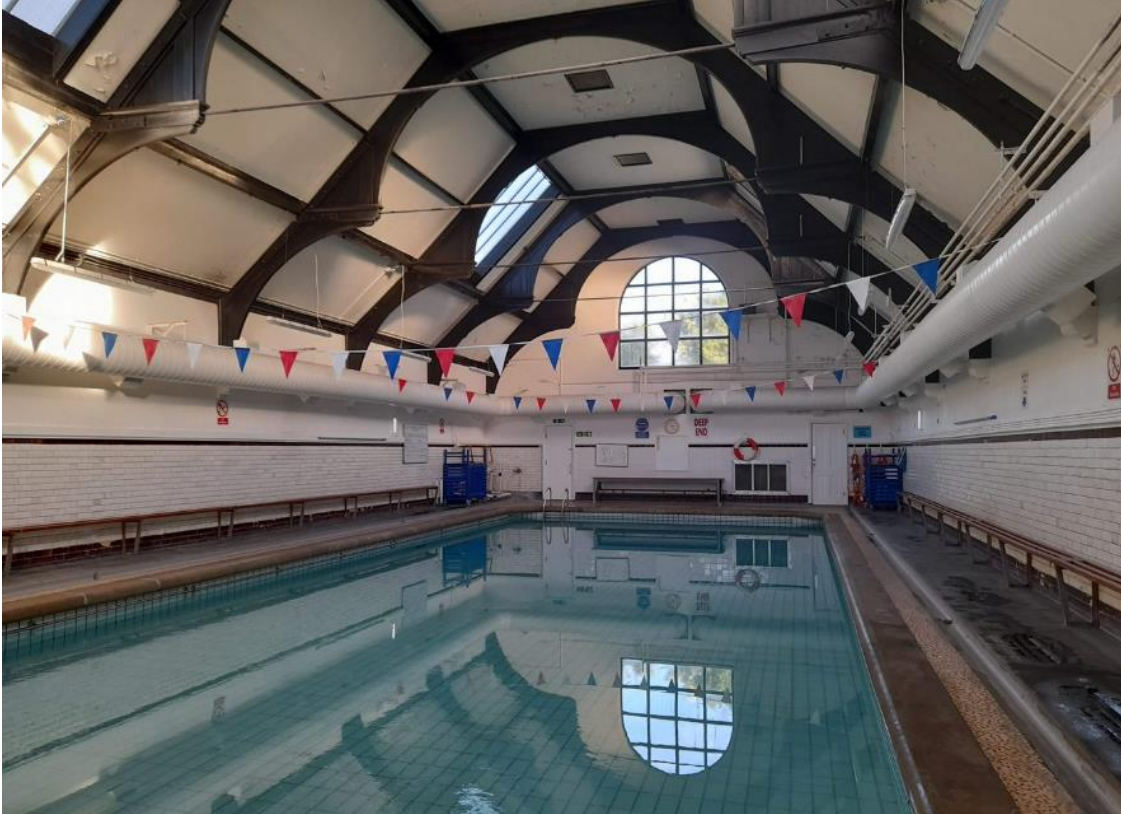
Figure 5.169: Swimming pool in EFAE, facing east.
