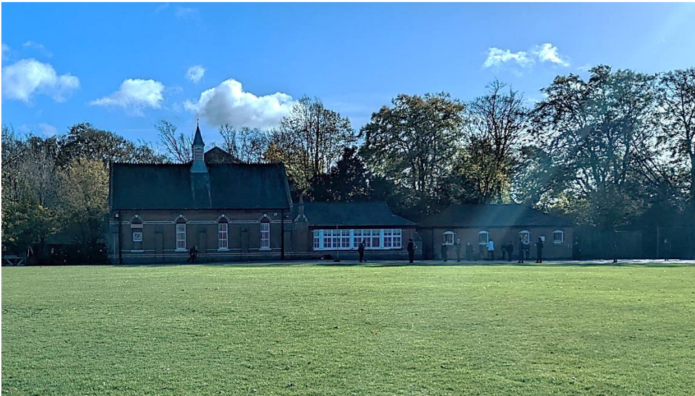
Figure 5.156: The north-western elevations of EFAD and EFAF.
