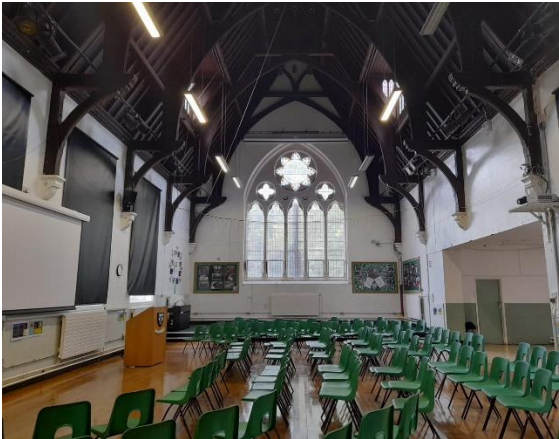
Figure 5.35: Main Hall, facing north-west (EFAA).
