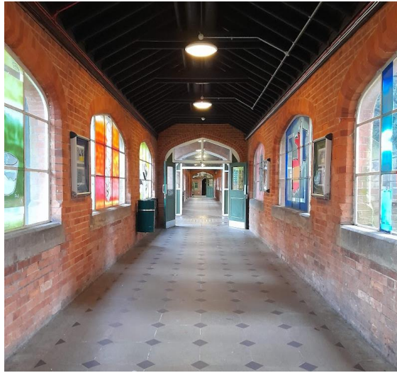
Figure 5.70: The cloister, facing south-west (EFAA).
