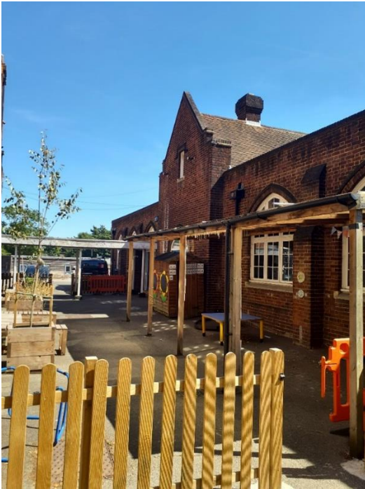
Photo 4.11: Annexe to Harris Kent House (MM13), looking south-east
