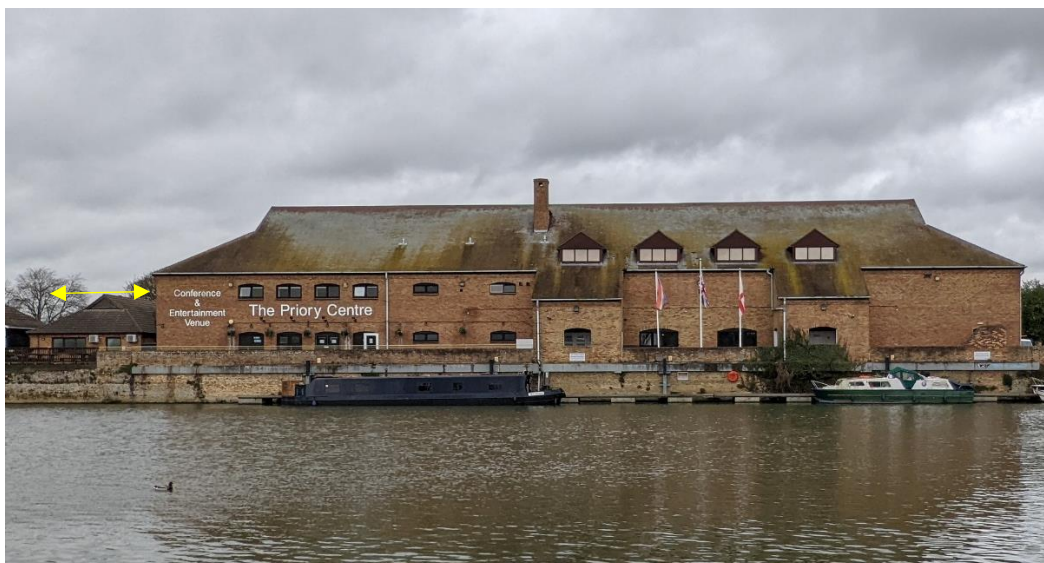
Figure 4.14: Proposed development area 3, including the riverside wall, as viewed from the western bank of the River Great Ouse, proposed area of demolition indicated in yellow
