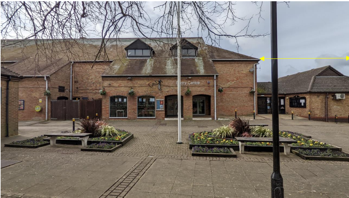
Figure 4.10: Northern end of the Priory Centre (proposed development area 3), as viewed from the east, proposed area of demolition indicated in yellow
