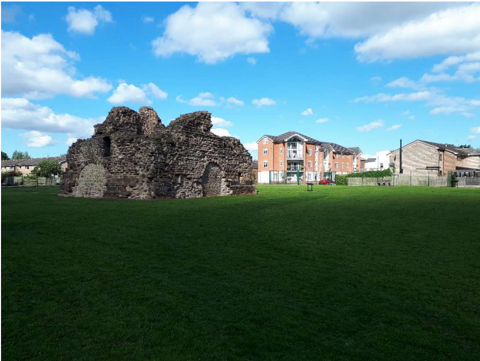
Photo 2: Radcliffe Tower. Facing North-west
