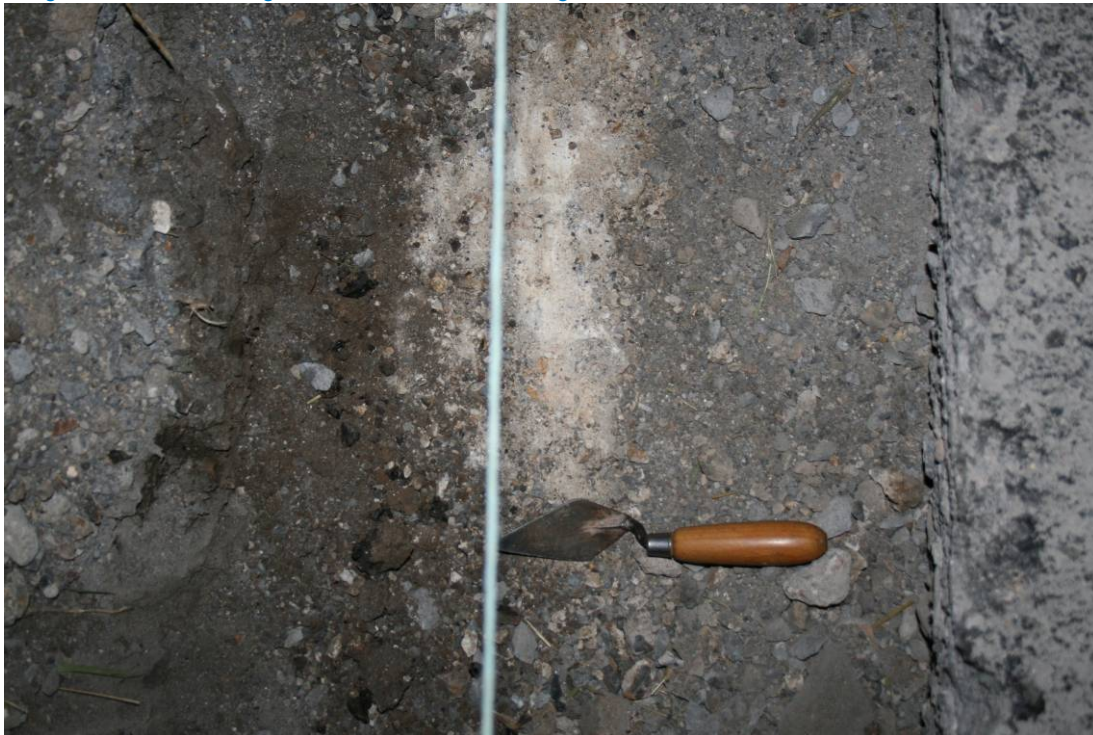
Image04, View of kerbing trench from above showing sub surface concrete and road material.
