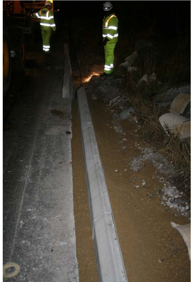
Image 02, New kerbing installed
