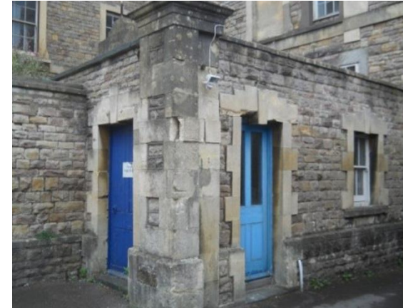
Photo 5.3: Original building adjacent to turret looking NW
