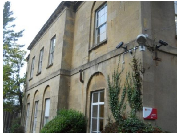
Photo 5.5: The original Westmead house looking NE
