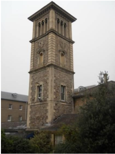
Photo 5.7: The Italianate tower looking NE
