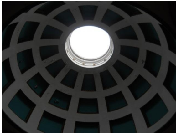
Photo 5.13: The dome roof in the chapel
