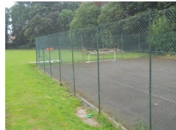
Photo 5.18: Old tennis courts looking west
