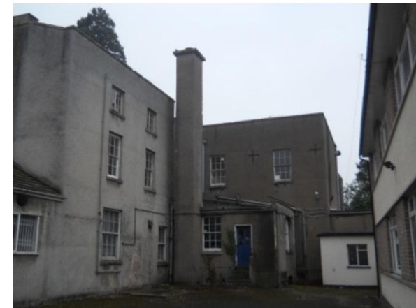
Photo 5.6: Westmead house from the rear looking West
