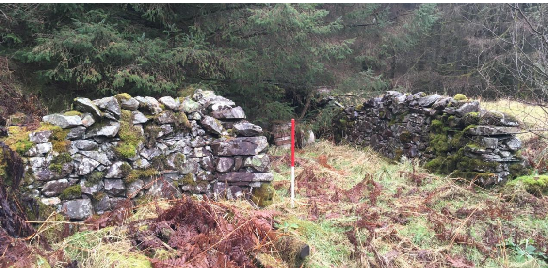
Photo 5.6: Detailed view looking west of the drystone structure
