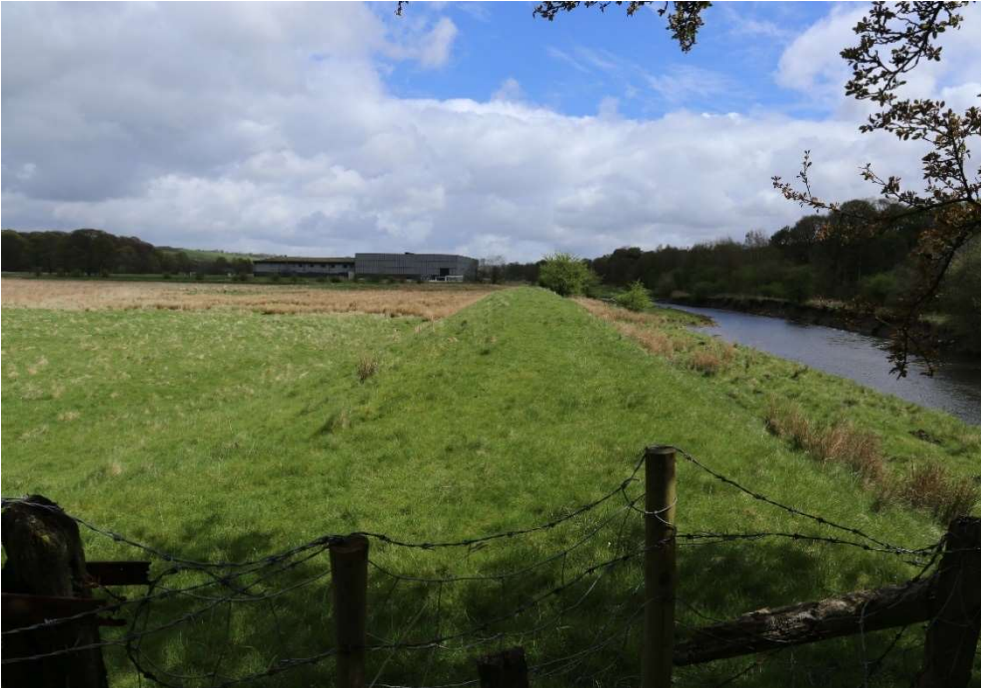
Photo 1: Overview of Embankment & Flood Storage Area (Works no.1)
