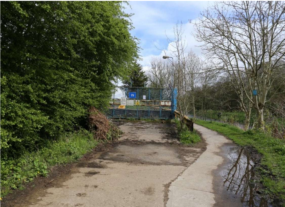
Photo 2 Rear Entrance to Industrial Unit (Works no. 2)
