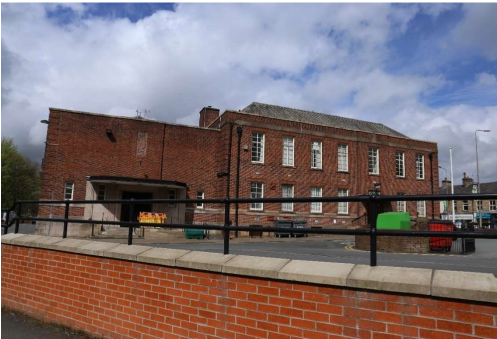
Photo 6: Existing Flood Defence Asset Protecting Town Hall (Works no. 3)
