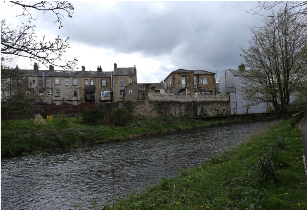
Photo 5: Flood Defence Wall near Padiham Bridge (Works no. 2)
