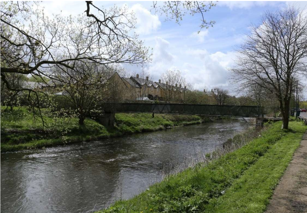
Figure 4: Pedestrian Footbridge (Works no.2)
