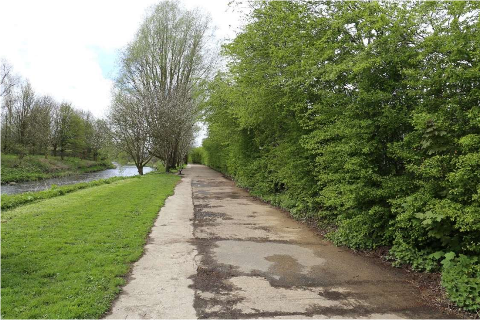
Photo 3: Hedgerow Adjacent to Current Flood Defence Wall (Works no.2)
