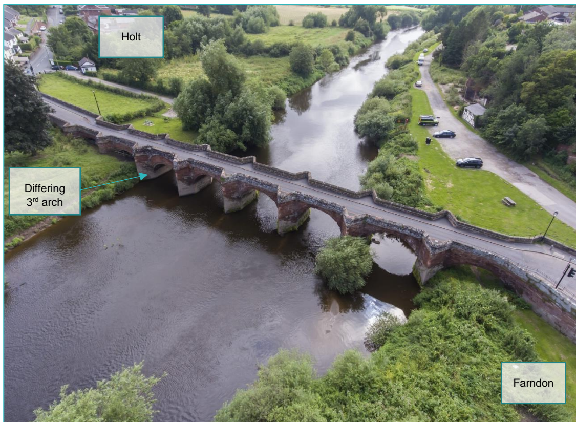
Figure 4.4: Farndon/Holt Bridge from above
