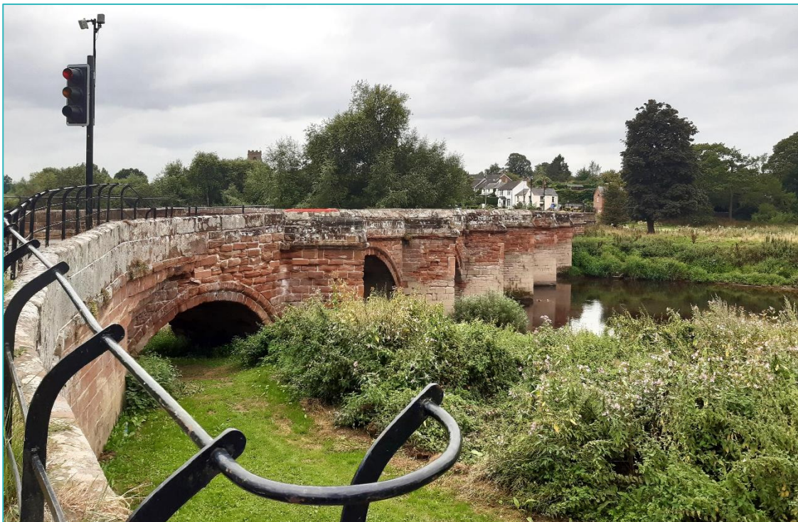
Figure 4.3: Farndon/Holt Bridge, looking towards Farndon
