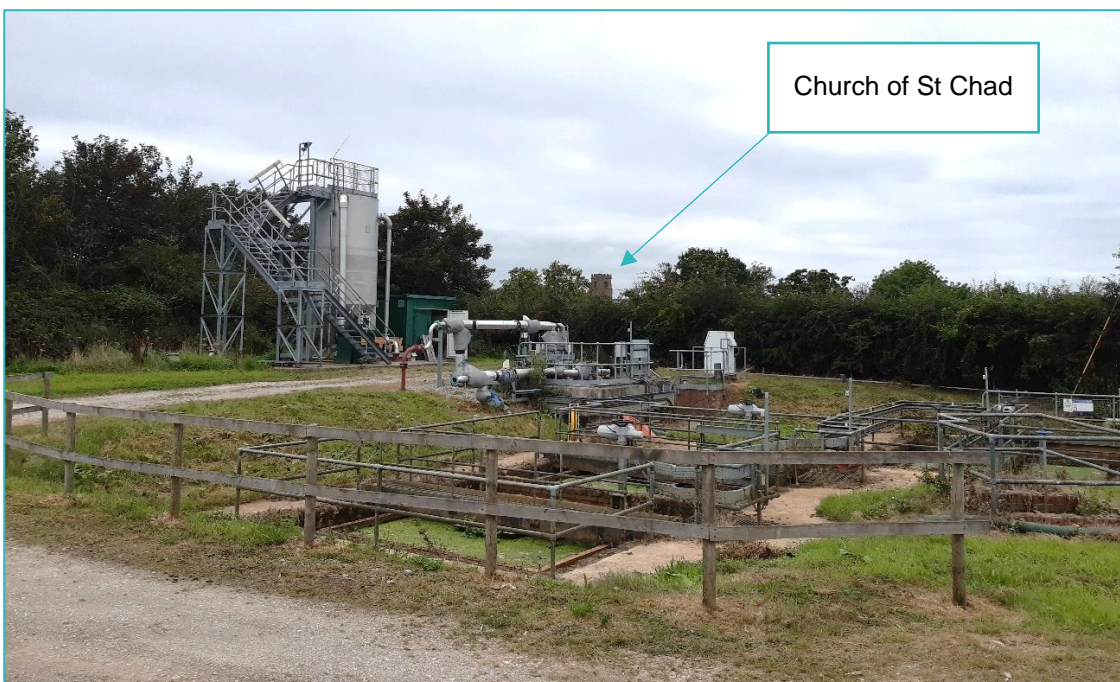
Figure 8.2: View towards Church of St Chad (Holt) from Farndon WwTW
