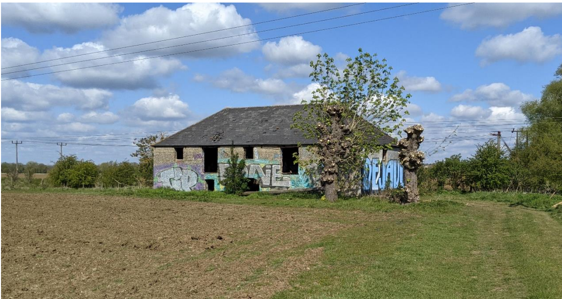
Figure 4.1: Exterior of the Concrete Barn from the south
