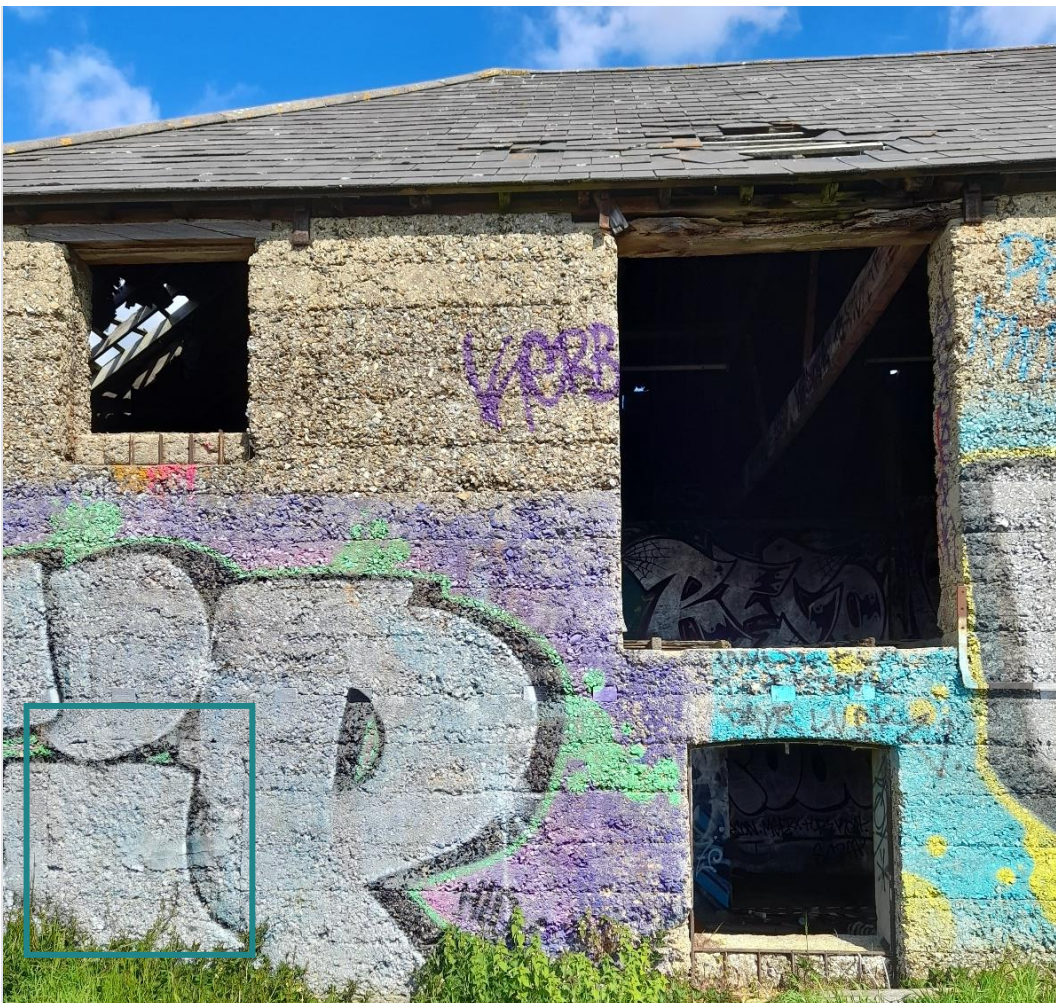
Figure 5.2: Southern elevation illustrating a blocked-up window (outlined in blue)
