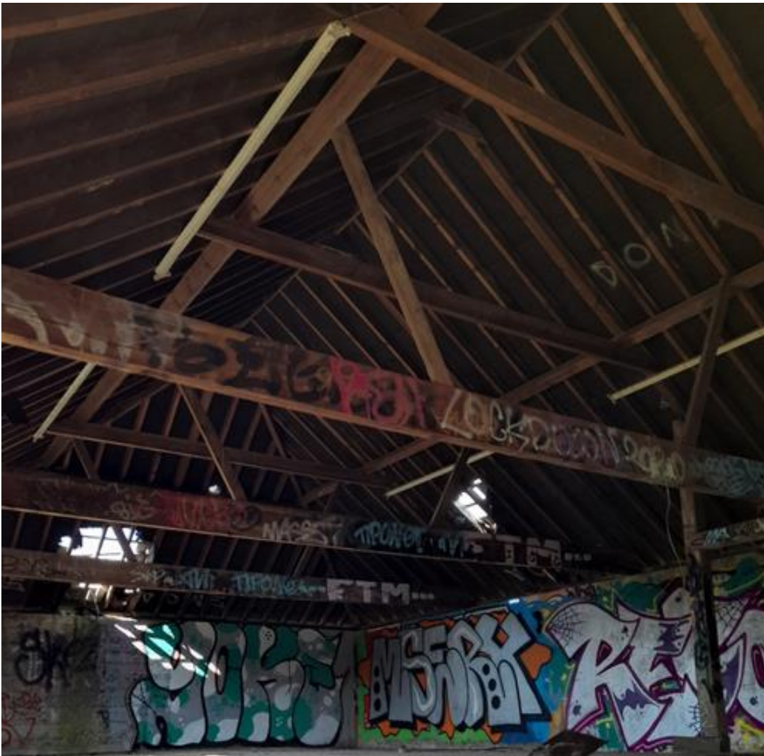
Figure 5.5: First floor showing timber roof trusses
