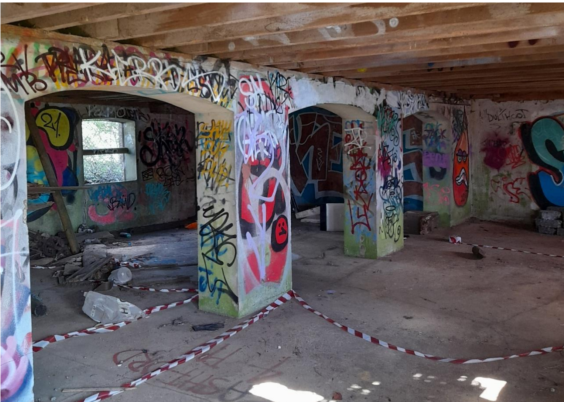
Figure 4.7: Concrete arcade supporting the first floor, facing north-east.
