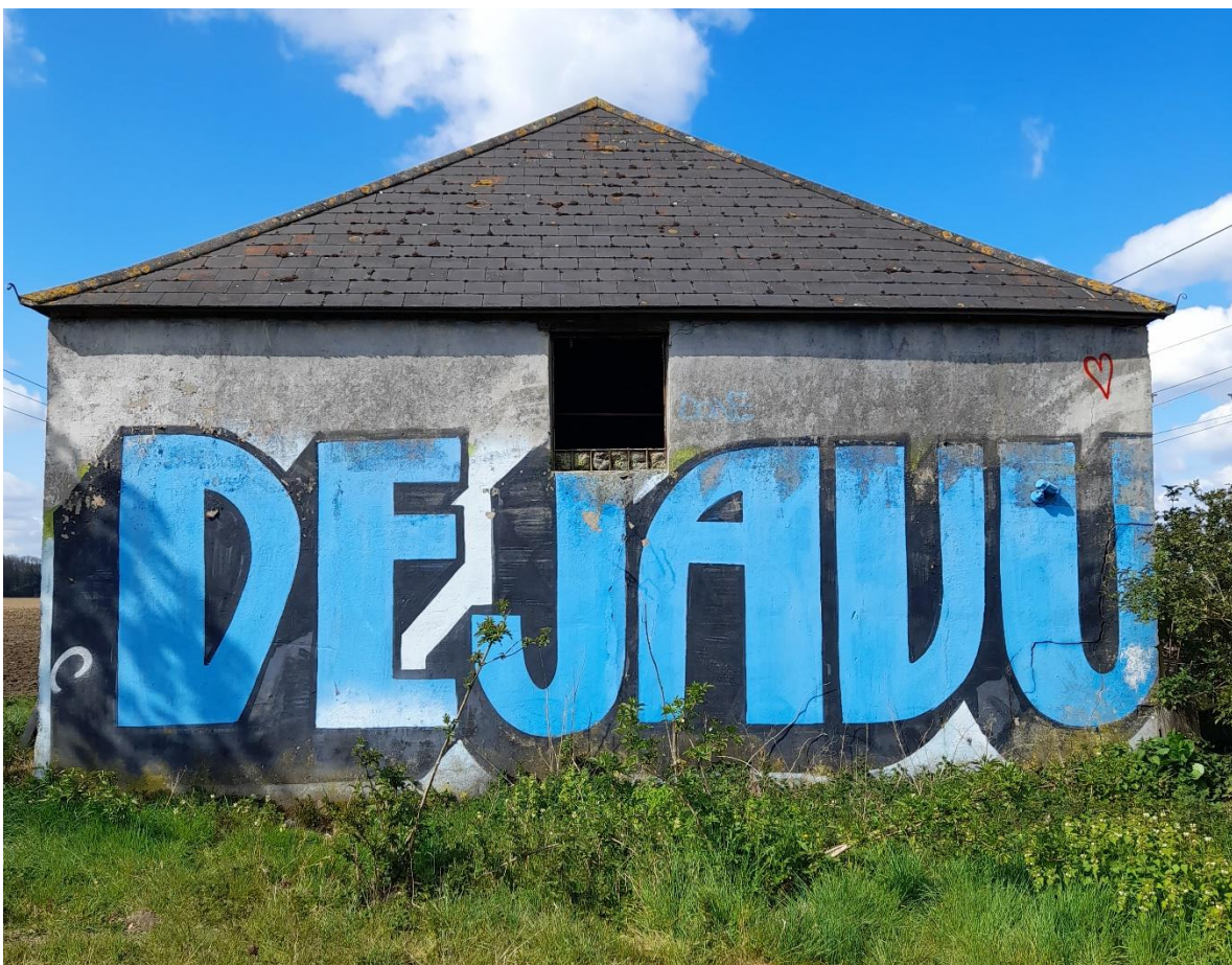
Figure 5.3: Eastern elevation of the Concrete Barn, featuring 'DE JAVU' graffiti.
