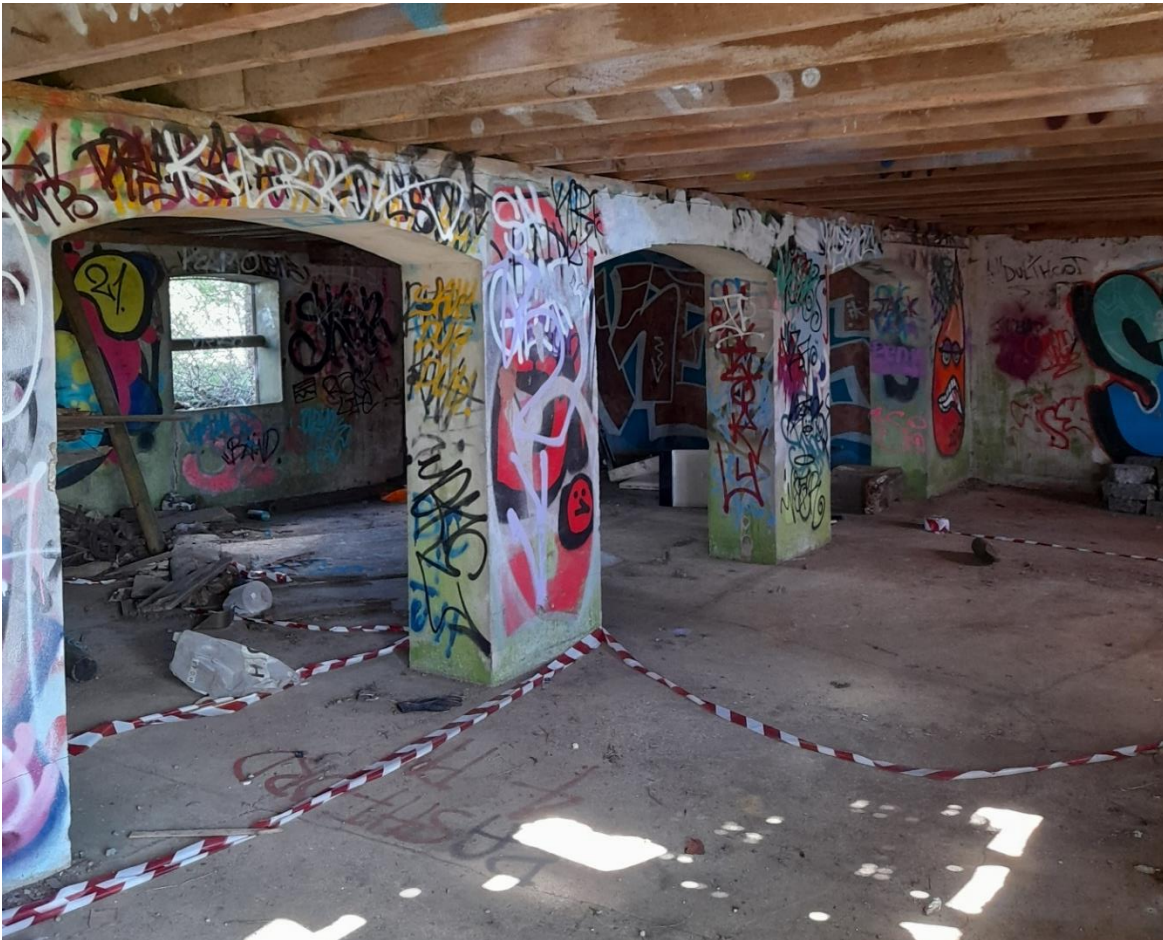
Figure 5.4: Ground floor arcade
