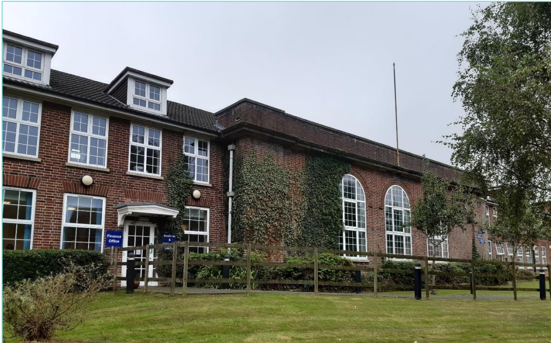
Figure 4.2: Eastern elevation of the main courtyard block
