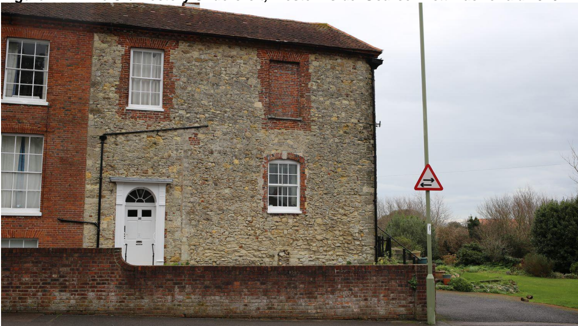
Figure 4.12: The Old Rectory Undercroft, Western side. Source: Mott MacDonald 2020.
