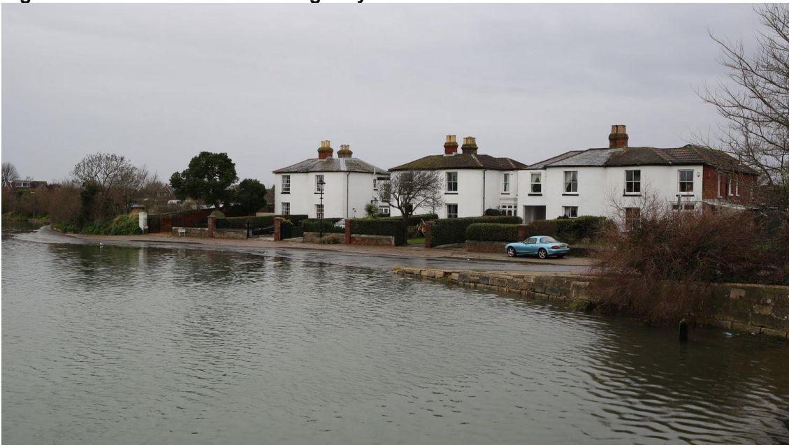
Figure 4.13: Numbers 1-6 Little Anglesey Road. Source: Mott MacDonald 2020.
