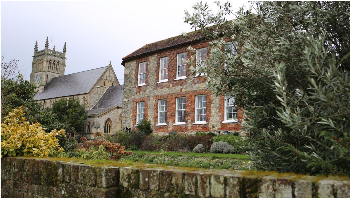
Figure 4.11: The Old Rectory Undercroft, Southern side. Source: Mott MacDonald 2020.
