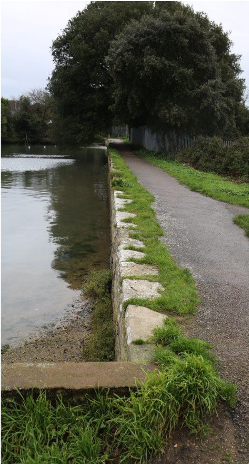
Figure 4.5: Scheme area looking South. Source: Mott MacDonald 2020
