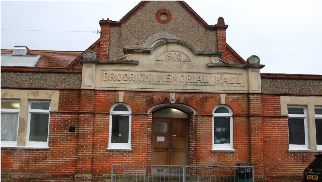
Figure 4.10: Brodrick Memorial Hall, Clayhall Road, South face. Source: Mott MacDonald 2020
