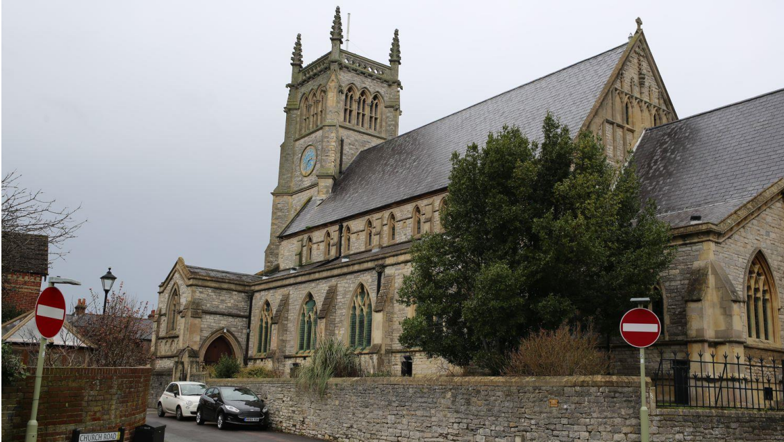
Figure 4.14: Southern side of the Church of St. Mary. Source: Mott MacDonald 2020.
