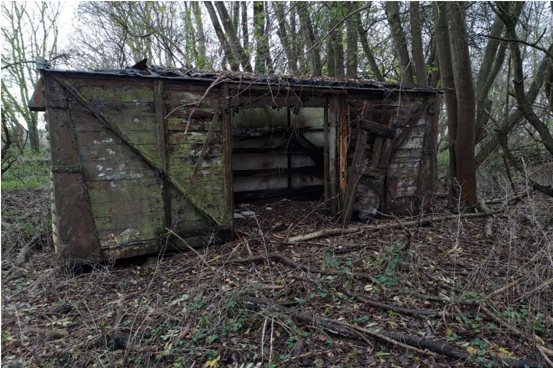
Photo 4.4: Abandoned Second War World train wagon, looking west
