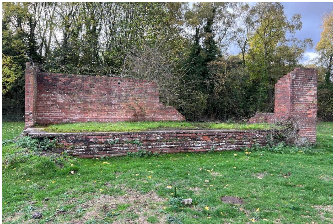
Photo 4.5: Single storey administration building, looking south-west
