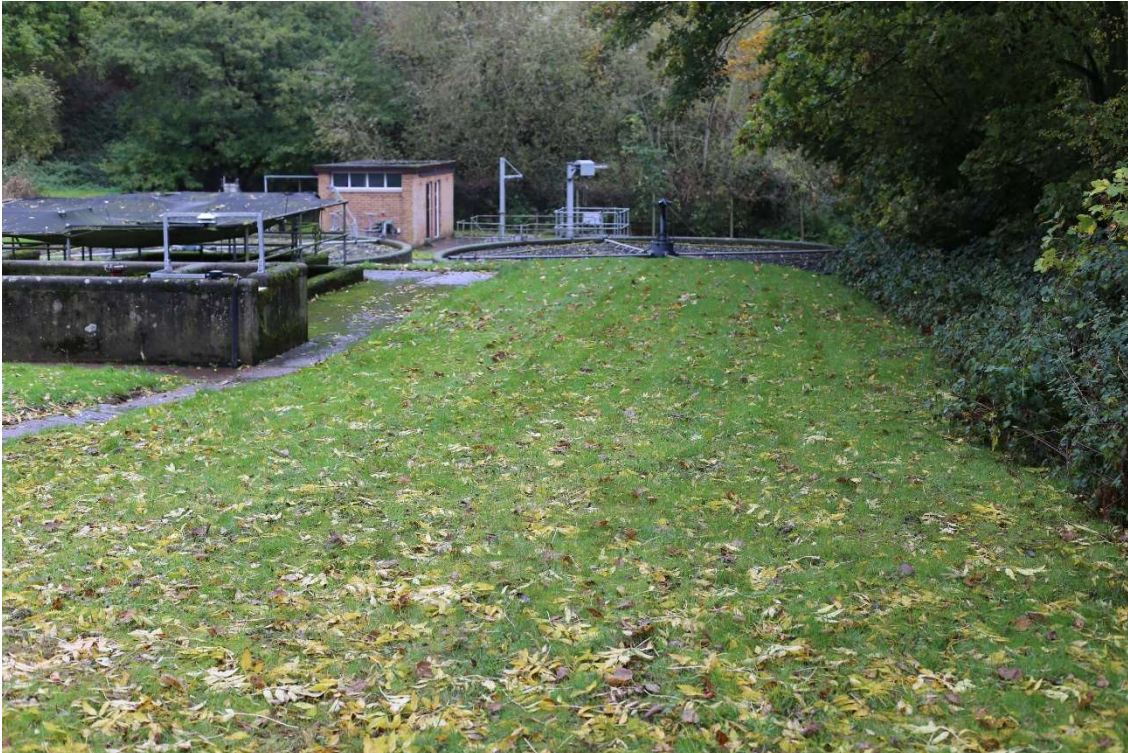
Photo 4.1: View of Ticknall STW, looking north
