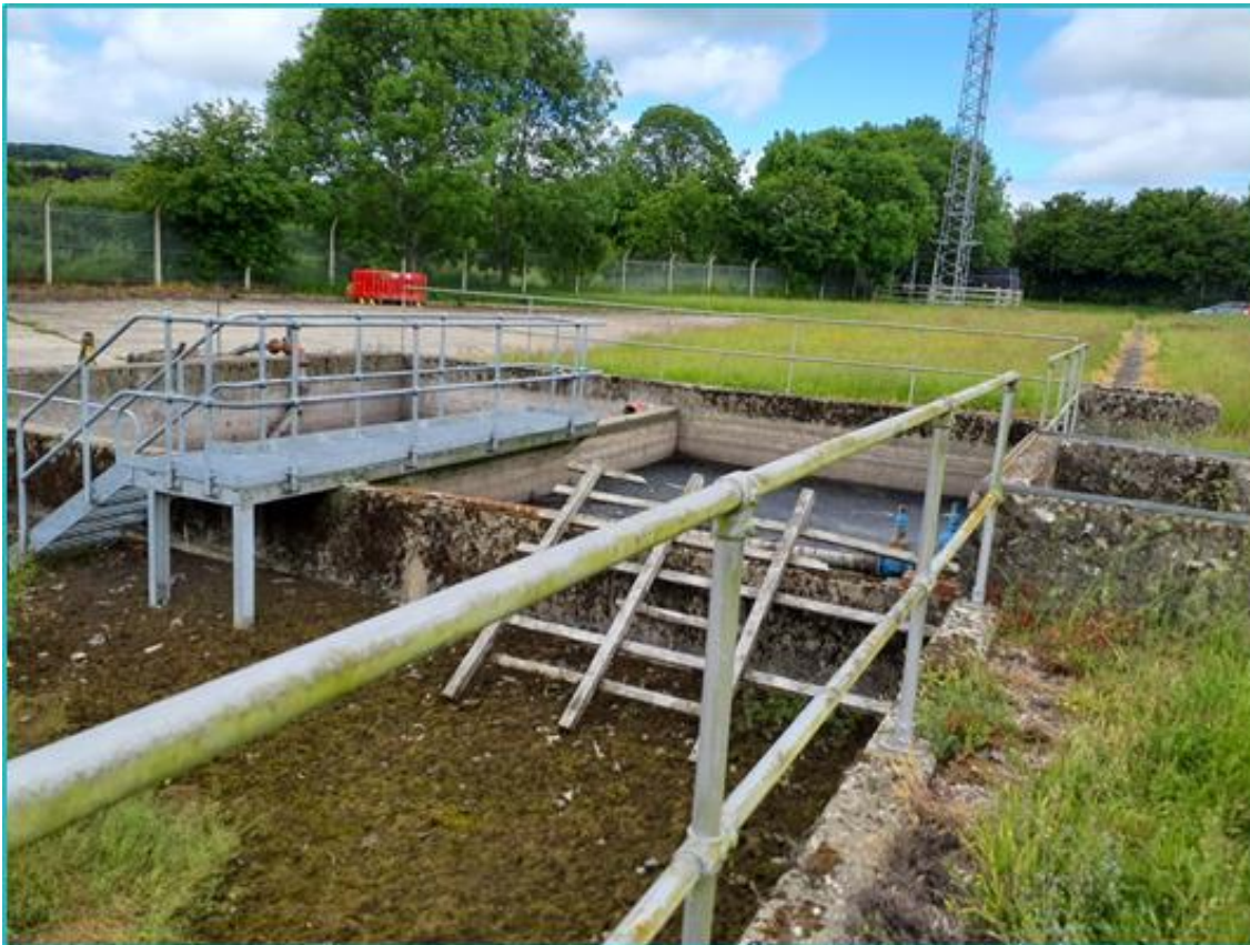
Figure 4.5: Ground disturbance caused by existing STW infrastructure
