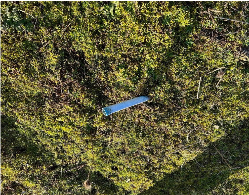
Photo 4.4: Building rubble and piping protruding from mossy ground to the east
