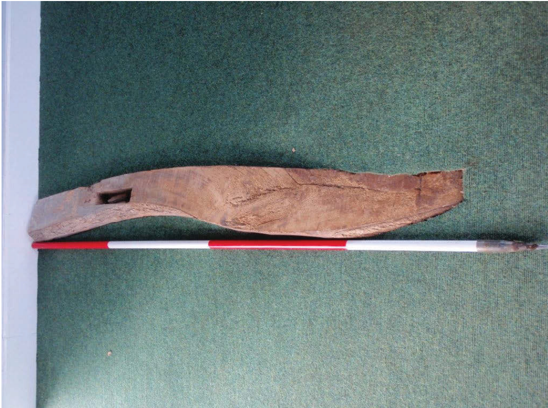
Plate 21: Exposed timber joist showing strut slot in floor of Upper Room
