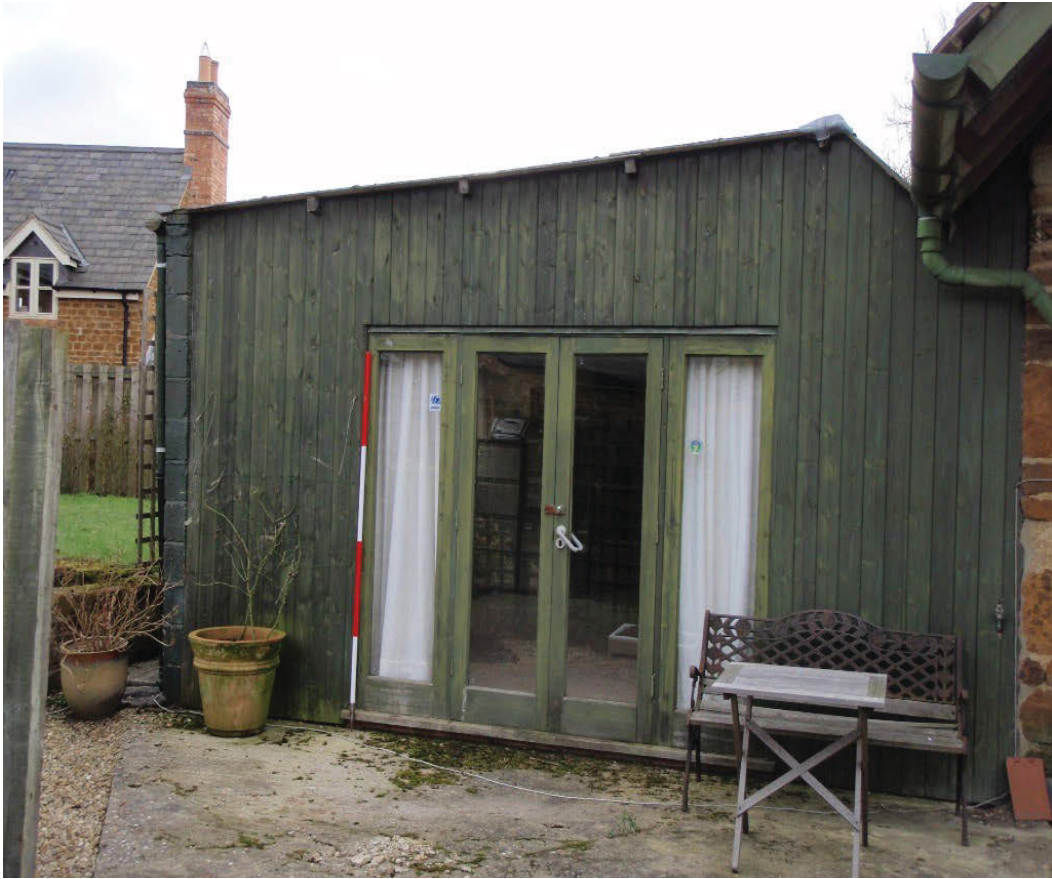
Plate 3: NW elevation, modern extension
