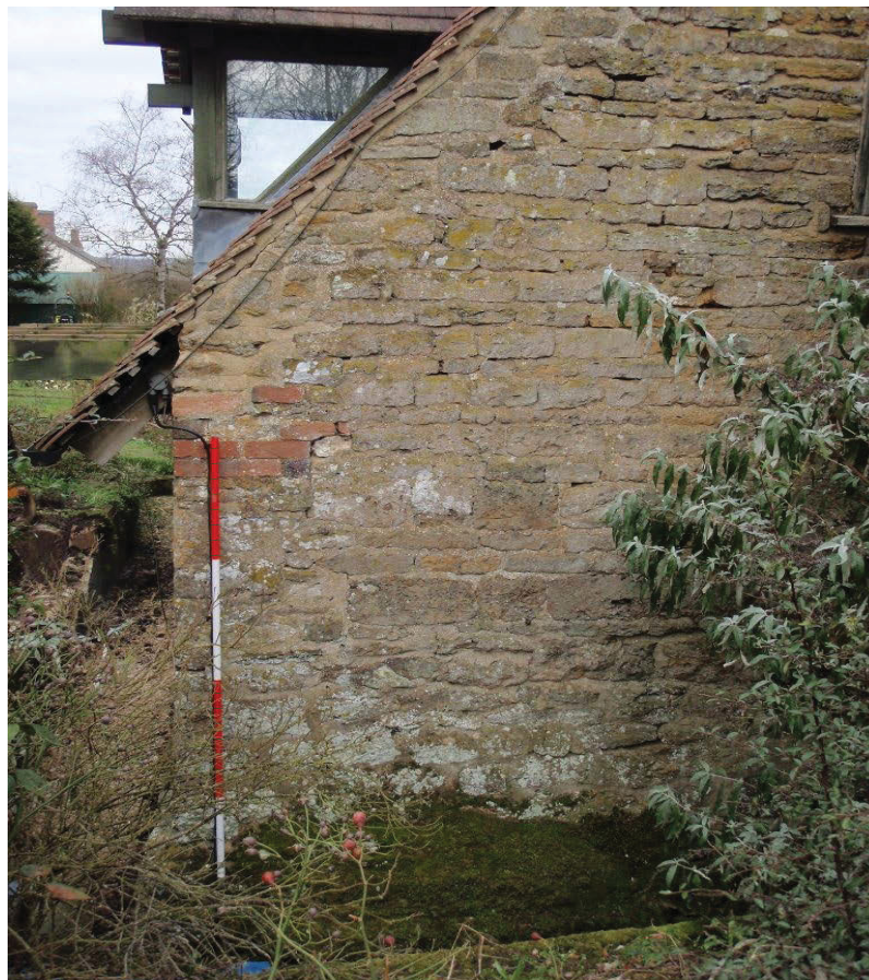
Plate 8: SE elevation showing brick repair
