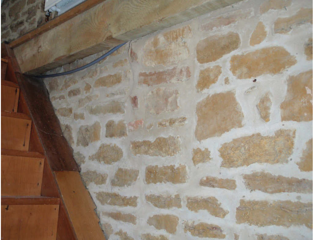
Plate 19: Possible blocked opening in SE gable wall
