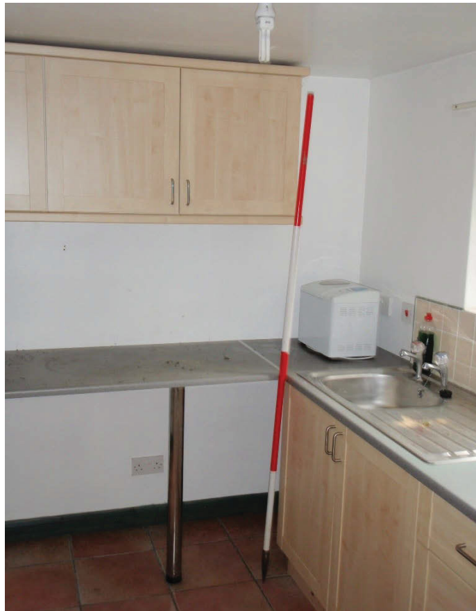
Plate 16: Kitchenette facing NE
