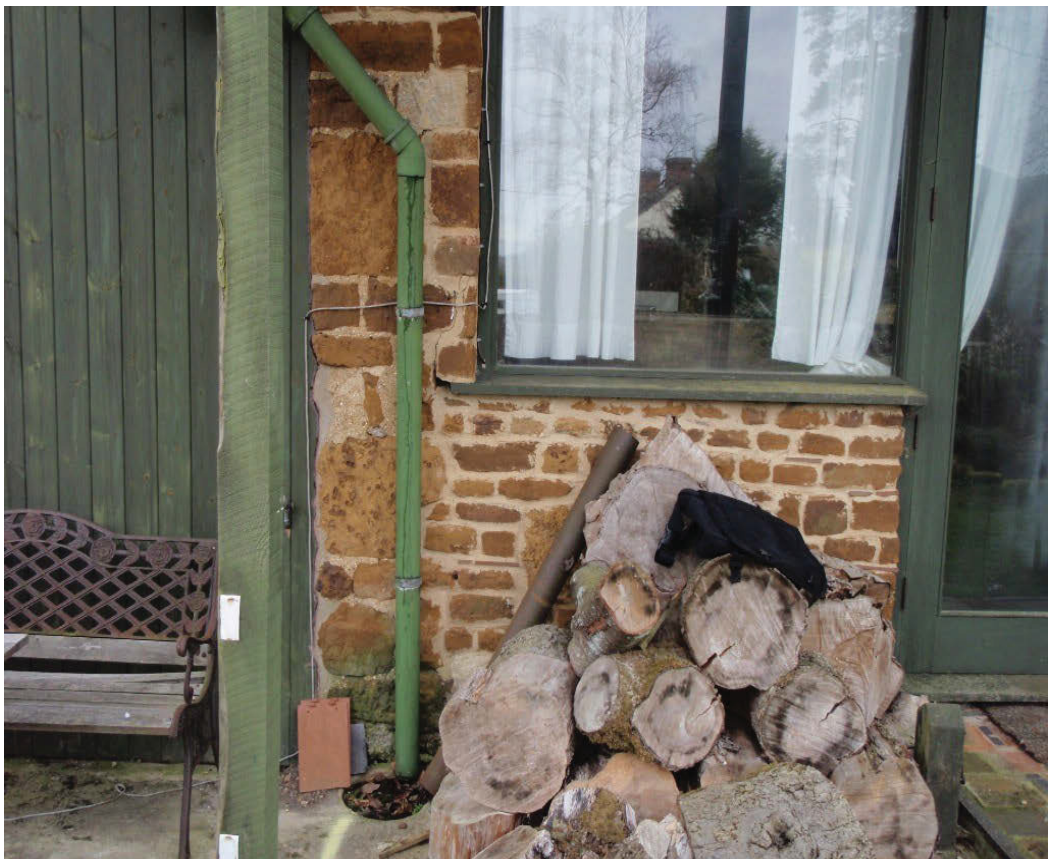
Plate 2: Detail of stonework in NW elevation
