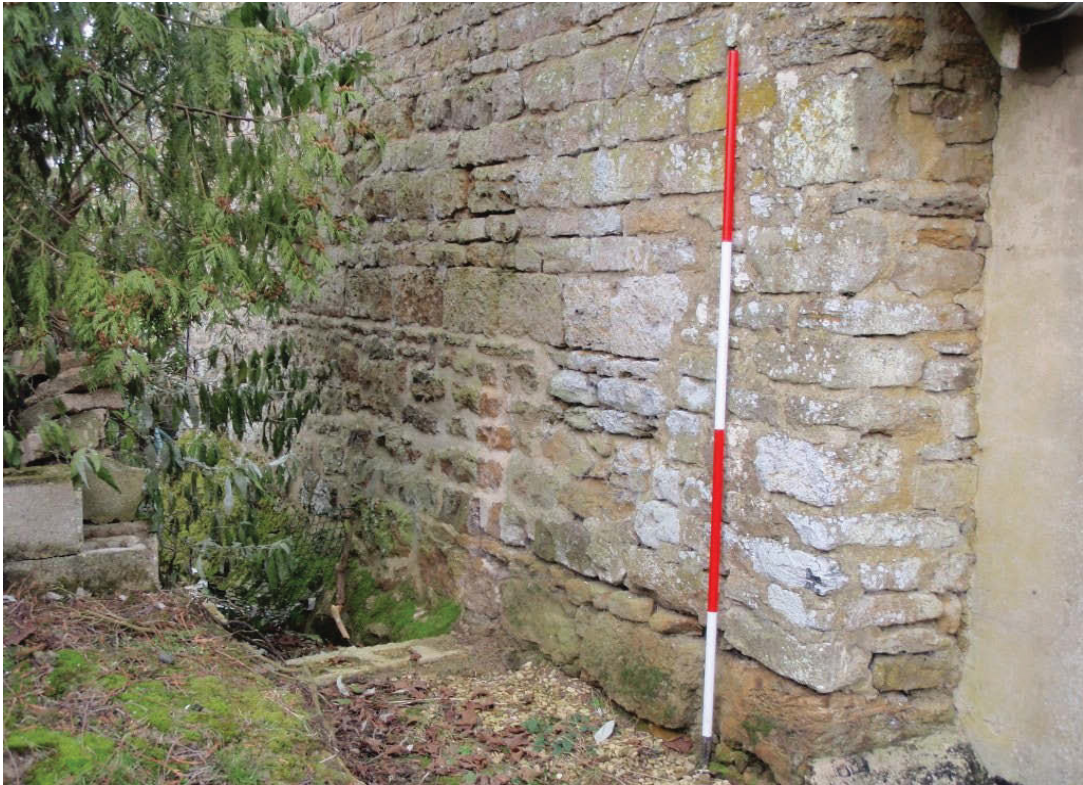
Plate 7: SE elevation showing repointing and part demolished block wall
