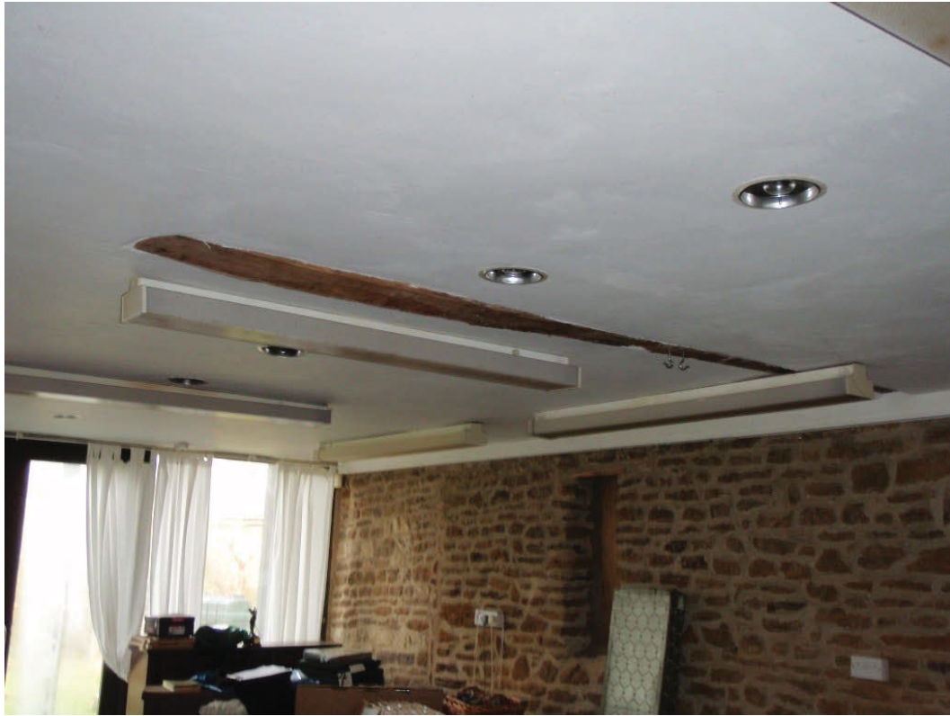
Plate 15: Games room, showing exposed timber joist in ceiling
