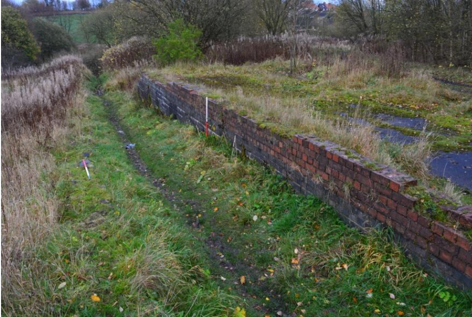
Figure 4.9. Brick foundations of Engine Shed (RSK 35) shown on 1898 OS map, Area C. Looking south east. 1m scales
