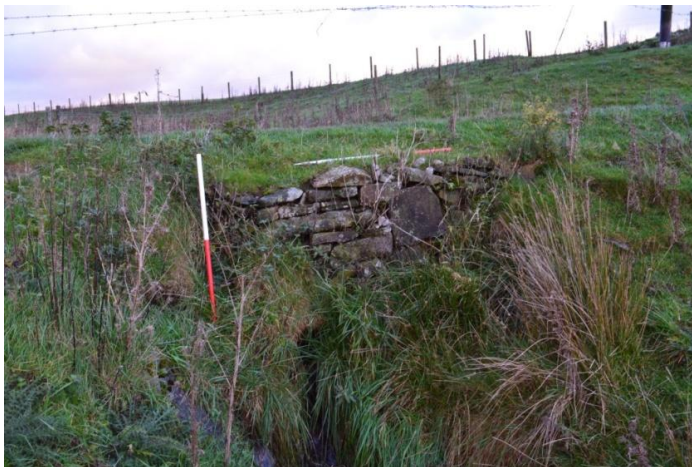
Figure 4.6. Dry stone revetment of tributary (RSK 37) in Area D. 1m scales
