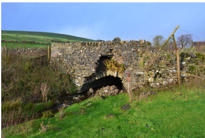
Figure 4.7. Bridge (RSK 36) in Area D over the Nun Brook. 1m scale
