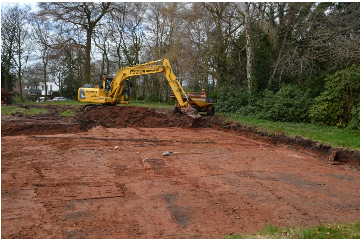
Figure 4. General view of Trench A, during excavation.
