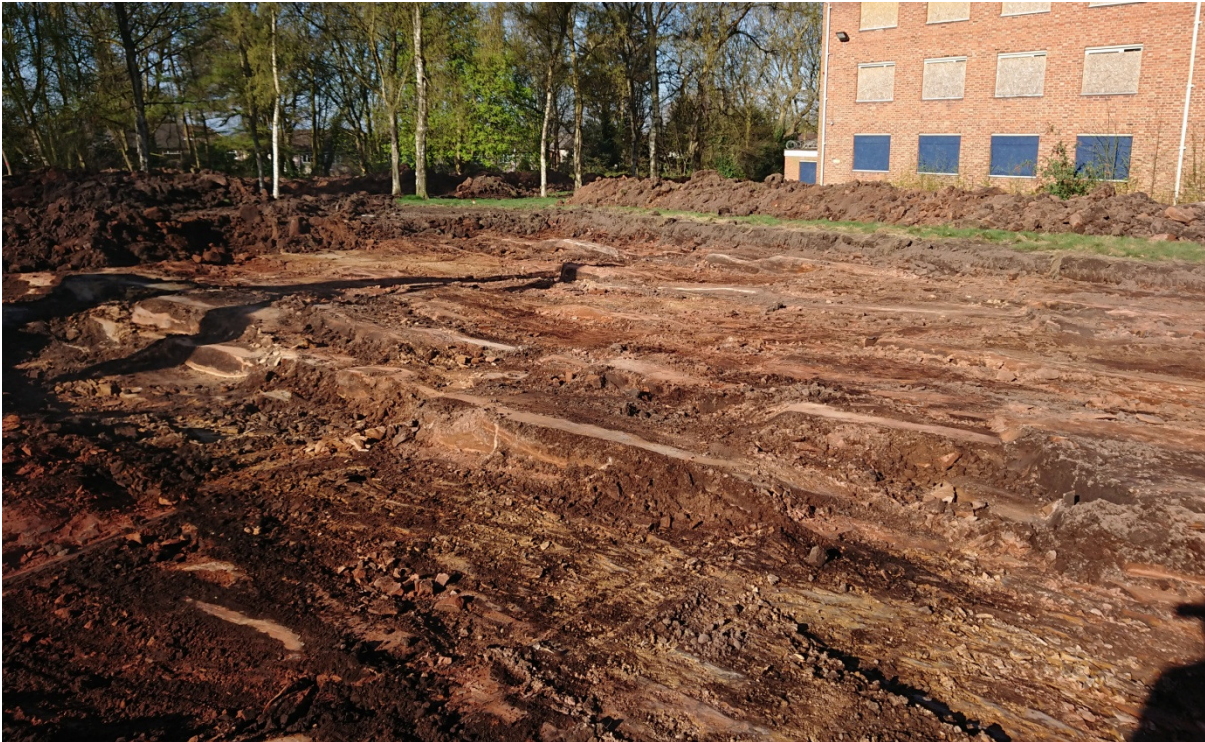
Figure 17. Trench B looking west.
