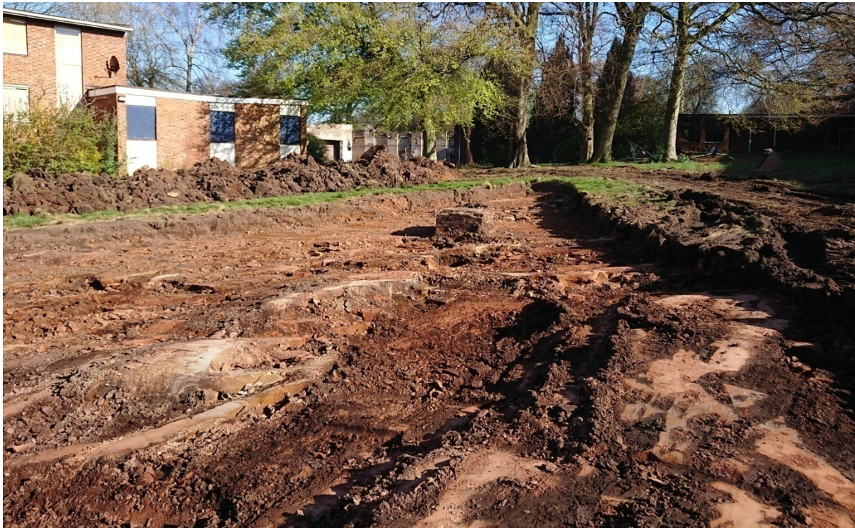
Figure 16. Trench B, looking north.
