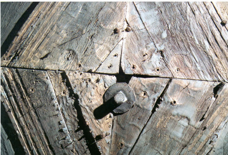
Raking light details showing some of the original painted decoration now showing as relief within the weathered timber surface.
