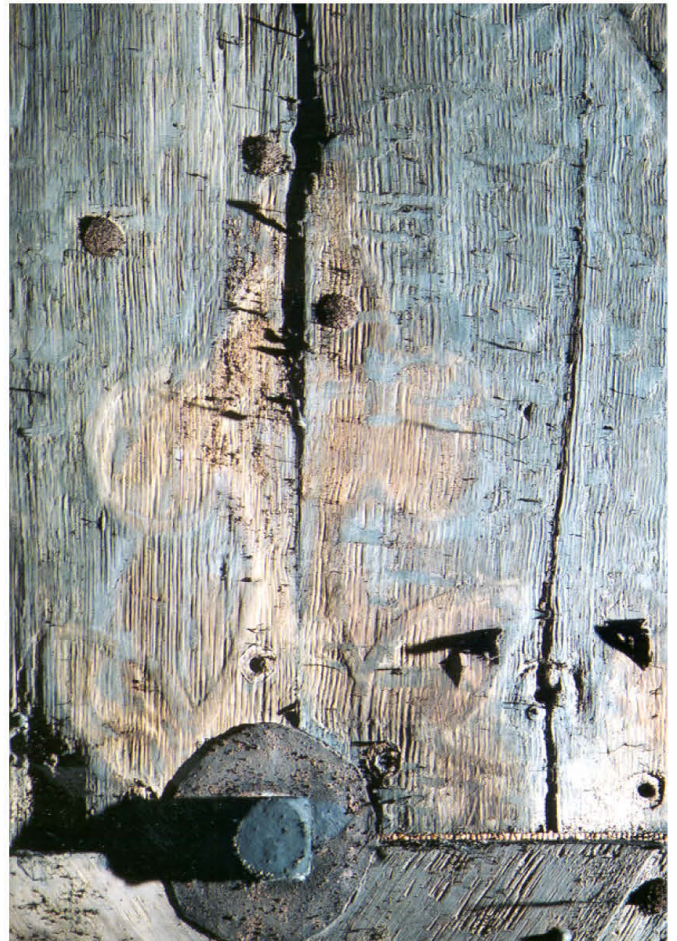
Plate 7. Detail of glue drips on the edge of 1890s boards. Removal tests indicate the glue may be removed by swabbing with warm water. On drying the underlying wood appears slightly lighter than if it were cleaned with wishabs only.
