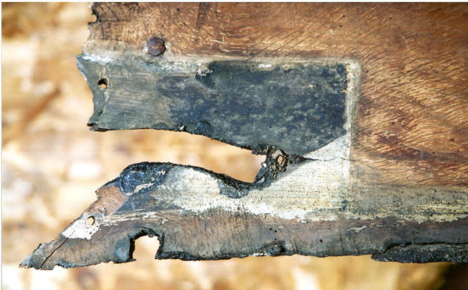
A typical lozenge showing the machined 1890s oak boards, some partially smeared with residue resulting from the stripping of painted decoration from the early thirteenth century original boards and the seventeenth century 'intermediate' boards.
