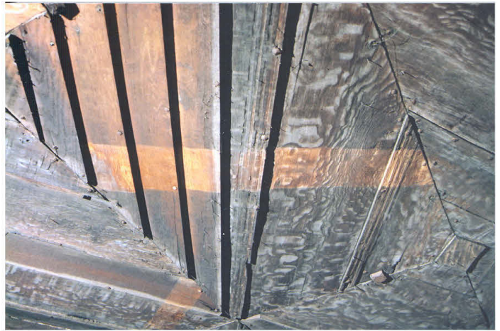
Plate 2. A surface cleaning test using wishab sponges to remove the thick accretions of soot and surface dirt across original and 1890s ceiling boards.
