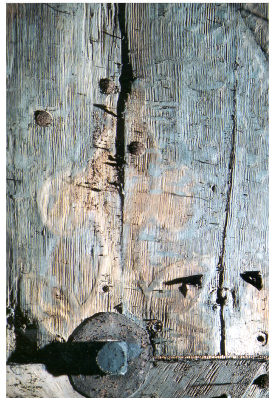
Raking light details showing some of the original painted decoration now showing as relief within the weathered timber surface.
