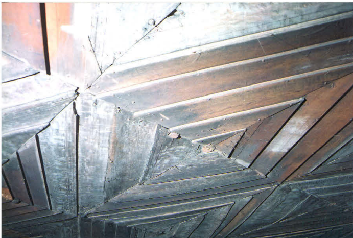
Plate 1. A typical lozenge showing the smooth-faced 1890s oak boards that are partially smeared with a darkened coating and/or some form of white ground where they are adjacent to early boards.
