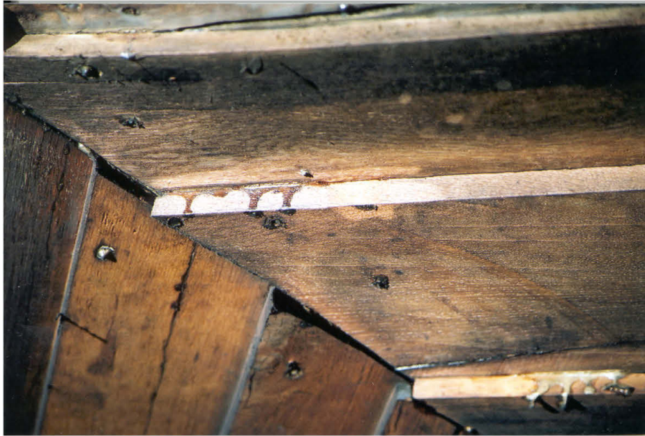
Plate 7. Detail of glue drips on the edge of 1890s boards. Removal tests indicate the glue may be removed by swabbing with warm water. On drying the underlying wood appears slightly lighter than if it were cleaned with wishabs only.
