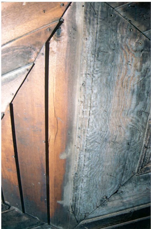
Plate 1. A typical lozenge showing the smooth-faced 1890s oak boards that are partially smeared with a darkened coating and/or some form of white ground where they are adjacent to early boards.
