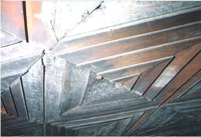
A typical lozenge showing the machined 1890s oak boards, some partially smeared with residue resulting from the stripping of painted decoration from the early thirteenth century original boards and the seventeenth century 'intermediate' boards.
