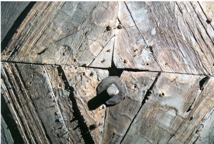
Plates 8 & 9. Raking light details showing some of the original painted decoration now showing as relief within the weathered timber surface.
