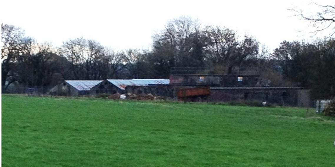
Figure 13. The Former Operations Block before renovation. Looking south-east
