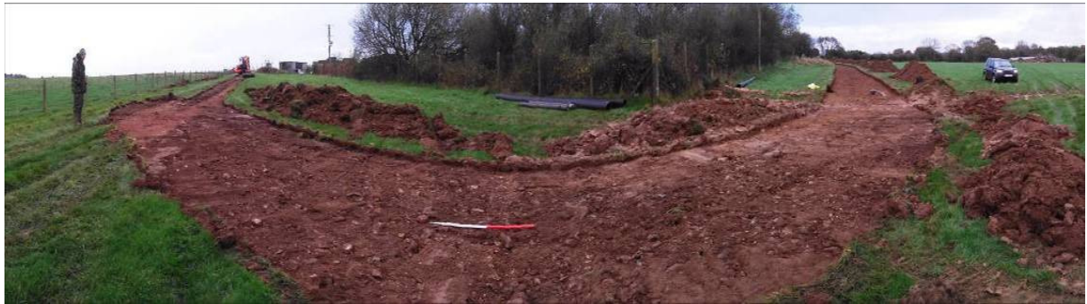
Figure 26. Panorama photograph of the corner between the western and northern arms of the watching brief trench. Surface of the old track exposed (left), Modern-disturbed subsoil102 (right) Looking NW from 331470 / 107230
