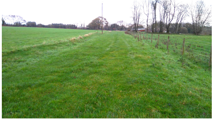
Figure 25. Remnants of the 'old track' as an earthwork. The Former Operations Block is in the background. Possible round-side drainage gully, and removed field boundary (left). Looking NE from 331550 / 107200
