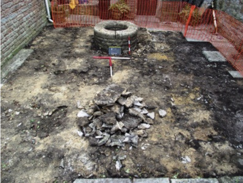
Figure 11 - Lias slabs (201) removed. Mixed surface of (202) & (203) exposed. A pile of cement associated with (201) is in the foreground. The trench from 1992 is visible on the right side of the photograph. Looking south.
