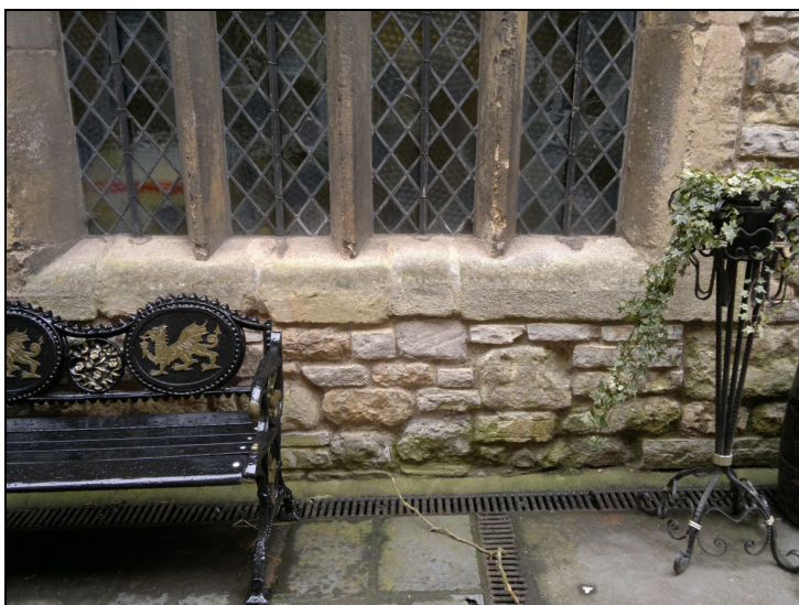
Figure 39. A blocked doorway can be seen below the east-facing window in Room 5.
