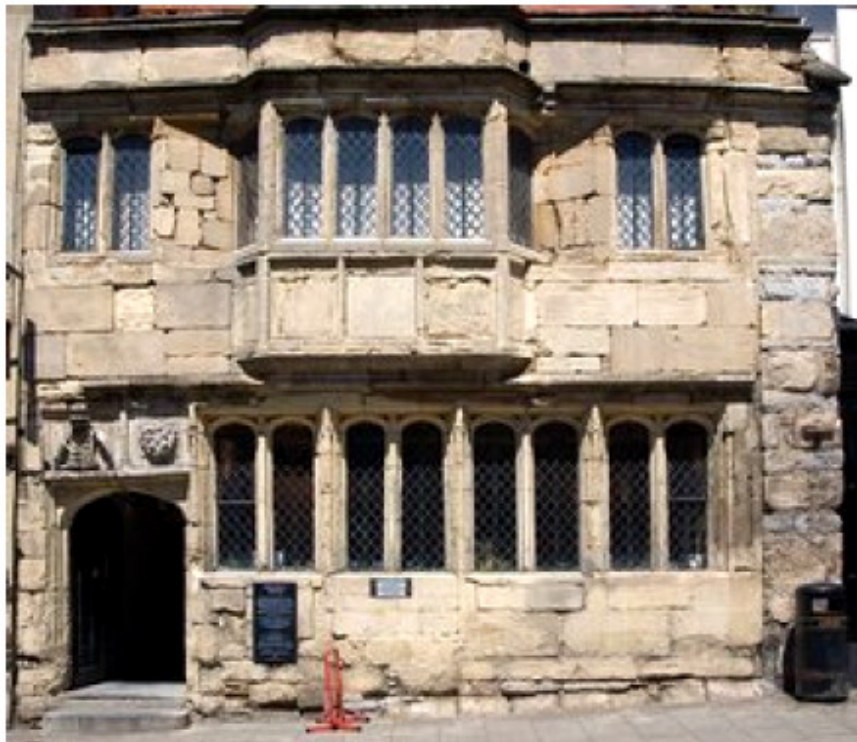
Figure 3. The street frontage of the building known as the Tribunal 6 ; note the earlier masonry of the east gable wall to the right of the photograph. The facade of the building displays several additions and alterations carried out during the medieval period.
