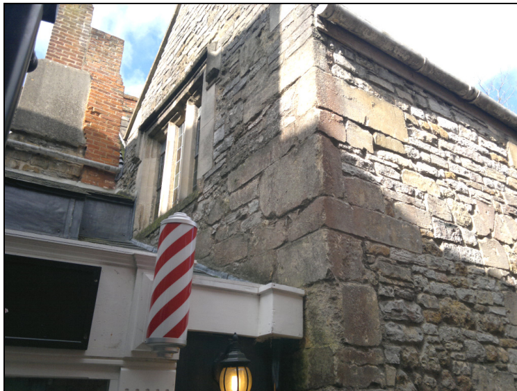
Figure 5. Photograph of Room 5 from the rear of 11 High Street.
