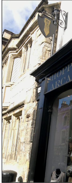
Figure 4. Detail of the join between the Tribunal and number 11 High Street.
