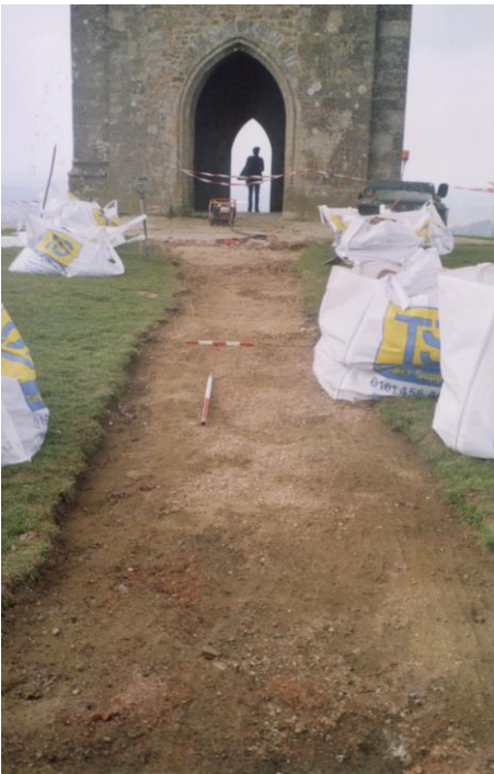
path east of tower: finished ground reduction
