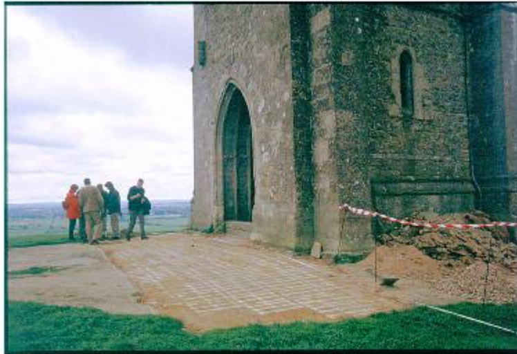
Figure 4. Photograph of exposed 1983 works.
