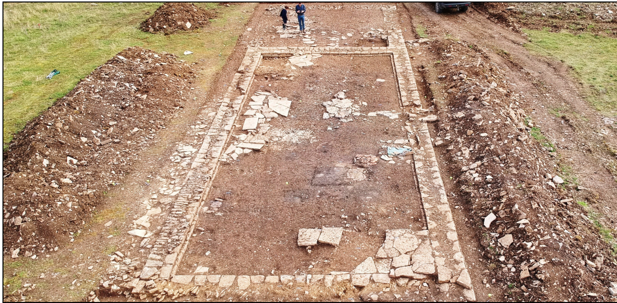
Figure 108. Drone photograph of RB Structure 1. Main building component F24101 is in the foreground, and extension F24102 is in the background. The partially subsided and collapsed western wall is visible, along with the buckled western end of the northern wall where the surface of the foundations have been exposed and the faced stone is absent. Looking ESE.
