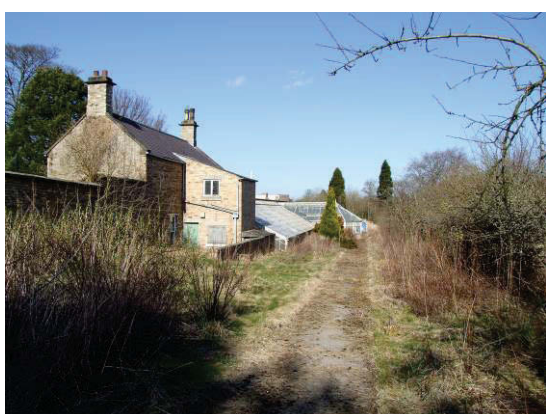
Figure 8 The walled garden was probably built c.1870, to supply the house with produce. The glasshouses were altered c.1904 by the important firm, Richardson of Darlington.
