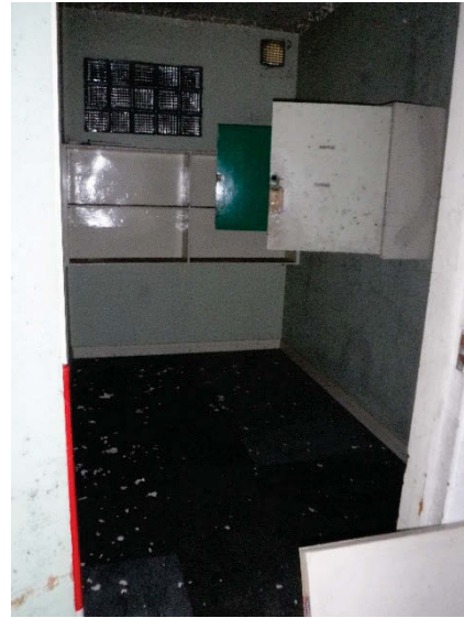
Plate 221 Building 45, Cavell, interior converted secure bedroom. Facing south-east. [2674]
