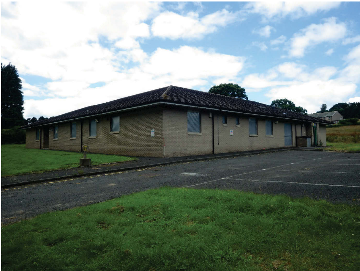
Plate 23 Building 7: Stephenson House Special Care Unit. General setting view. Facing north-west.
