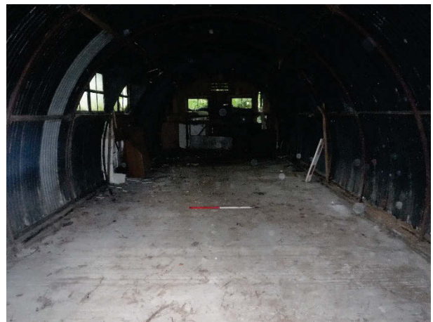
Plate 247 Building 62, interior general view. Facing north-east. [2837]
