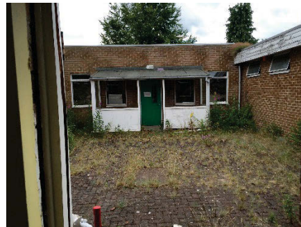
Plate 39 Building 12 Fraser House internal courtyard
