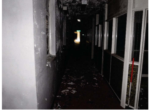
Plate 272 Building 69, Darwin & Seguin, first floor internal corridor, south end. Facing north-east. [2612]
