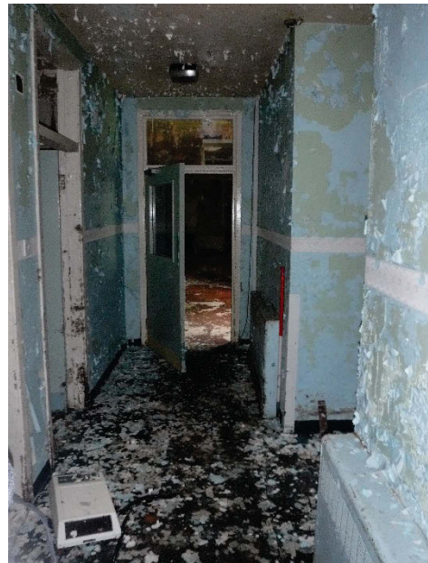
Plate 253 Building 67, Greengates interior corridor, central wing. Facing south. [2737]
