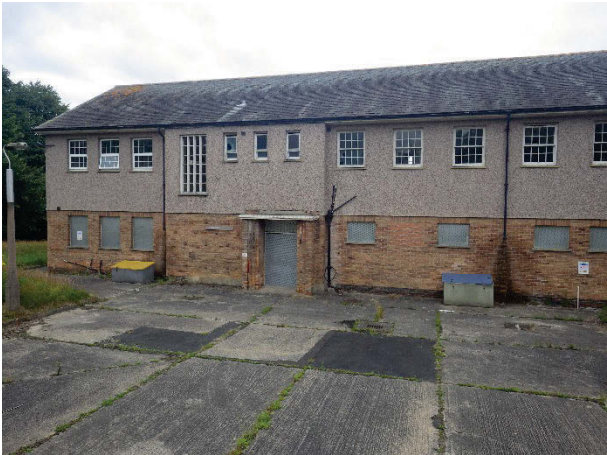
Plate 57 Building 17 Brinkburn west elevation, north side [1668]
