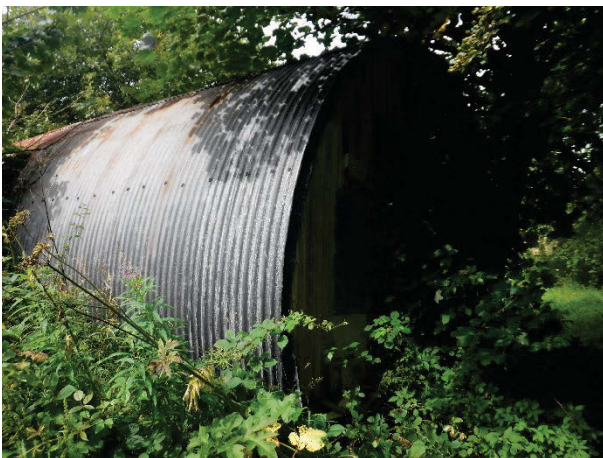
Plate 246 Building 62, exterior general view. Facing north-west. [2852]
