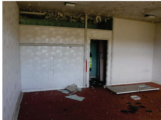
Plate 223 Building 45, Cavell, interior first floor dormitory, ?altered partitions. Facing north. [2688]
