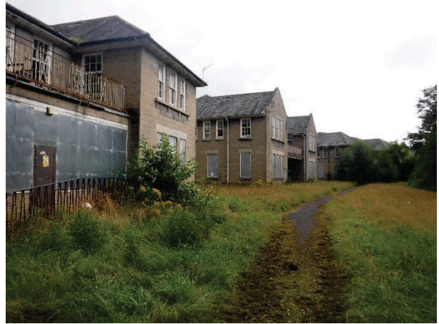
Plate 227 Buildings 49 (foreground) – 47 (background), general setting view. Facing north-east. [2826]
