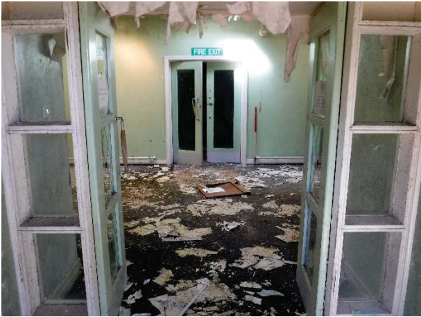
Plate 182 Building 38, main entrance hall. Facing west. [1012]
