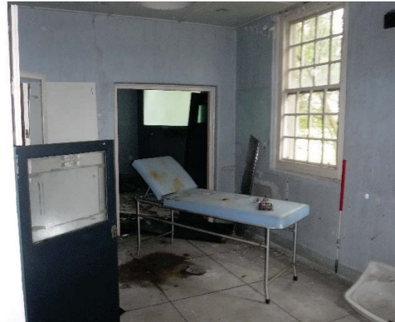
Plate 113 Building 29, Redburn interior. Ground floor anaesthetist room. Facing west. [2372]
