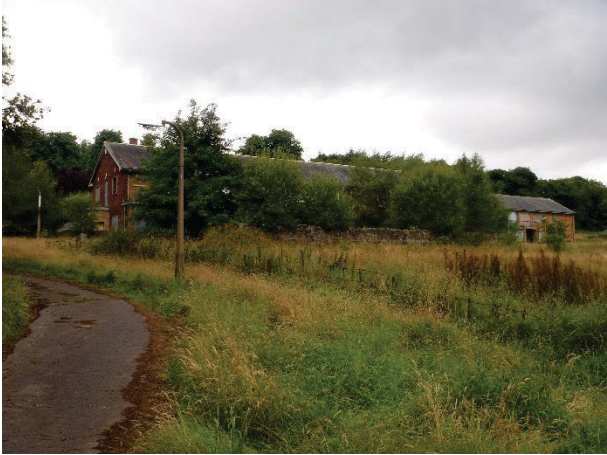
Plate 186 Building 39, Nurses Accommodation general setting view. Facing north. [2783]
