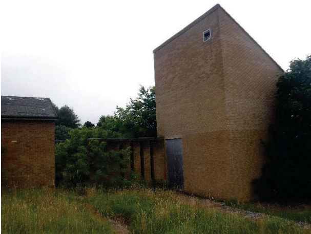
Plate 192 Building 41 exterior. Facing east. [2219]
