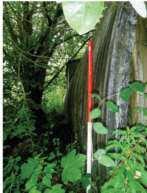
Plate 245 Building 62, exterior general view. Facing east. [2835]
