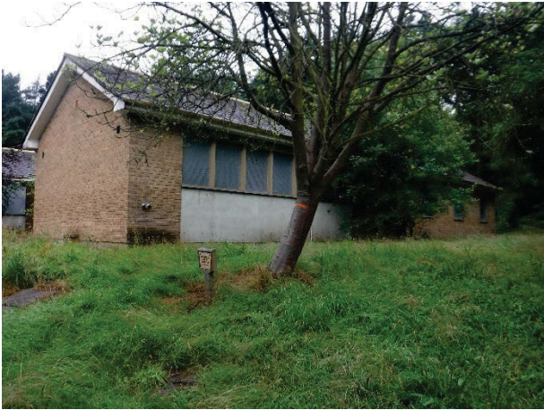
Plate 250 Building 67 Greengates exterior north-east elevation. Facing west. [2720]
