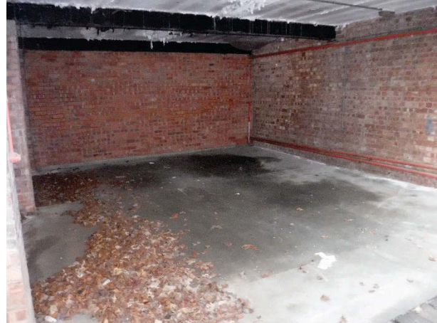
Plate 241 Building 54 interior. Facing south-east. [2352]
