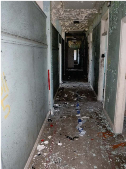
Plate 222 Building 45, Cavell, interior first floor internal corridor. Facing south-west. [2685]
