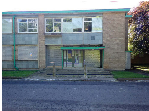
Plate 125 Building 31, McCoull Clinic exterior, north west (front) elevation detail of entrance mosaic.
