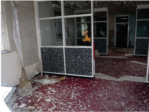
Plate 258 Building 67, Greengates interior cross-range dormitory. Facing north-east. [2767]
