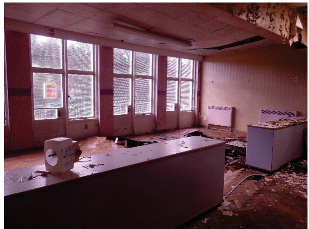
Plate 131 Building 31, McCoull Clinic interior, waiting room. Facing south. [1827]
