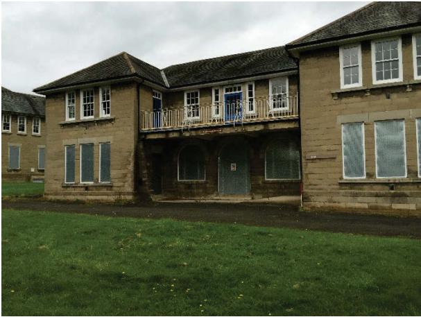
Plate 87 Building 24, Tyne Villa exterior, south (front) elevation. Facing north. [3078]
