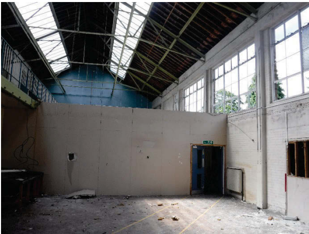
Plate 164 Building 35, Central Stores, interior, partitioned main hall. Facing south-west. [1940]
