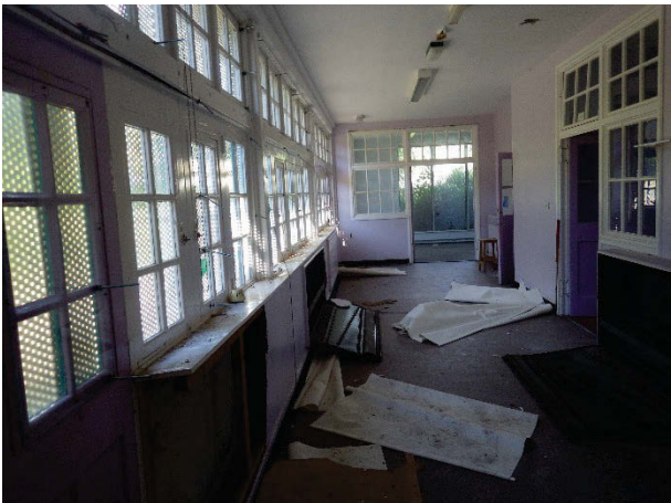
Plate 122 Building 30, The Close, interior corridor. Facing west. [1764]
