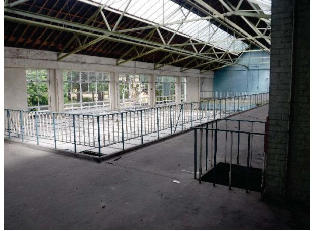
Plate 169 Building 35, Central Stores, interior, first floor walkway. Facing north-east. [1968]
