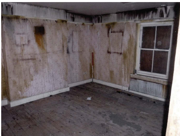
Plate 7 Building 56, Gardener's Cottage interior first floor bedroom 1. Facing west. [2282]
