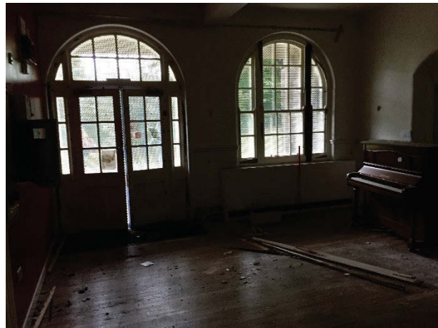
Plate 90 Building 24, Tyne Villa interior, main hall/dayroom. Facing south. [3103]
