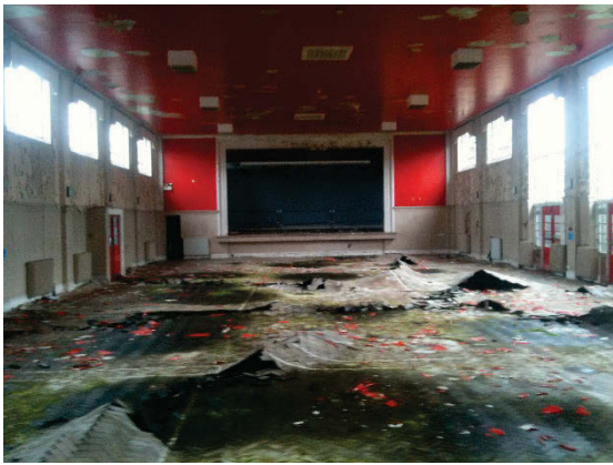
Plate 146 Building 32, Recreation Hall interior main hall. Facing south-west [3237]
