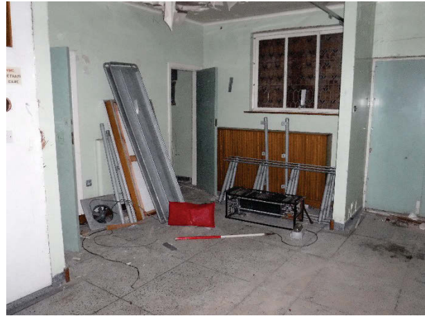
Plate 97 Building 27, Mortuary interior. Facing south-west. [1009]
