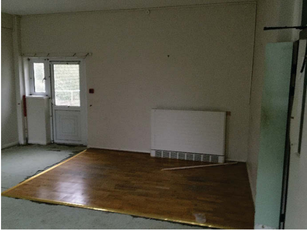
Plate 104 Building 28, Riding interior. "Lounge". Facing south. [3208]
