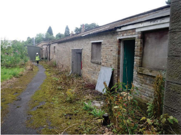
Plate 13 Building 58-60, Potting sheds exterior general view. Facing east. [2298]
