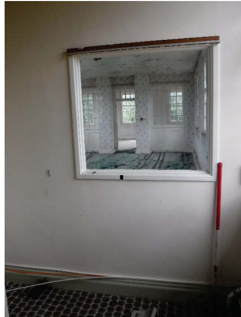
Plate 179 Building 37, Holly/Cedar interior, first floor view from nurses station. Facing south-west. [2035]
