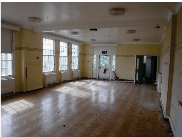
Plate 63 Building 17 Brinkburn ground floor day room; annexe wing stairs in background. Facing south. [1698]
