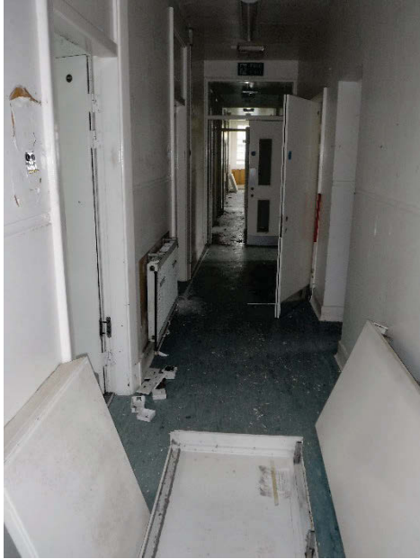
Plate 116 Building 29, Redburn interior. First floor internal corridor. Facing south-west. [2419]
