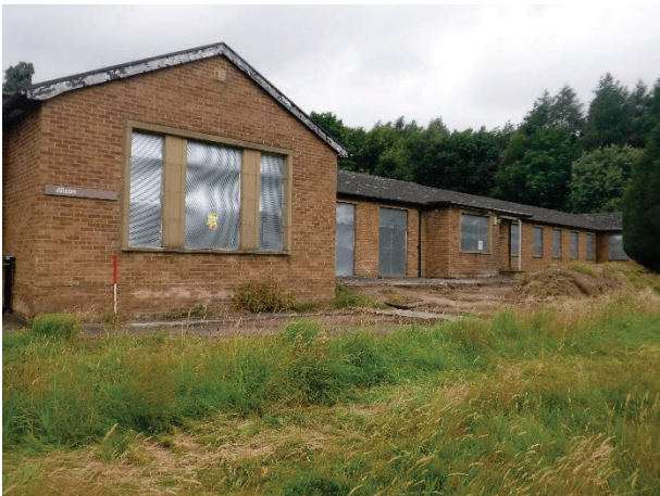
Plate 190 Building 40, Alison exterior south-east (front) elevation. Facing north. [2152]
