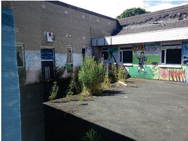
Plate 30 Building 7 Stephenson House Internal Courtyard. [1494]
