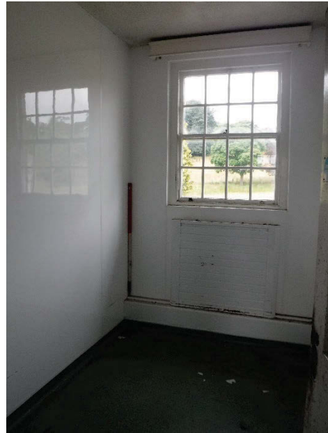
Plate 66 Building 17 Brinkburn first floor single dormitory room with wall surface treatment [1726]
