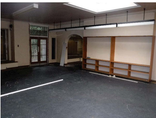
Plate 212 Building 44, Patients' Shopping Centre, general view room g25, 'shop male'. Facing south-east. [2141]
