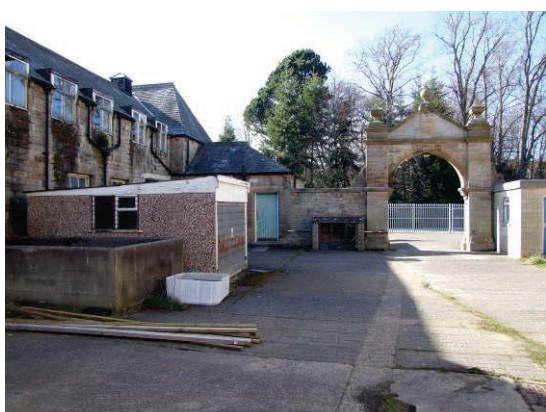
Figure 6 The service yard to the south west of the hall. The former stables buildings to the left were been heavily altered in the twentieth century.
