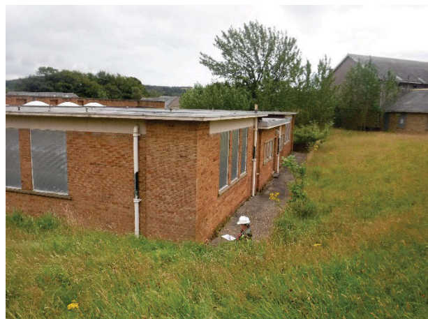
Plate 207 Building 44, Patients' Shopping Centre, external north elevation. Facing south-west. [2092]
