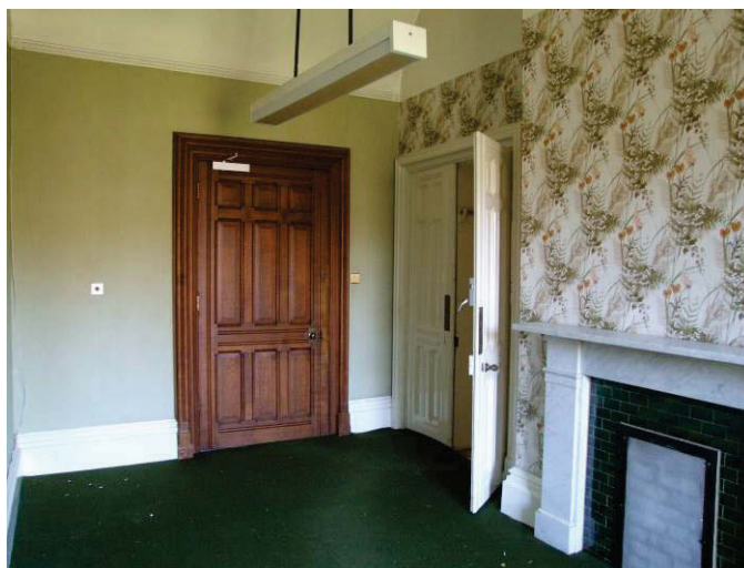
Figure 72 One of the heavily altered rooms in the first floor of the 1870s block.
