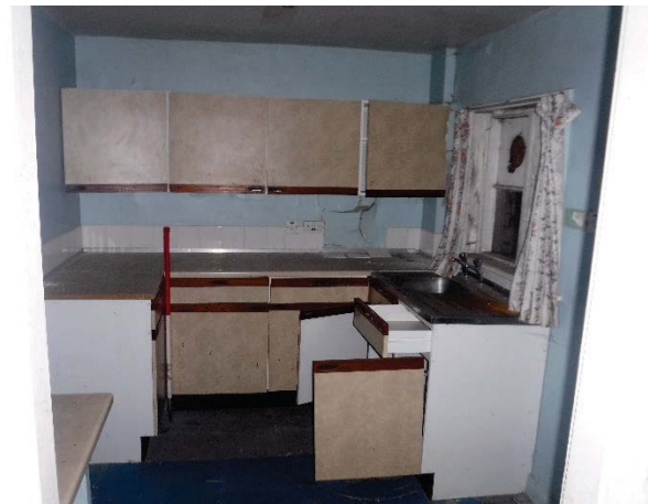
Plate 6 Building 56, Gardener's Cottage interior ground floor kitchen. Facing south-east. [2274]
