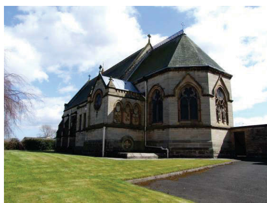
Figure 9 Our Lady & St Cuthbert's Church, Highfield Lane, Prudhoe. This is the chapel chevet which was built for the Liddell family c.1870. It was moved and extended with a nave c.1889, and finally moved to its present site in 1904, when the hall was sold.
