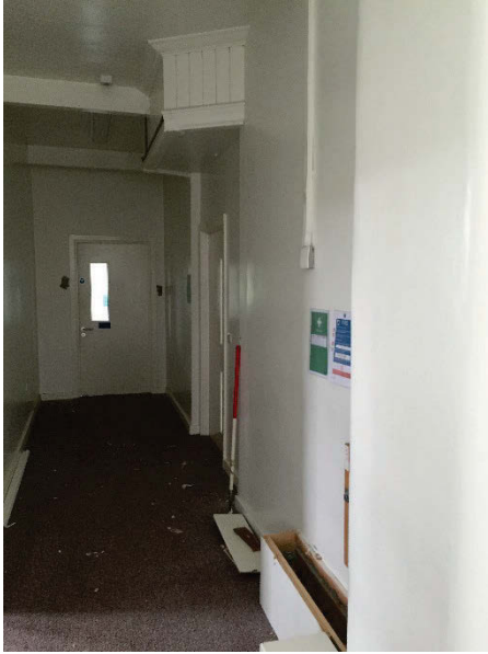
Plate 93 Building 24, Tyne Villa interior, first floor east wing partitioned dormitory. Facing south. [3130]
