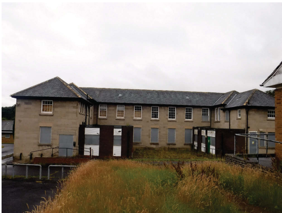
Plate 86 Building 23, Skerne Villa, external north-west elevation. Facing south-east. [1404]
