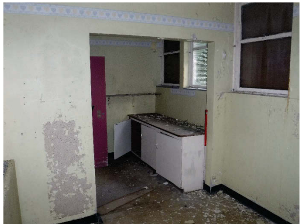
Plate 261 Building 67, Greengates interior subdivided bathroom and drying room. Facing north. [2776]
