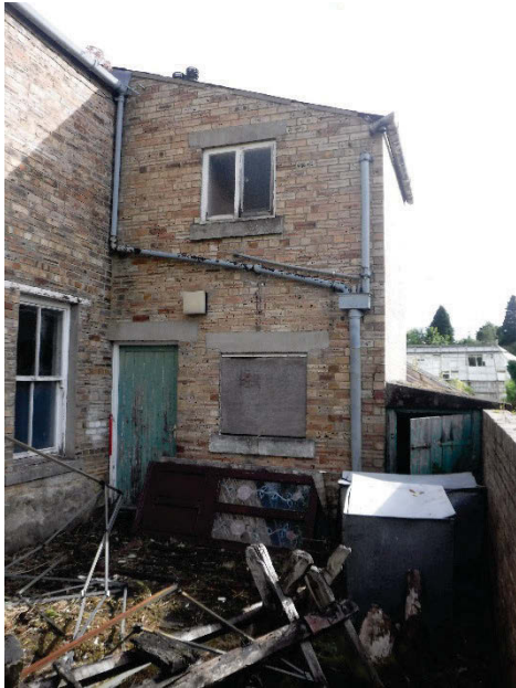
Plate 3 Building 56, Gardener's Cottage rear external elevation, kitchen and yard. Facing north-east. [2284]
