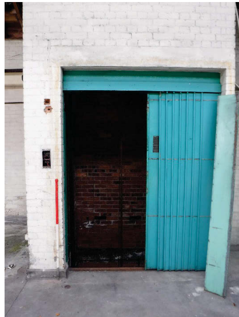
Plate 171 Building 35, Central Stores, interior, first floor walkway lift shaft. Facing south-east. [1969]
