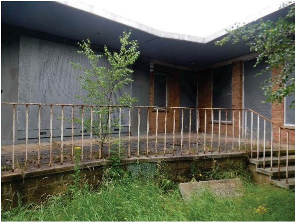
Plate 202 Building 44, Patients' Shopping Centre, external east (front) elevation. Facing north-west. [2101]
