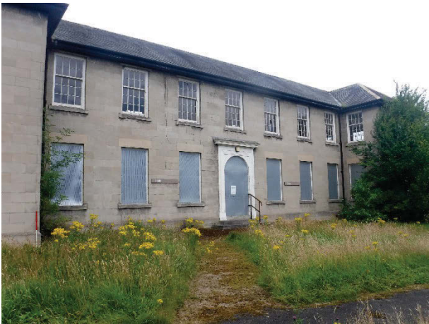
Plate 172 Building 37, Holly/Cedar exterior south-east (front) elevation. Facing north. [1987]
