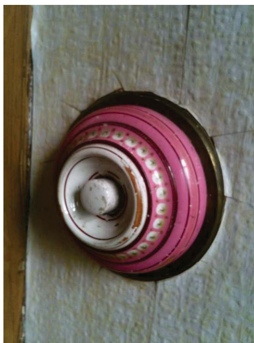
Figure 55 Electric bell-pushes. These may date from the 1889 installation of electricity in the hall.
