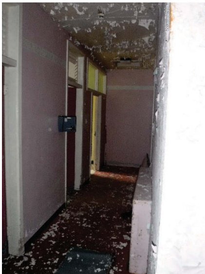
Plate 260 Building 67 interior corridor with new and blocked doors. Facing south-east. [2774]
