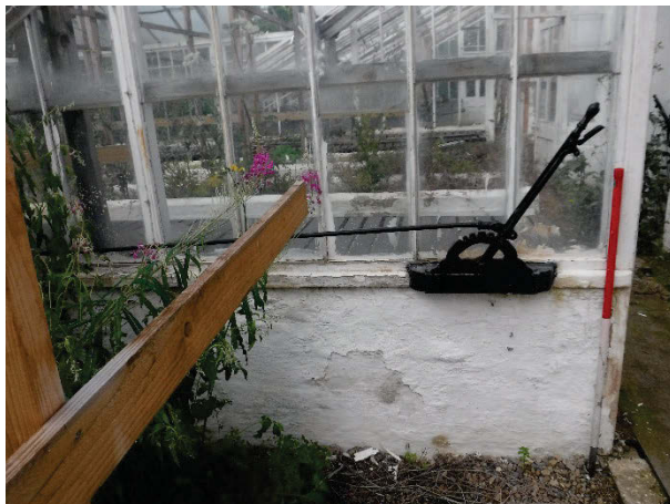
Plate 11 Building 58-60, Glasshouses detail of window lever marked 'Richardson Darlington'. Facing south-west. [2326]
