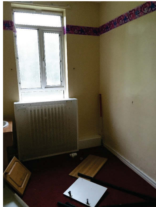
Plate 107 Building 28, Riding interior. Ward room, north-east wing. Facing north-west. [3222]
