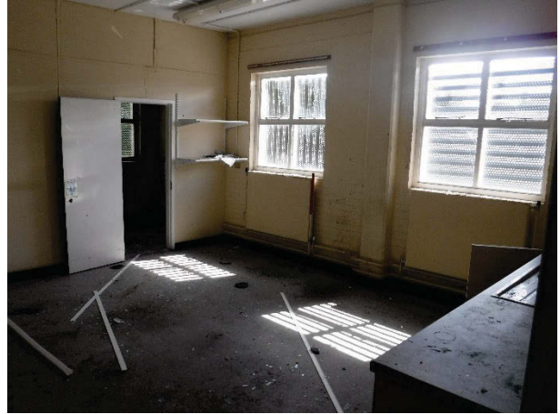
Plate 163 Building 35, Central Stores, interior, partitioned room g19. Facing east. [1935]
