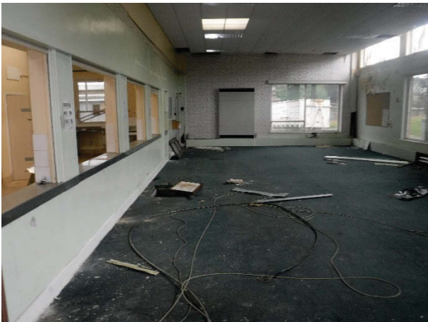
Plate 154 Building 34, Derwent Kitchens and Dining Hall interior, dining hall. Facing south-east. [2478]
