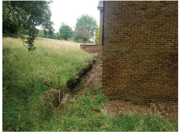
Plate 69 Building 18 Tredgold Hall, detail of sandstone terrace wall. Facing north. [3008]
