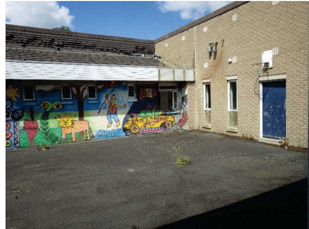
Plate 31 Building 7 Stephenson House Internal Corridor. Facing SW.Courtyard [1495]
