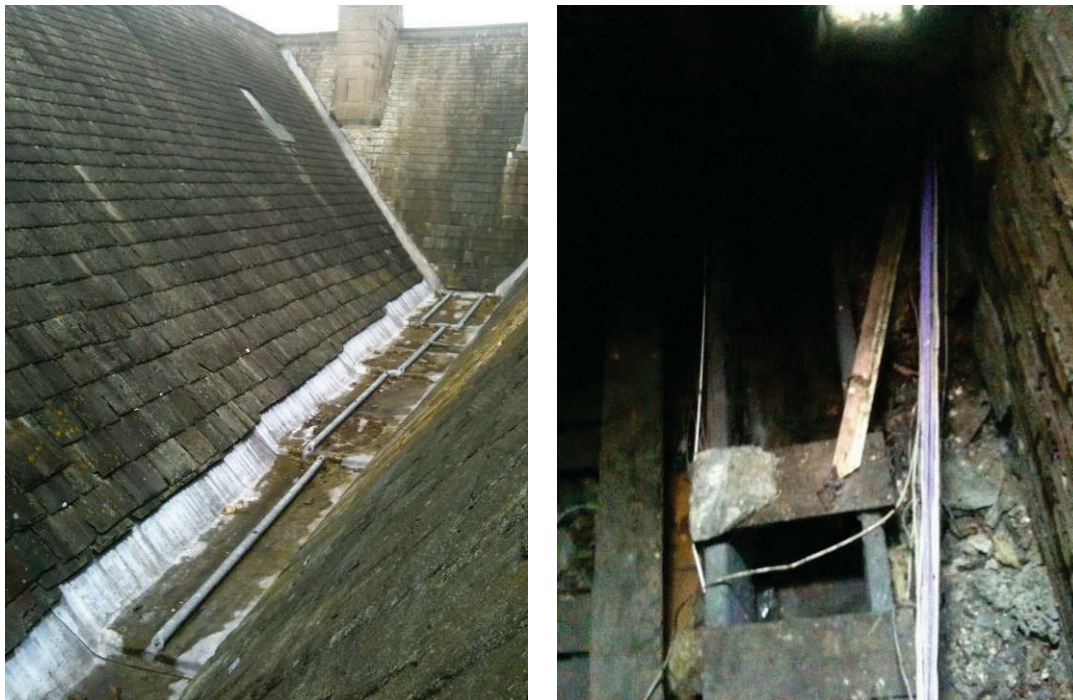
Figure 33 The lead-lined valley between the inward-facing pitches, over the 1870s core of the hall. It falls to the west, and water passes into the west pitched roof, through a lead-lined box channel, and into a rain-water hopper on the tower, at the centre of the south garden façade.
