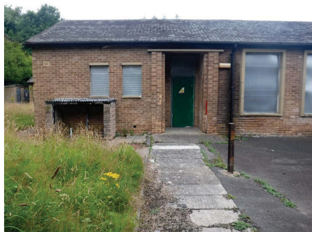
Plate 191 Building 40, Alison exterior south-west pavilion wing SW elevation. Facing NE. [2149]
