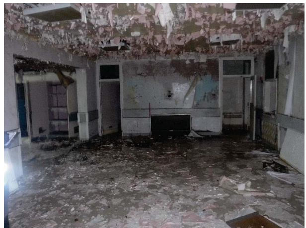
Plate 255 Building 67, Greengates interior day room. Facing south-west. [2744]
