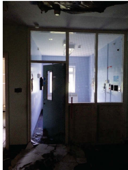
Plate 27 Building 7 Stephenson House Nurses' Station [1468]
