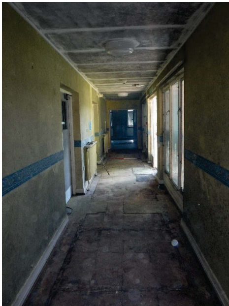
Plate 184 Building 38, main angles corridor, S end. Facing south-east. [1018]
