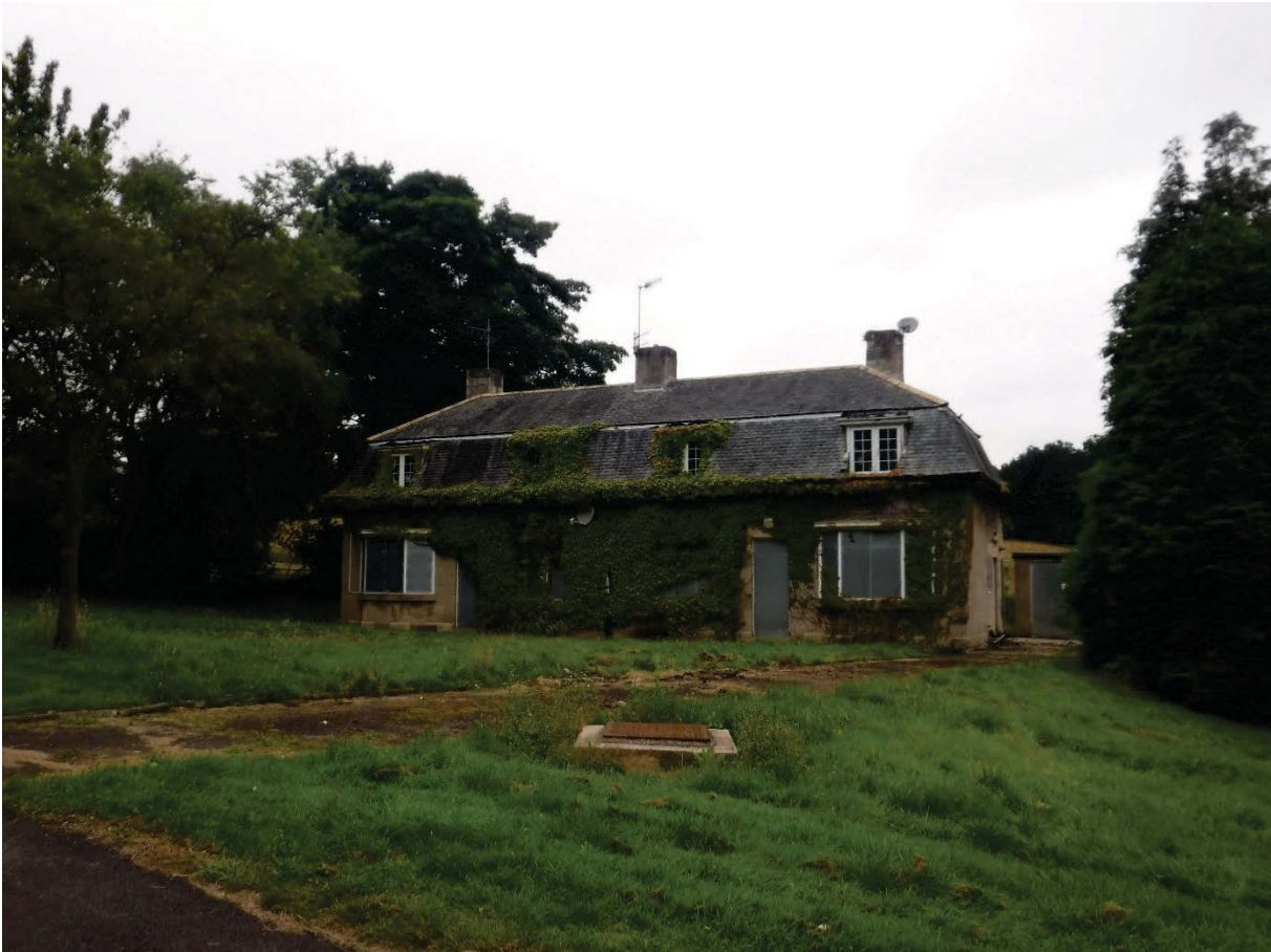
Plate 18 Building 5 General view [1383]
