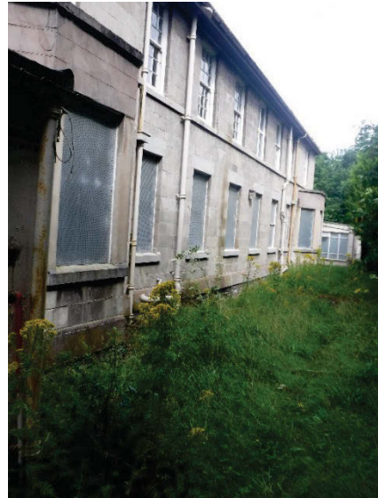
Plate 111 Building 29, Redburn exterior, south-east (rear) elevation. Facing north-east. [2451]
