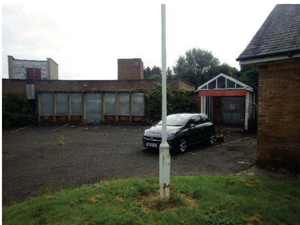
Plate 42 Building 13 Midway/Janie Hepple Unit exterior view: main entrance. Facing south-east [1555]
