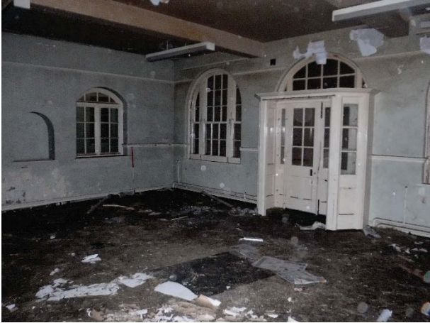
Plate 232 Building 47, Lime, interior day room with main external doors. Facing east. [2056]
