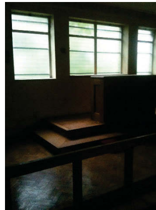
Plate 147 Building 32, Recreation Hall interior chapel. Facing south-west [3233]
