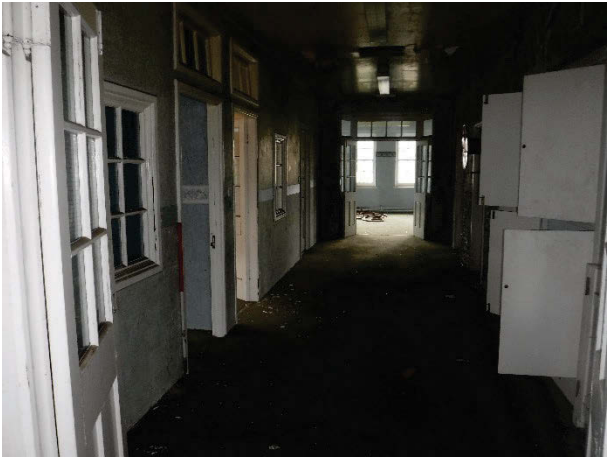
Plate 234 Building 47, Lime, first floor central corridor. Facing south-west. [2076]
