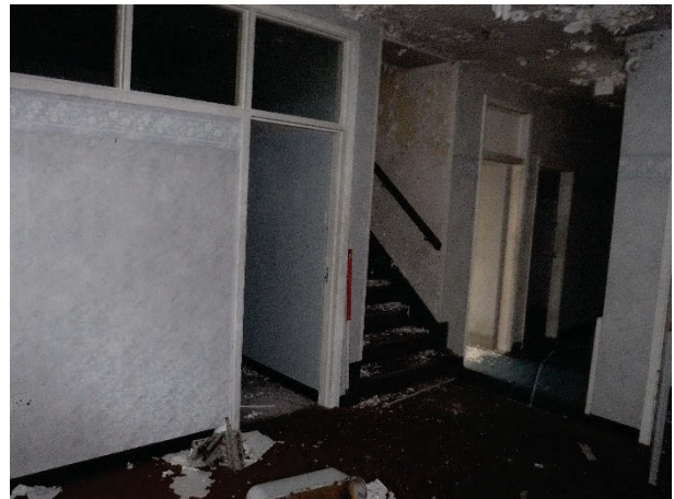
Plate 270 Building 69, Darwin & Seguin, hallway, south-west end. Facing west. [2600]
