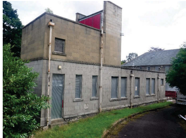
Plate 109 Building 29, Redburn exterior, north-west (front) elevation, middle wing. Facing east. [2455]
