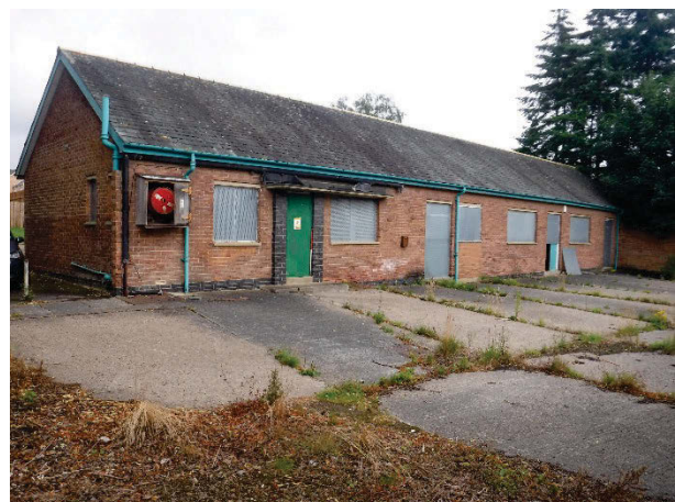
Plate 239 Building 54 external south-east elevation. Facing north. [2351]
