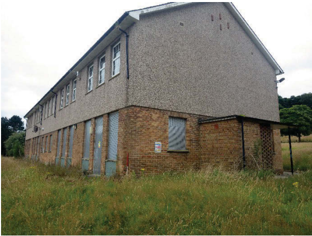
Plate 59 Building 17 Brinkburn east elevation and north gable end. Facing south-west
