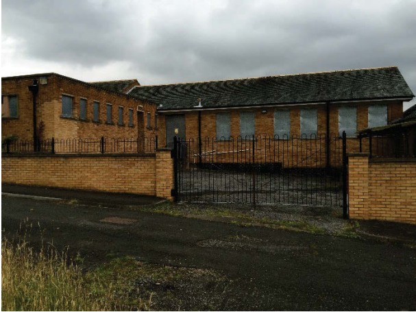
Plate 77 Building 22, Workshops exterior, south-west elevation at south. Facing north. [3050]
