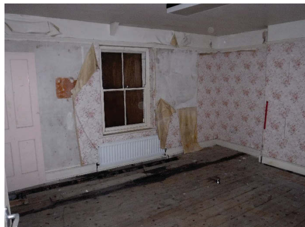
Plate 8 Building 56, Gardener's Cottage interior first floor bedroom 2. Facing north-east. [2278]
