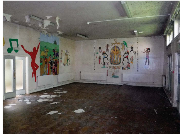
Plate 183 Building 38, main hall. Facing south-east. [1013]
