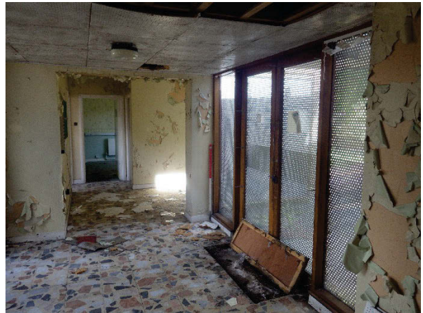
Plate 129 Building 31, McCoull Clinic interior, external doors in projecting wing. Facing south-west. [1814]
