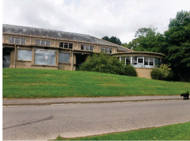
Plate 145 Building 32, recreation Hall exterior east (front) elevation. Facing north-west [2875]
