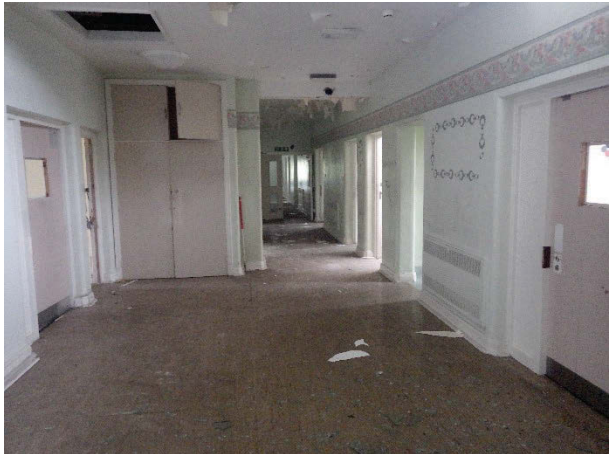
Plate 54 Building 13 Midway West internal hallway Facing south-west [1659]
