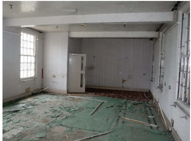
Plate 175 Building 37, Holly/Cedar interior, day room with front door vestibule. Facing south. [2007]
