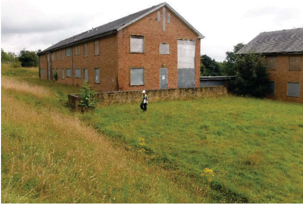
Plate 188 Building 39, Nurses Accommodation north-west (rear) elevation, north block. Facing east. [2795]
