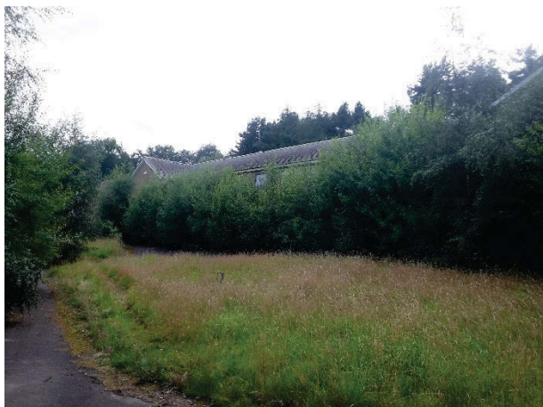
Plate 263 Building 69, Darwin & Seguin, general setting view. Facing west. [2644]
