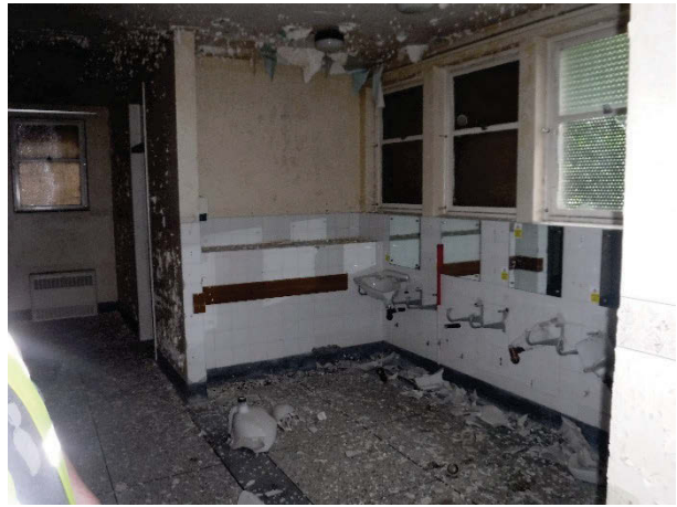
Plate 257 Building 67, Greengates interior central wing lavatory block. Facing north-west. [2762]
