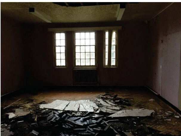
Plate 72 Building 18 Tredgold Hall interior, partitioned Workroom 2. Facing east. [3017]
