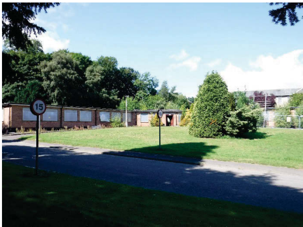
Plate 180 Building 38, general setting view. Facing north-west. [1030]
