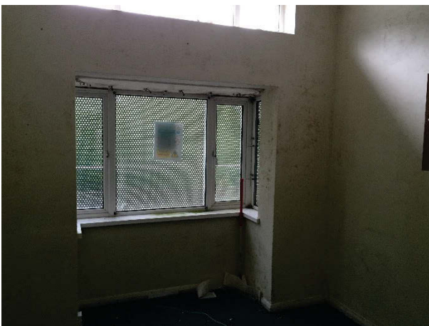
Plate 102 Building 28, Riding interior. "Sisters Room". Facing south-east. [3201]
