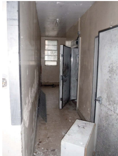
Plate 159 Building 34, Derwent Kitchens and Dining Hall interior, cold stores. Facing north-west. [2528]
