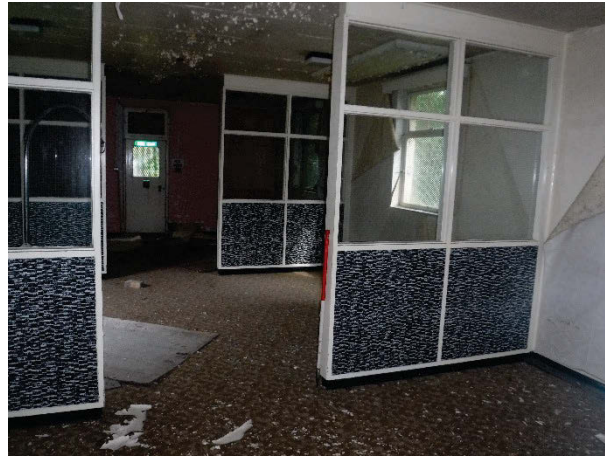
Plate 262 Building 67, Greengates interior north-west wing dormitory. Facing north. [2780]
