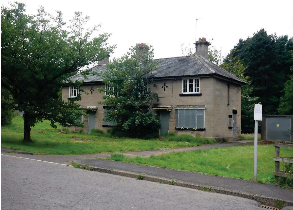
Plate 17 Building 2 General view [#1375]
