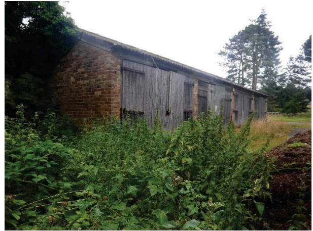
Plate 243 Building 61, exterior general view. Facing north-east. [2831]
