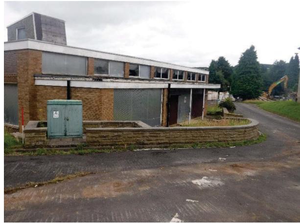
Plate 151 Building 34, Derwent Kitchens and Dining Hall exterior, main access, south-west elevation. Facing east [2555]
