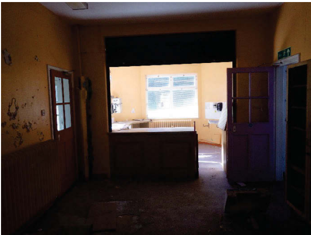
Plate 120 Building 30, The Close, interior reception area. Facing south. [1759]
