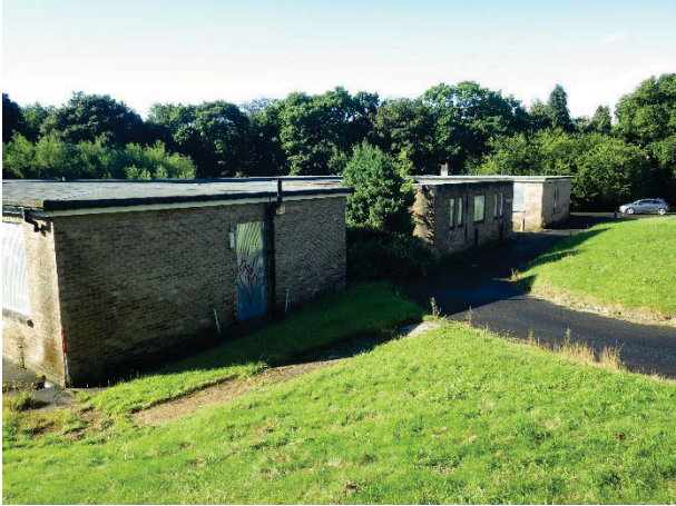
Plate 98 Building 28, Riding exterior general view, north-west (front) elevation. Facing south. [3155]
