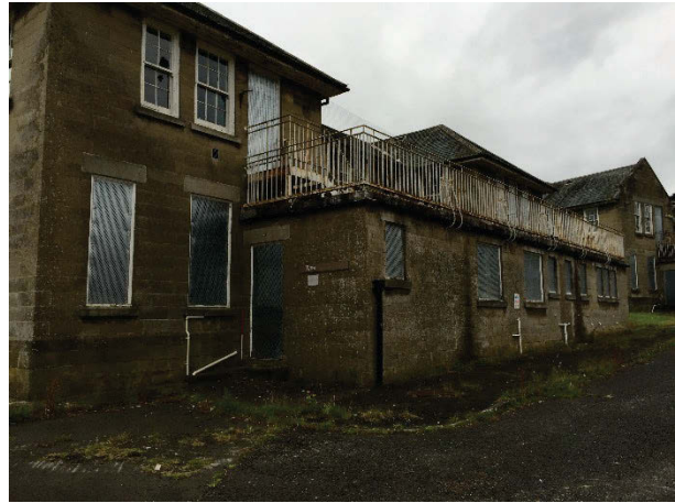
Plate 88 Building 24, Tyne Villa exterior, north (rear) elevation. Facing south-east. [308]
