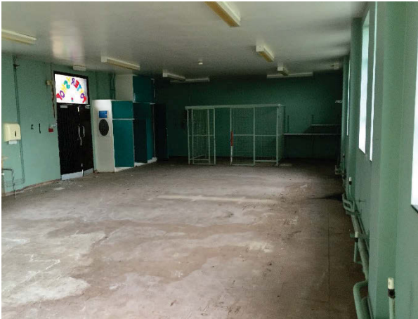
Plate 83 Building 22, Workshops interior, east wing. Facing north-west. [3062]
