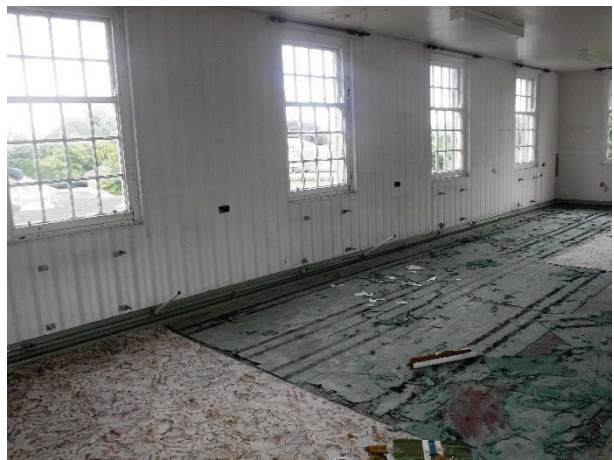
Plate 177 Building 37, Holly/Cedar interior, first floor pavilion wing dormitory. Facing east. [2025]
