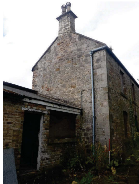
Plate 2 Building 56, Gardener's Cottage exterior, east gable end. Facing south-west. [2288]
