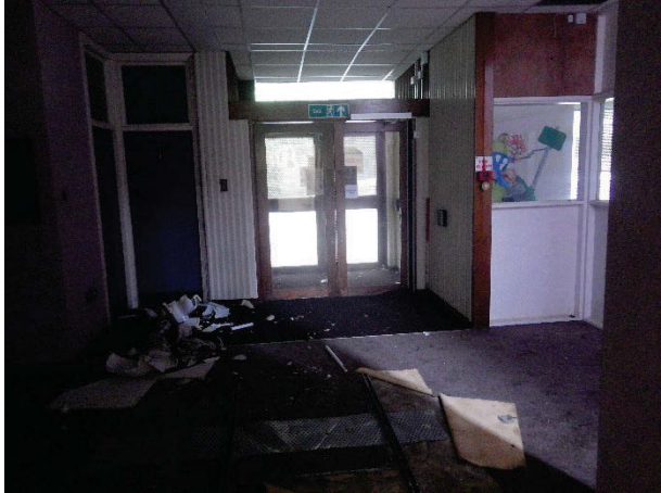
Plate 138 Building 31, McCoull Clinic interior, front block main access hall [1863]
