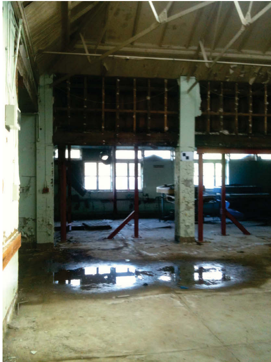
Figure 77 Looking south, across the courtyard, roofed c.1913.
