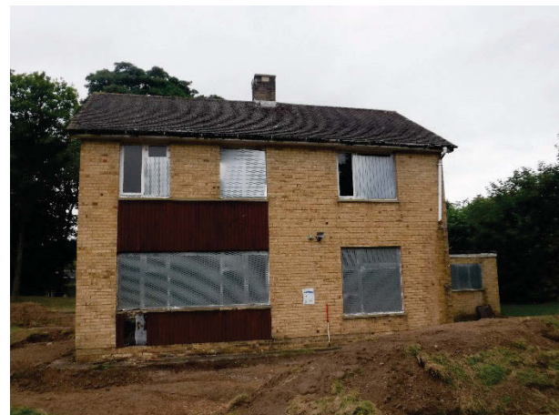
Plate 20 Building 8 Back (south-west) elevation. Facing NE. [1392]
