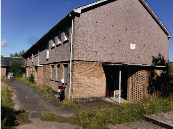
Plate 214 Building 45, Cavell, general view exterior. Facing east. [2707]
