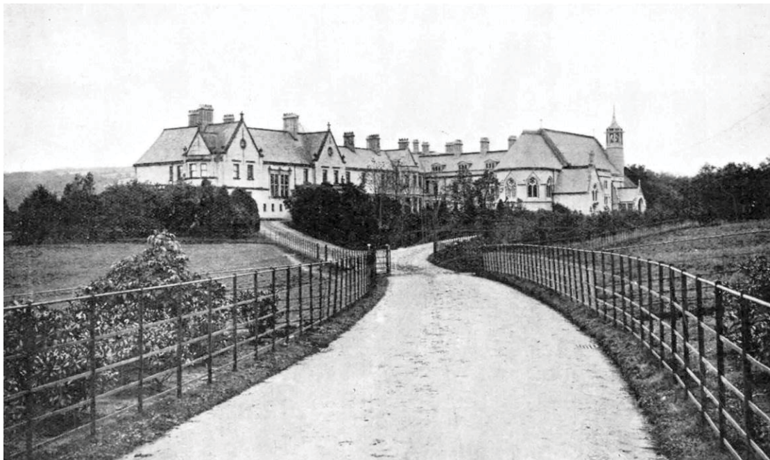
Figure 23 Photograph taken between 1889 and 1904, from the drive looking south. It shows that the drive divided, directing visitors to the church away from the front entrance of the hall. Zielinski 'History of the Parish of Our Lady and St Cuthbert'
