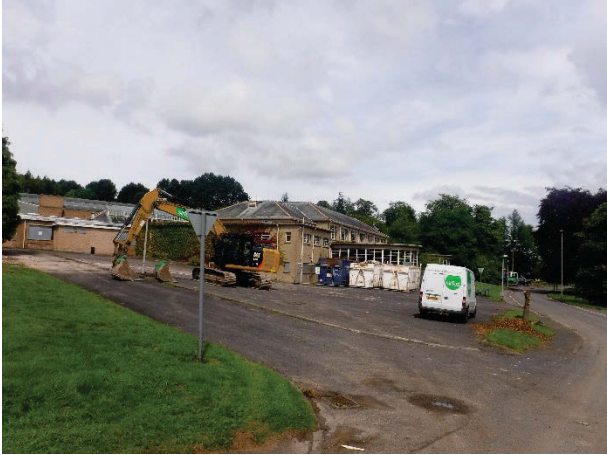
Plate 144 Building 32, recreation Hall exterior general setting shot. Facing north [2870]
