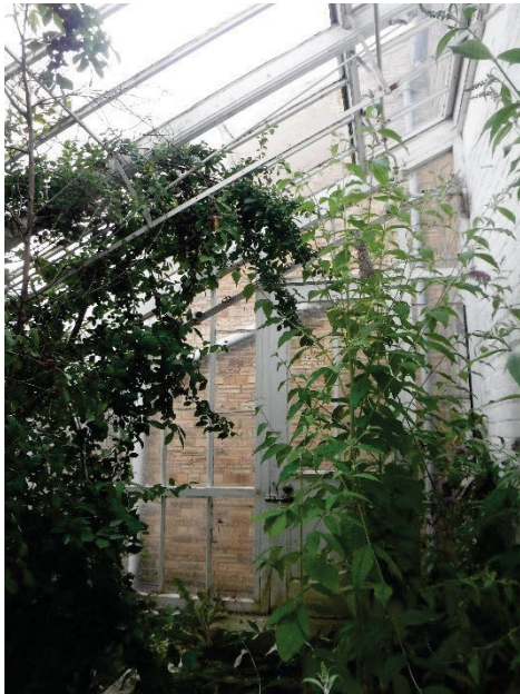
Plate 9 Building 58-60, Glasshouses south-west ('Peach House') interior. Facing south-west. [2294]
