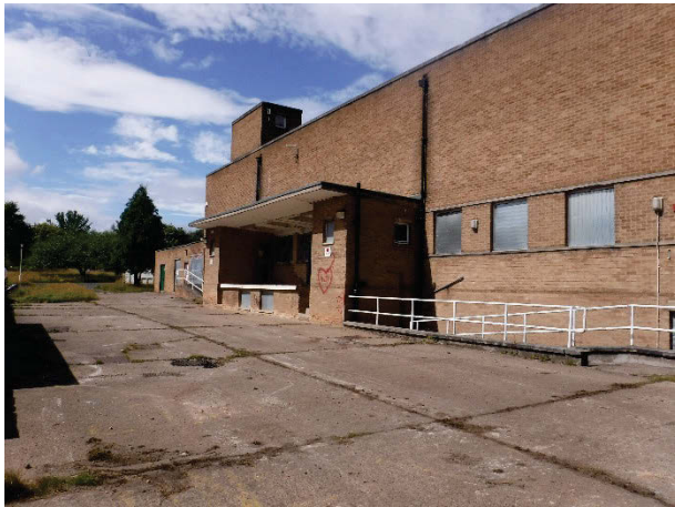
Plate 160 Building 35, Central Stores, exterior south-east elevation. Facing south-west. [1913]
