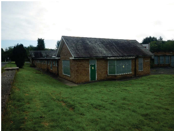
Plate 40 Building 13 Midway/Janie Hepple Unit exterior view. Facing north-east [1523]
