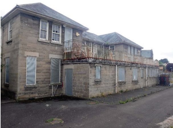
Plate 230 Building 47, Lime, general view exterior west (rear) elevation. Facing south. [2043]
