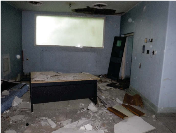
Plate 112 Building 29, Redburn interior. Ground floor operating room. Facing north-east. [2364]
