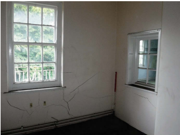
Plate 236 Building 47, Lime, first floor nurse's station. Facing south-east. [2085]
