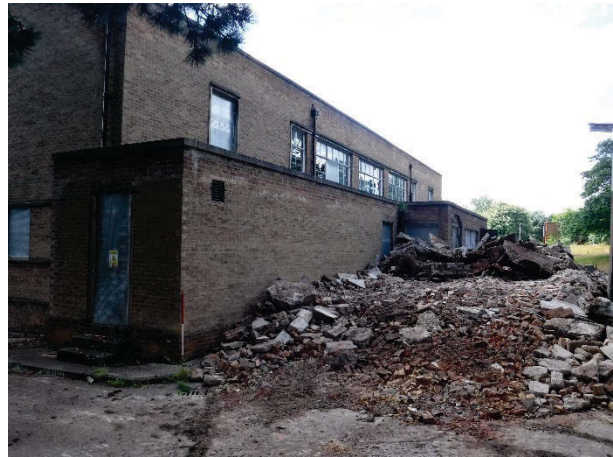
Plate 161 Building 35, Central Stores, exterior north-west elevation. Facing south. [1918]
