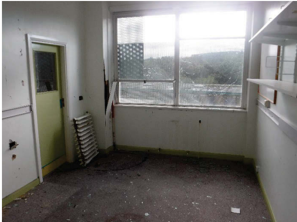
Plate 140 Building 31, McCoull Clinic interior, first floor partitioned laboratory room. Facing north-east [1890]
