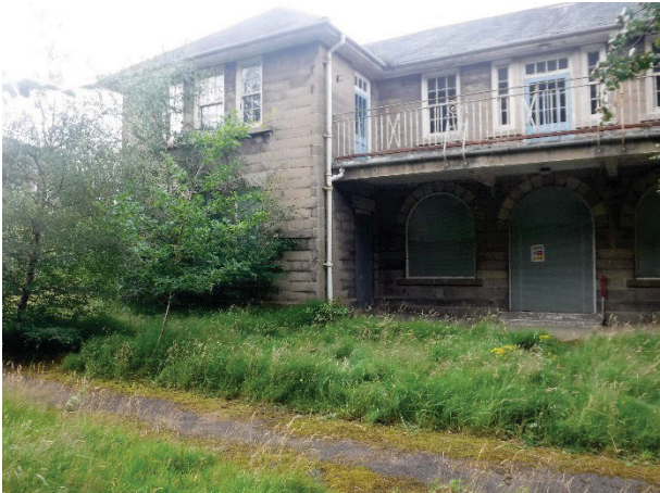
Plate 228 Building 47, Lime, general view exterior east (front) elevation. Facing west. [2037]
