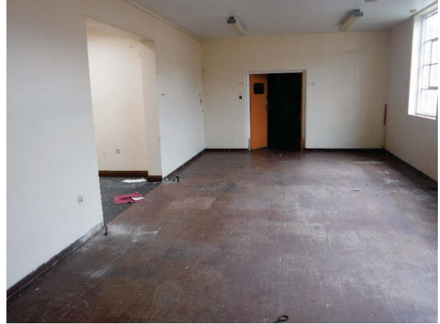
Plate 209 Building 44, Patients' Shopping Centre, general view room g21, 'steam press'. Facing south. [2120]
