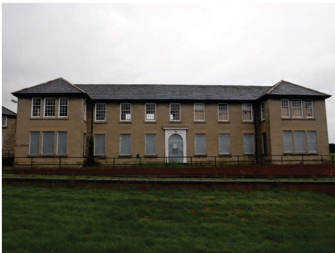
Plate 85 Building 23, Skerne Villa, external south-east elevation. Facing north-west. [1401]
