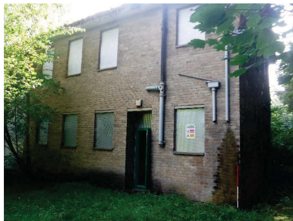
Plate 264 Building 69, Darwin & Seguin external south elevation. Facing south. [2638]
