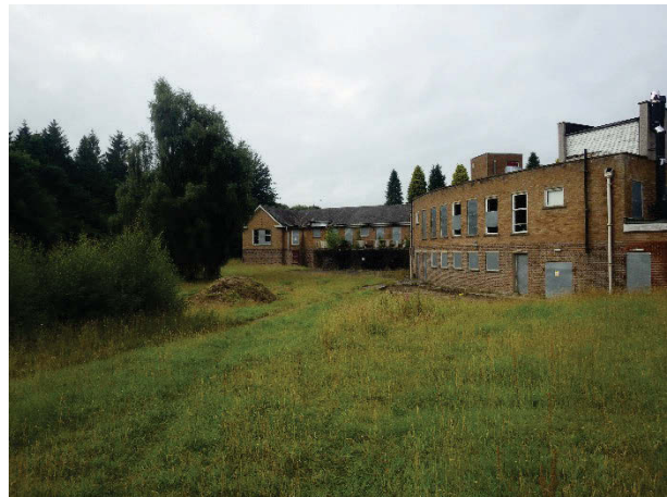
Plate 41 Building 13 Midway/Janie Hepple Unit exterior view, rear elevation. Facing south [1533]
