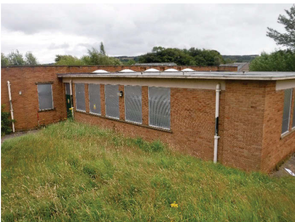
Plate 206 Building 44, Patients' Shopping Centre, external north and west elevations. Facing south-east. [2091]
