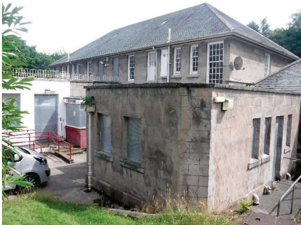
Plate 108 Building 29, Redburn exterior, north-west (front) elevation. Facing east. [2443]
