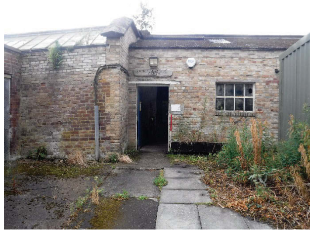
Plate 14 Building 58-60, Potting sheds signed entrance. Facing south-east. [2306]
