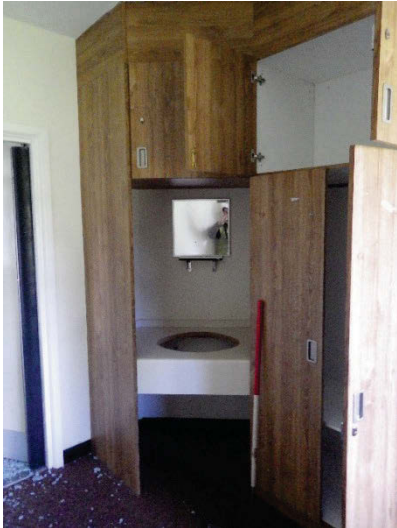
Plate 28 Building 7 Stephenson House Dormitory Room with surviving fittings [1441]
