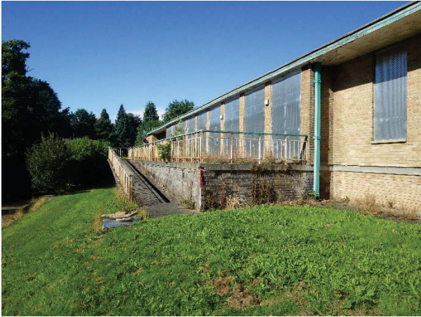
Plate 126 Building 31, McCoull Clinic exterior, south-east (back) elevation. Facing south-east. [1796]
