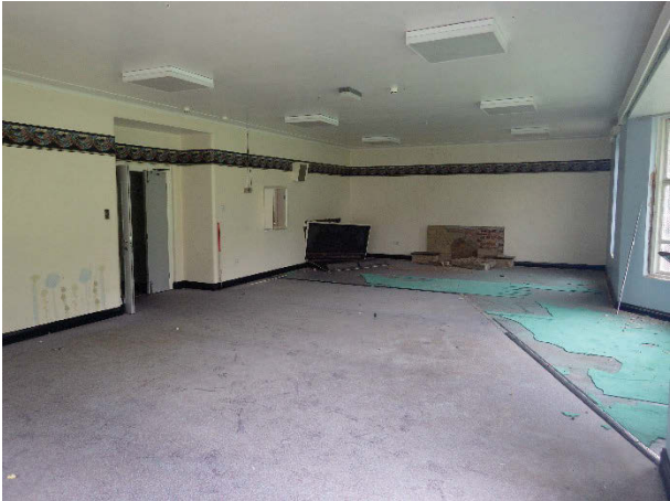
Plate 50 Building 13 Midway West dayroom. Facing east [1628]
