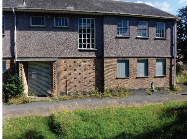
Plate 215 Building 45, Cavell, general view exterior. Facing east. [2708]
