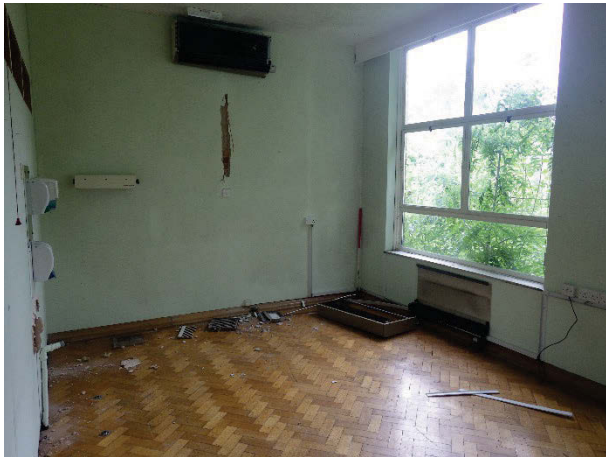
Plate 132 Building 31, McCoull Clinic interior, subdivided ward room. Facing south. [1835]
