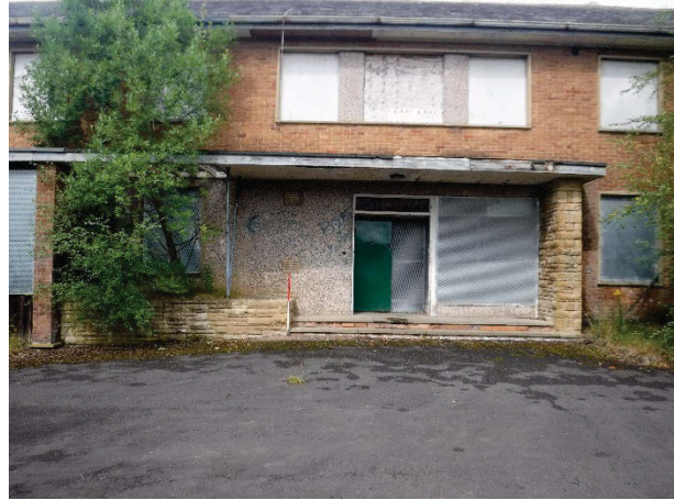
Plate 187 Building 39, Nurses Accommodation external south-east (front) elevation. Facing north-west. [2786]
