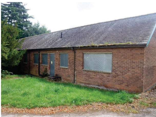
Plate 238 Building 54 external north-west elevation. Facing east. [2853]
