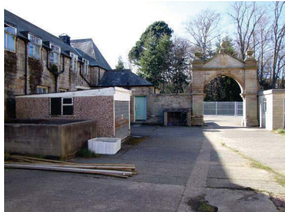
Figure 74 The service court looking north towards the entrance arch.
