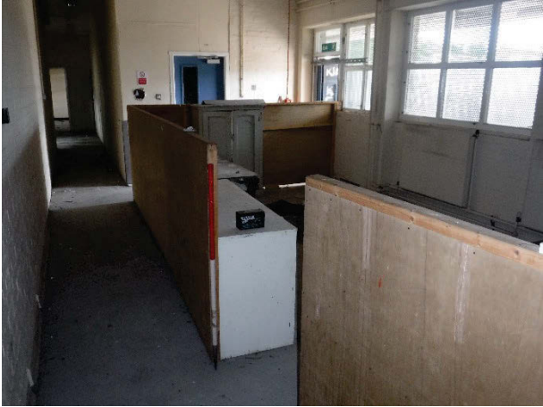
Plate 162 Building 35, Central Stores, interior office area. Facing east. [1960]
