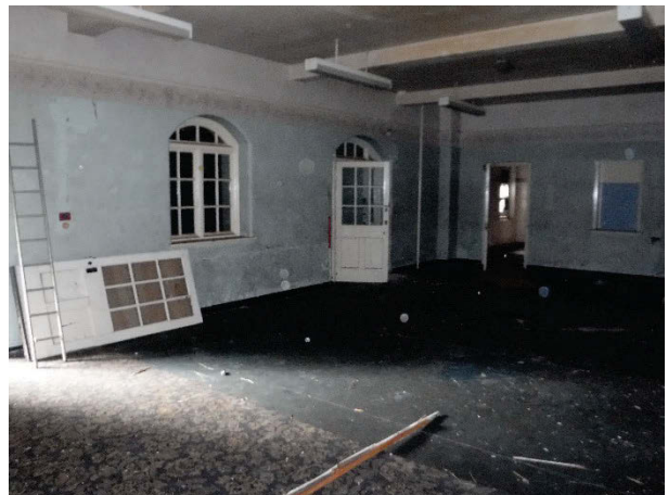
Plate 231 Building 47, Lime, interior dining room. Facing north-west. [2050]
