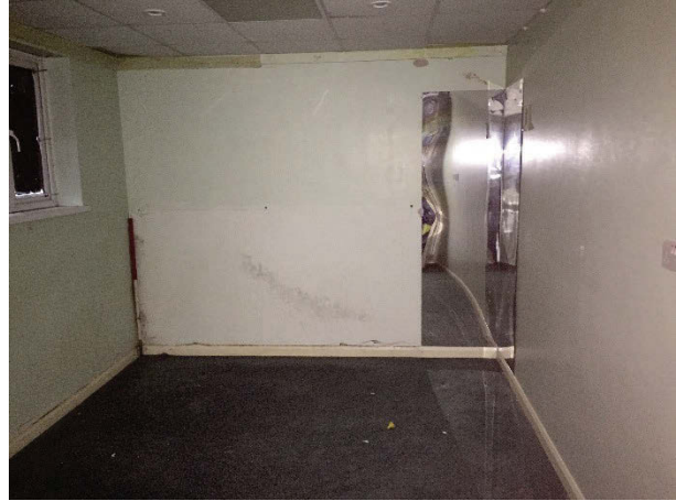
Plate 105 Building 28, Riding interior. Subdivided "Playroom". Facing south-east. [3208]
