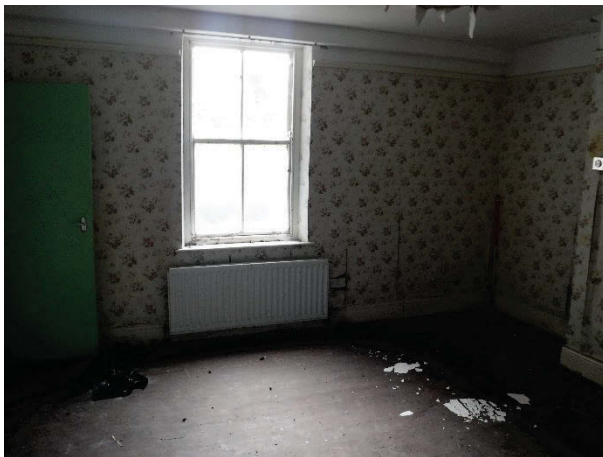
Plate 5 Building 56, Gardener's Cottage interior ground floor living room. Facing south. [2270]
