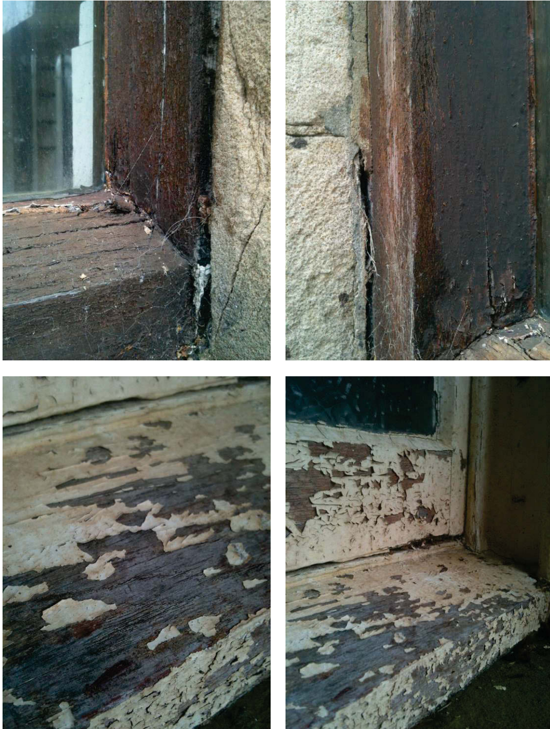
Figure 43 Ground storey windows showing possible red-brown original colour.
