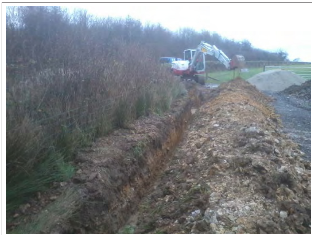
Plate 12: View of example section of cable trench - Area 3
