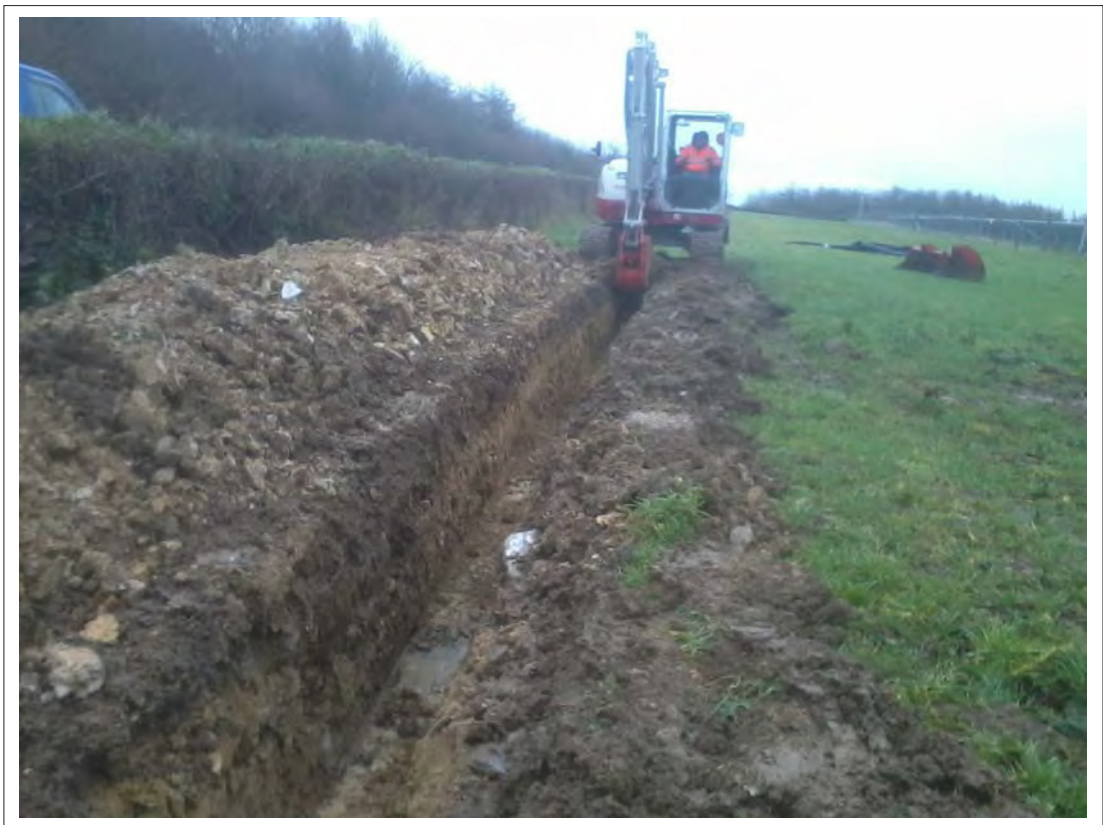
Plate 13: Example view of cable trenching, Area 3.
