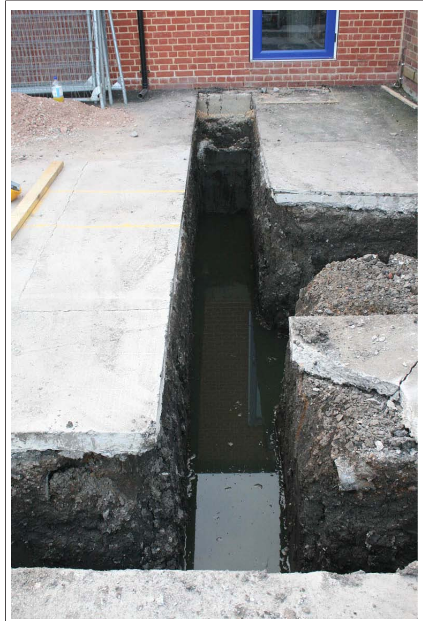
Plate 14: View east along completed southerly foundation trench
