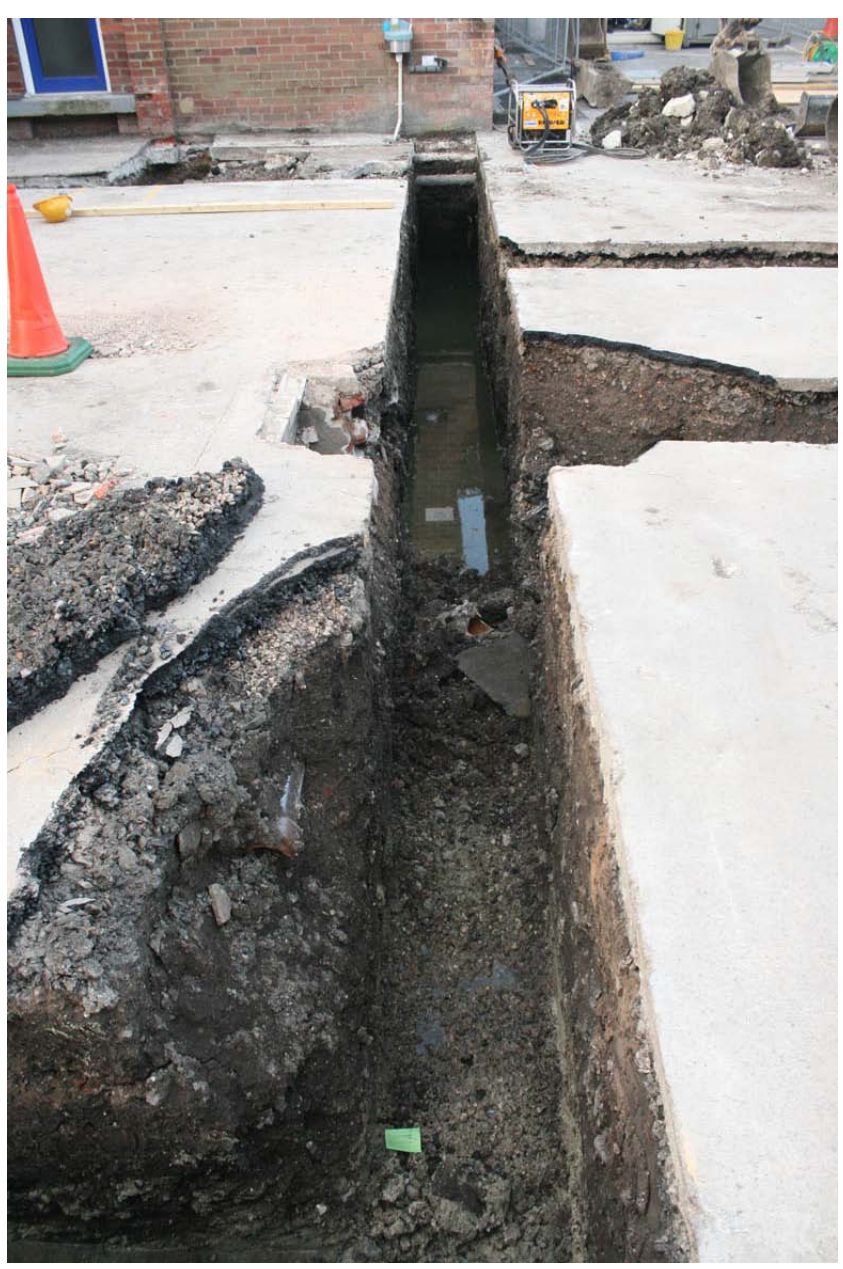
Plate 13: View south along completed westerly foundation trench
