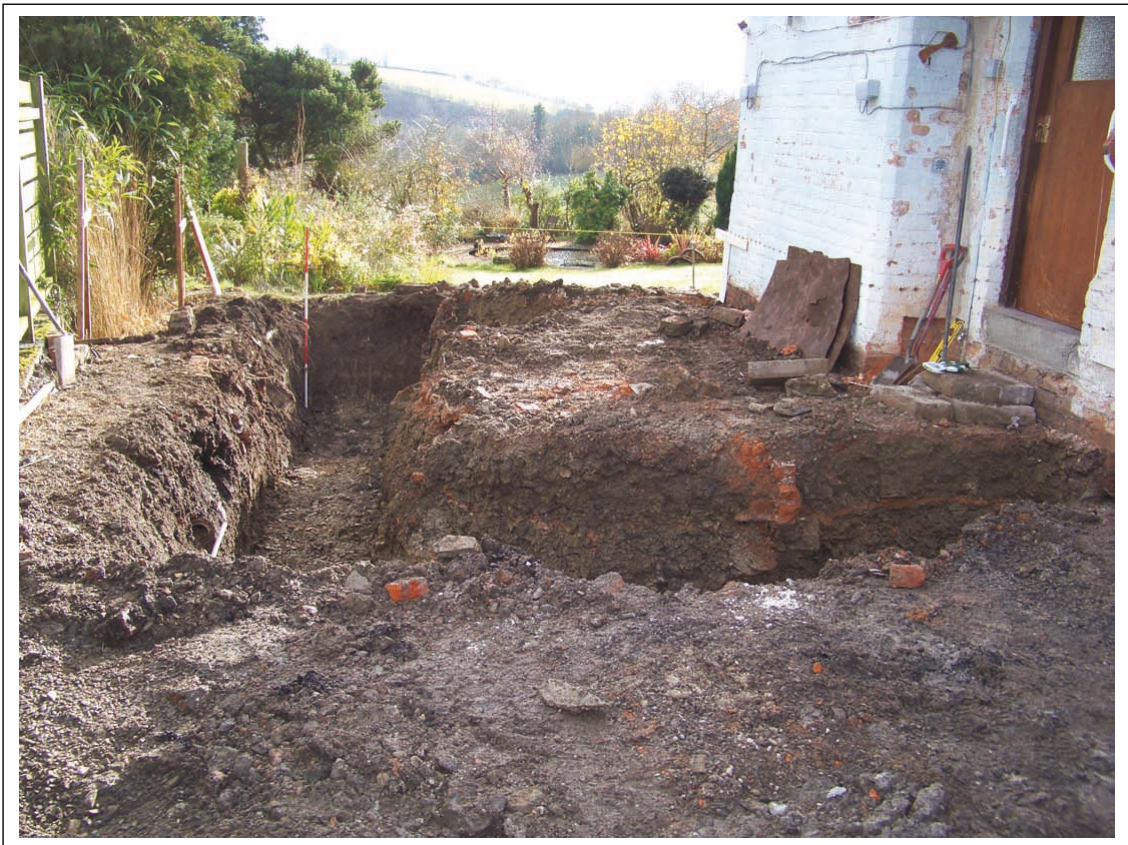
Plate 7 - Overall Shot of Excavation. Looking S. Scale 2m.
