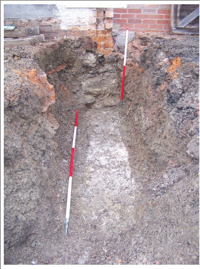
Plate 3 - Footings of Mistress Yard Wall in Area B. Looking W. Scale 1m x 2m.
