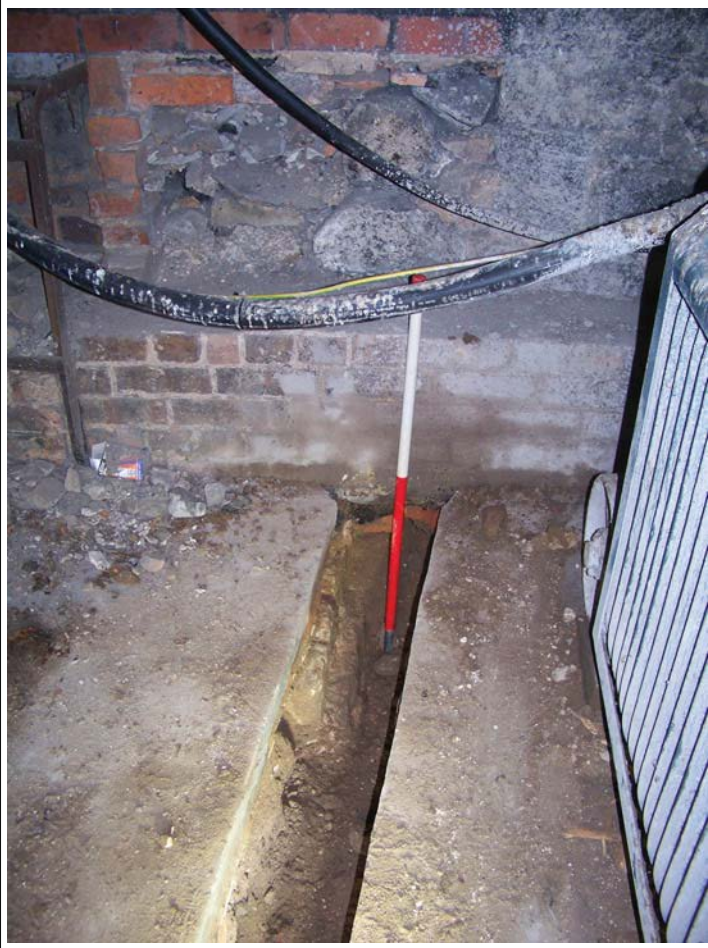
Plate 13. Possible Buttress (16) in Transformer Room. Looking East. Scale 1x1m
