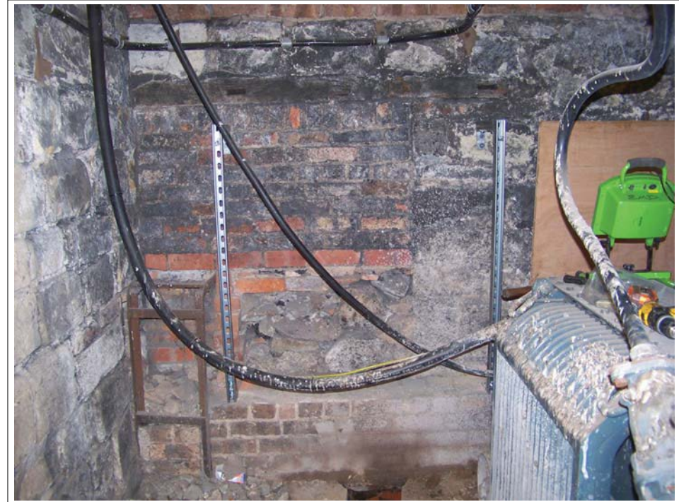
Plate 14. Transformer Room Wall with Brackets Fitted. Looking East.
