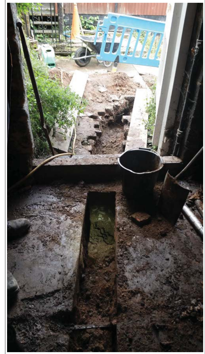
Plate 12. Transformer Room Threshold. Looking West.
