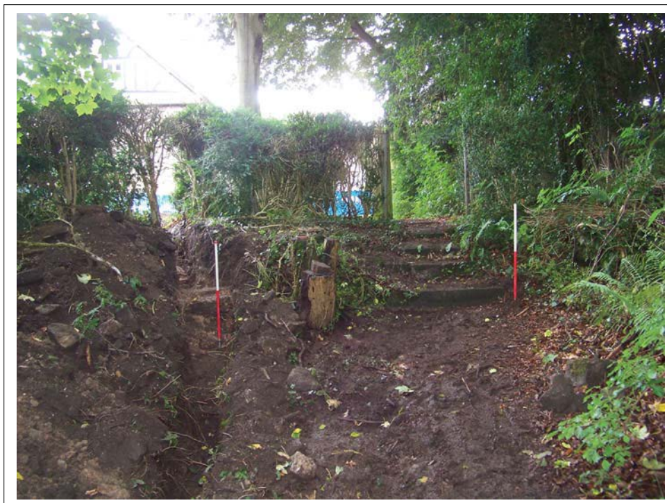
Plate 3. Overall Shot, Wall 03 on Left, Steps on Right. Looking South. Scale 2x1m
