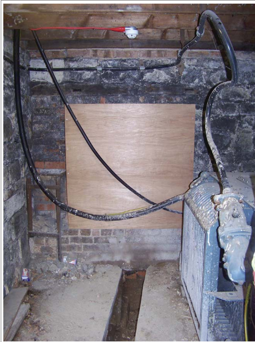
Plate 15. Transformer Room Wall with Board Fitted. Looking East.
