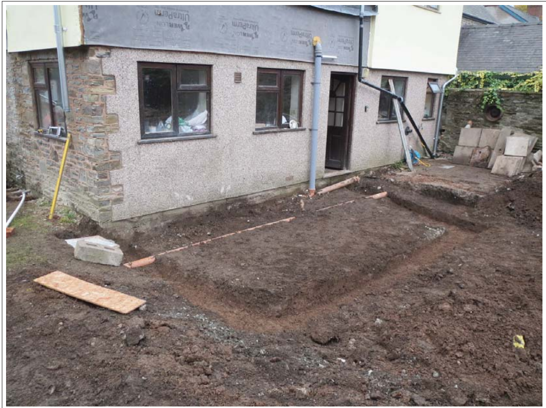
Plate 10. Area B: post-ex shot of foundations for the sunroom. Looking southeast.
