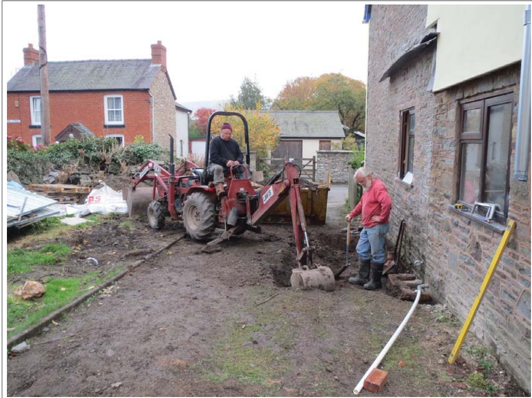
Plate 13. Area C: working shot of excavations for the porch. Looking east-northeast.
