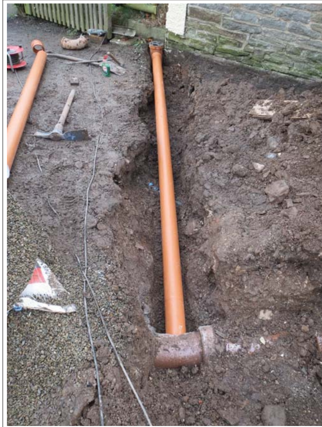
Plate 15. Excavations for drainage towards the front of Lake House. Looking southeast.
