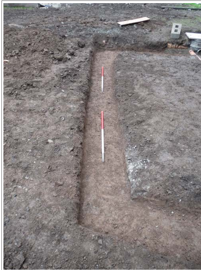
Plate 11. Area B: post-ex shot along the western side of foundations for the sunroom. Scales: 2x1m. Looking north-northwest.
