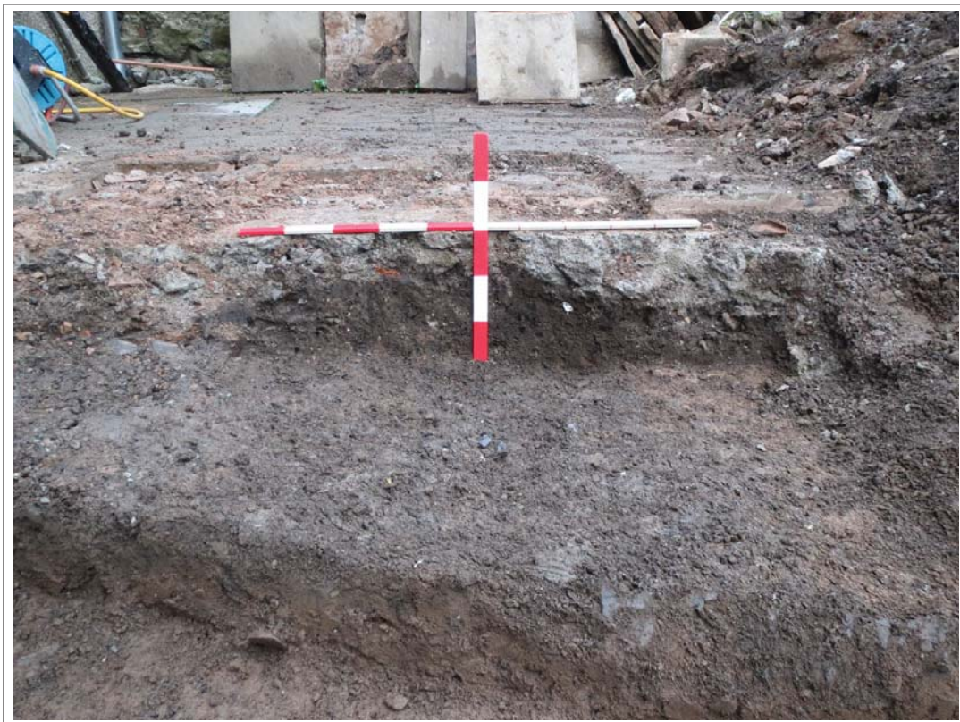
Plate 12. Area B: representative section of the excavation area for the sunroom, showing natural silty clay (202) below a disturbed soil layer (201) and concrete slab (200). Scales: 1x0.5m & 1x1m. Looking south-southeast.
