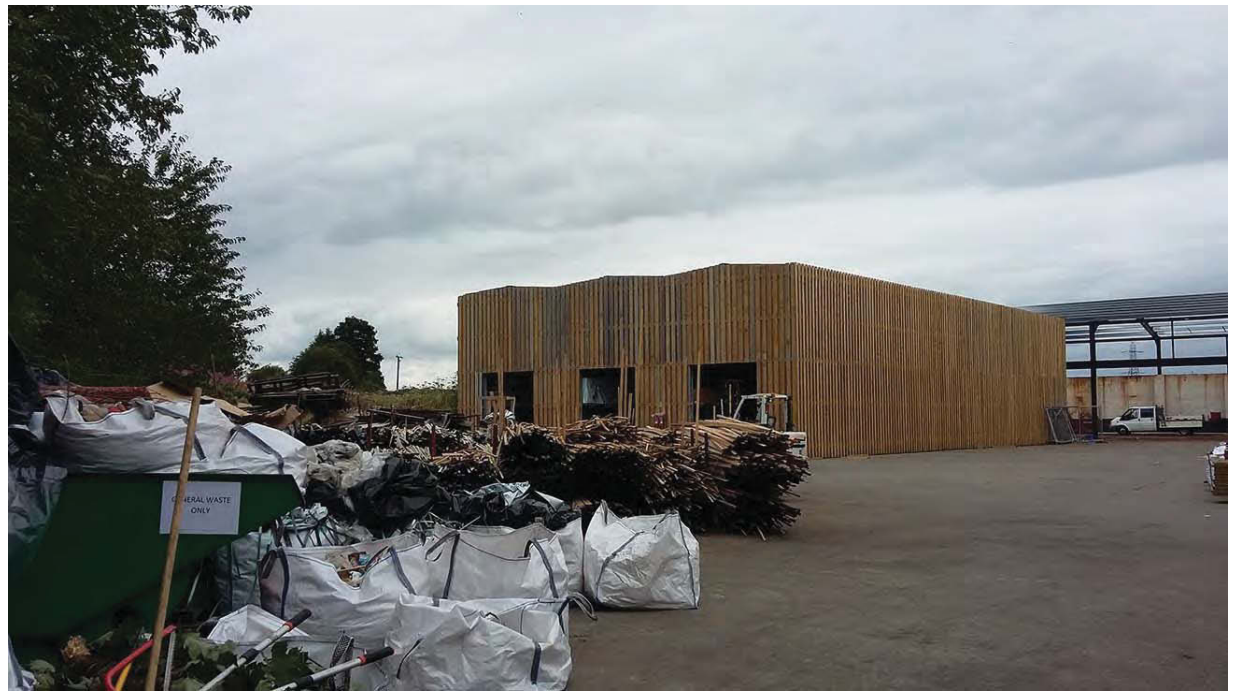
Plate 1. The front and southwest side of the new industrial unit, looking northeast
