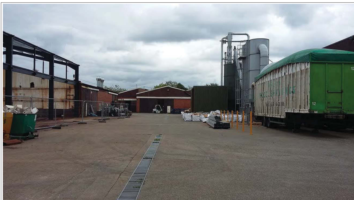
Plate 4. General view of the industrial estate from the front of the new unit, looking south-southeast
