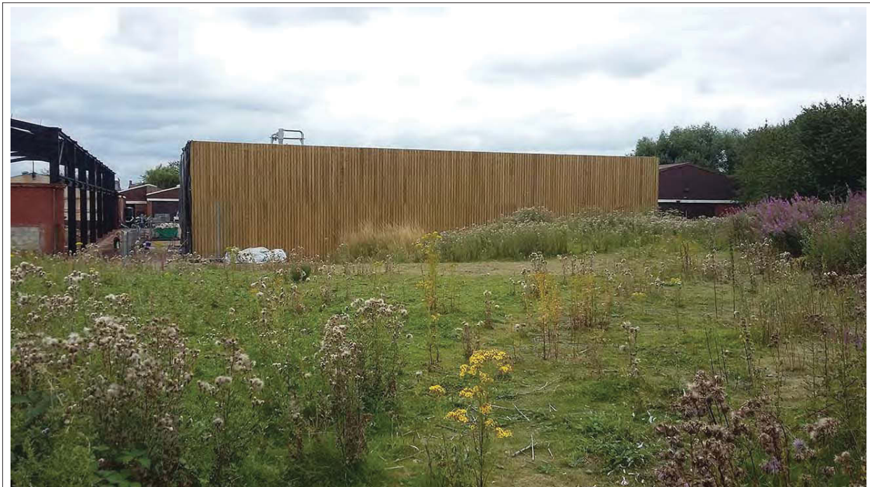
Plate 2. The rear elevation of the industrial unit, looking south-southeast
