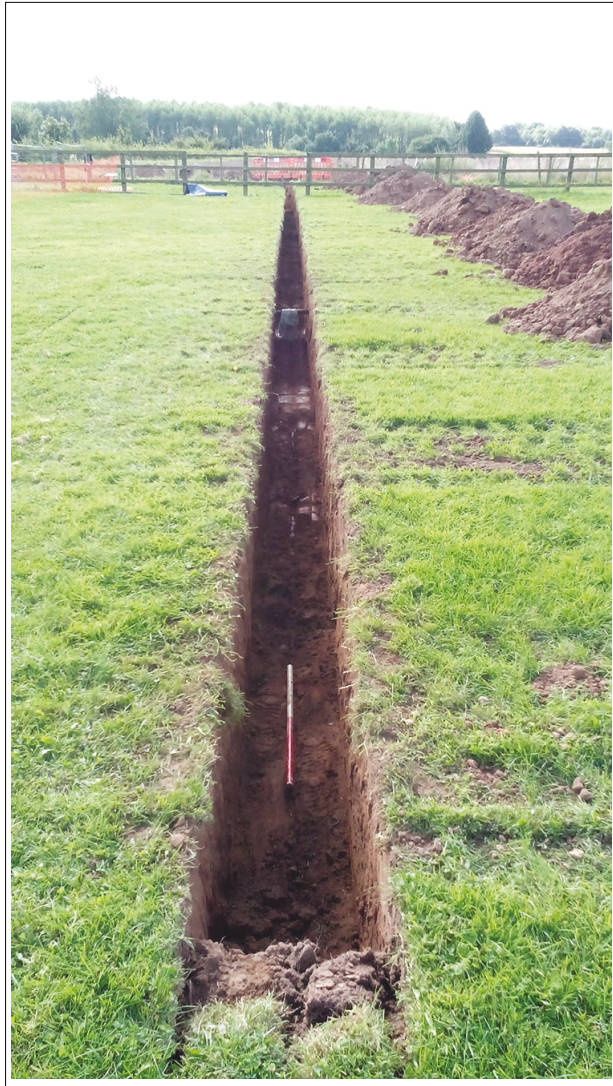
Plate 11. Shot along Cable Trench, looking south. Scale 1m
