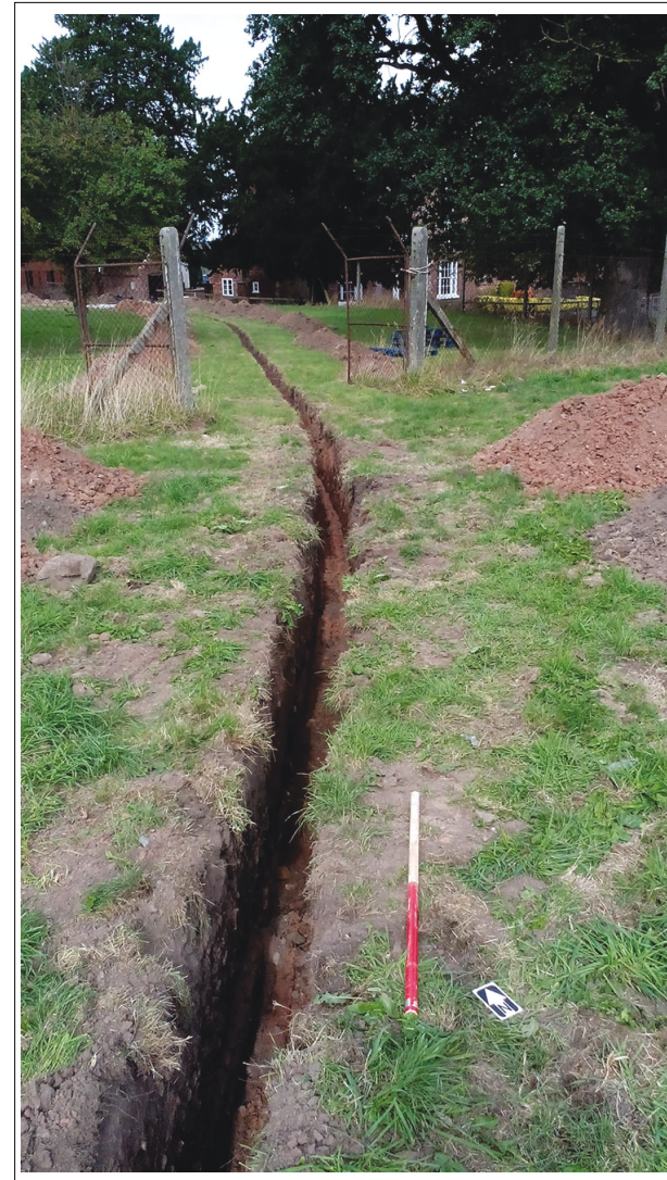
Plate 12. Shot along Cable Trench, looking north. Scale 1m
