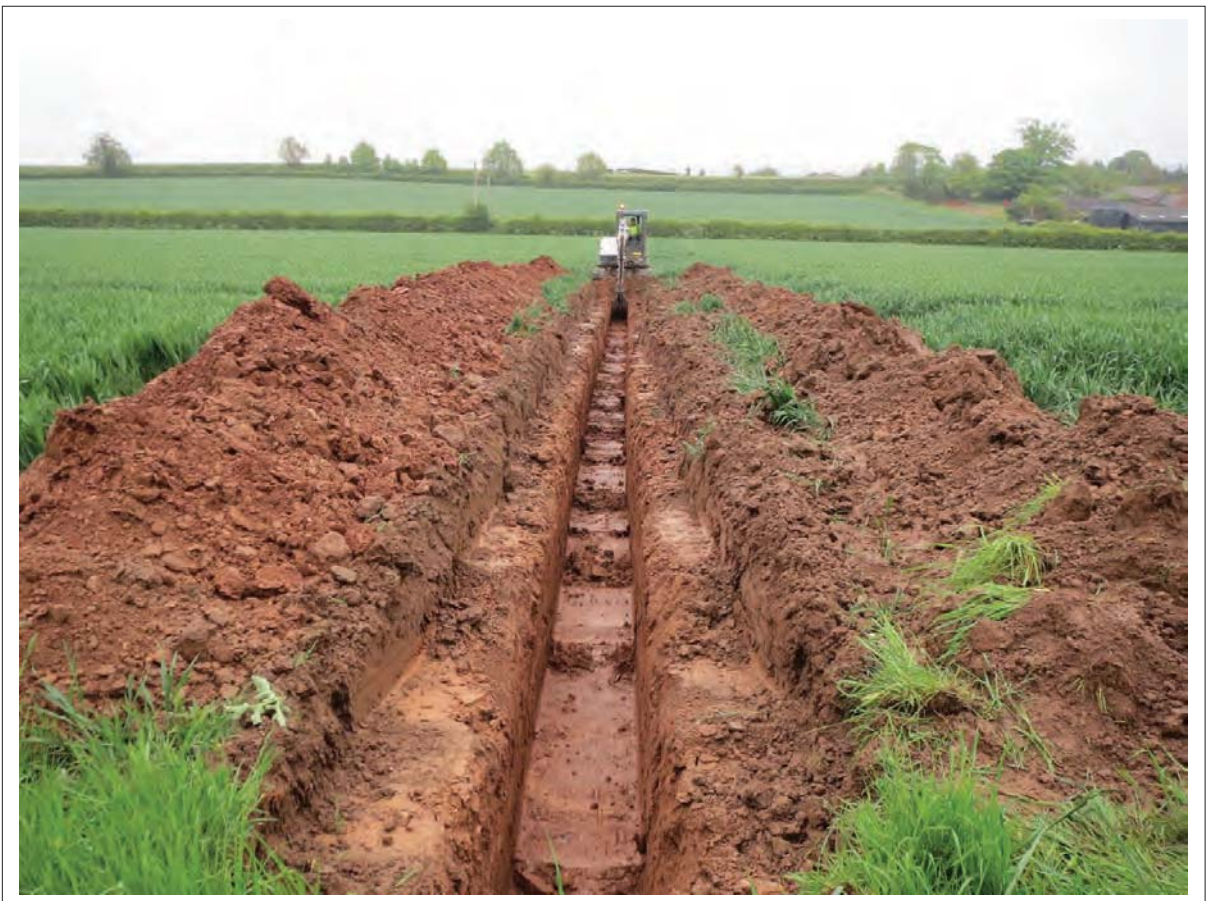
Plate 8: View north west of cable trench cutting in Area 3
