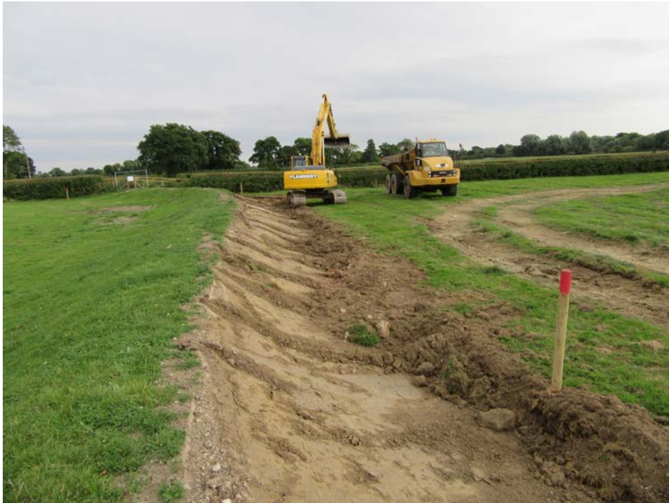
Plate 7. East facing view of flood embankment site strip
