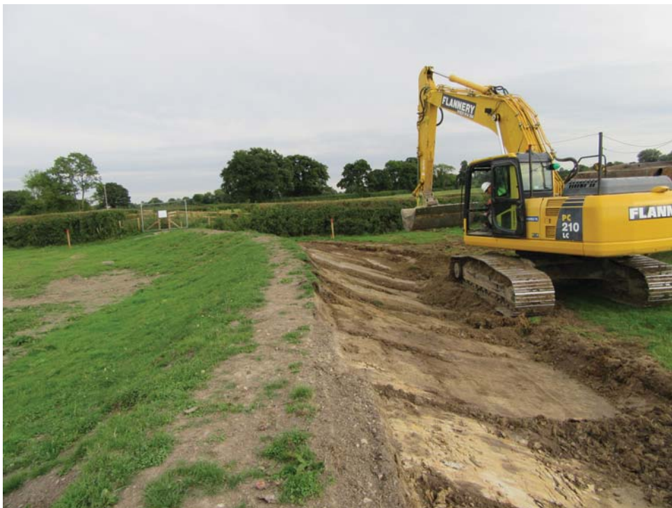
Plate 6. East facing view of flood embankment site strip
