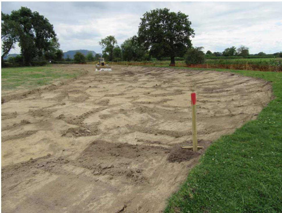
Plate 8. East facing view of flood embankment site strip
