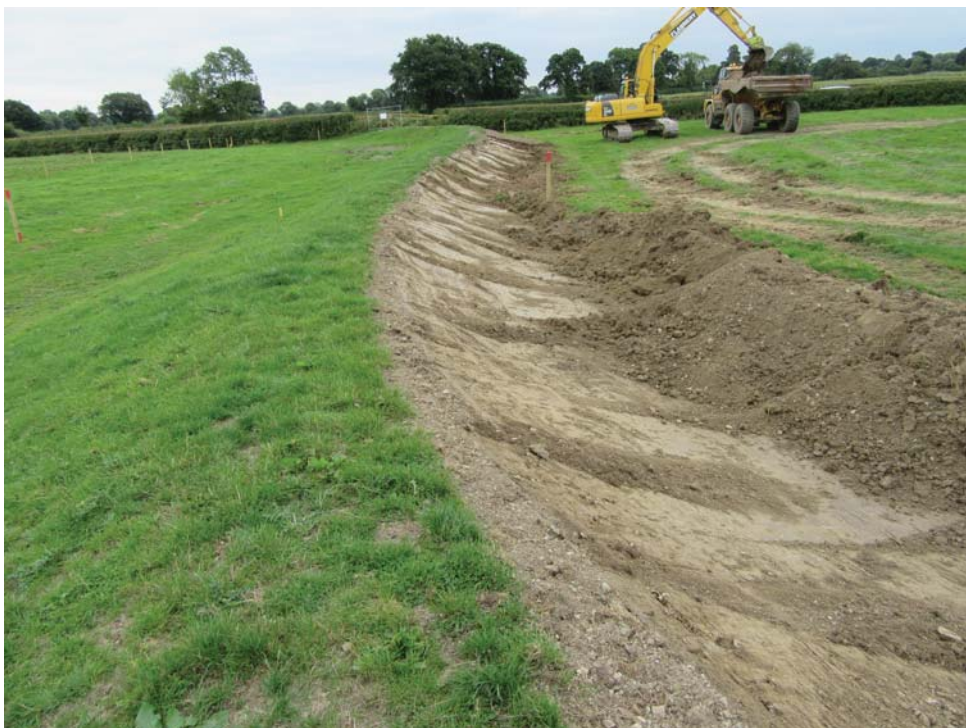
Plate 4. East facing view of flood embankment site strip
