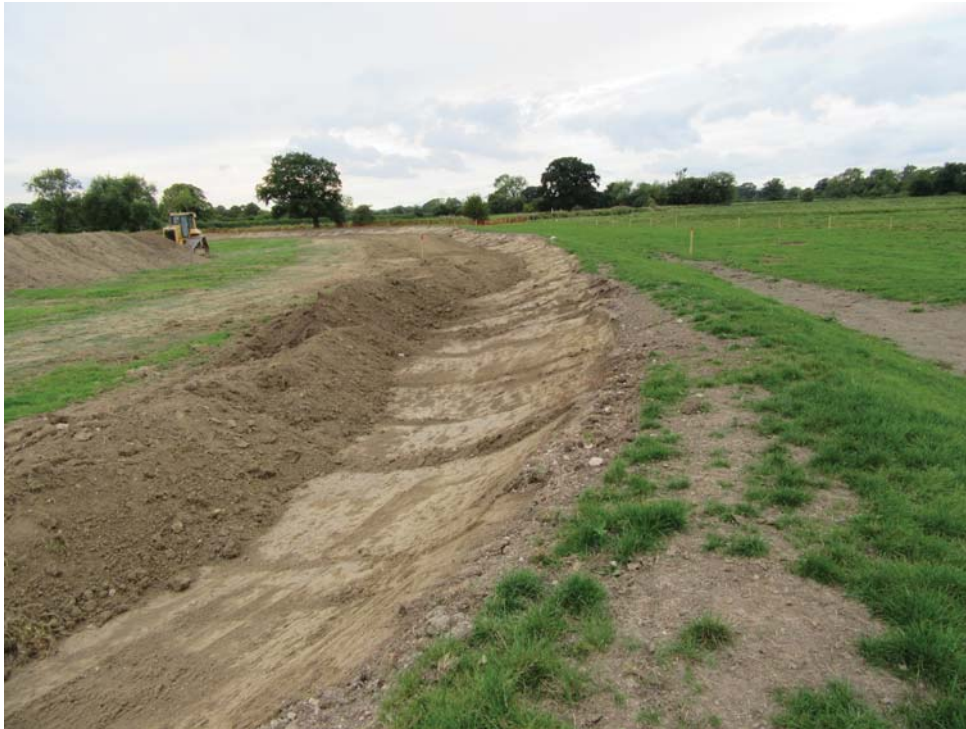
Plate 3. South facing view of flood embankment site strip
