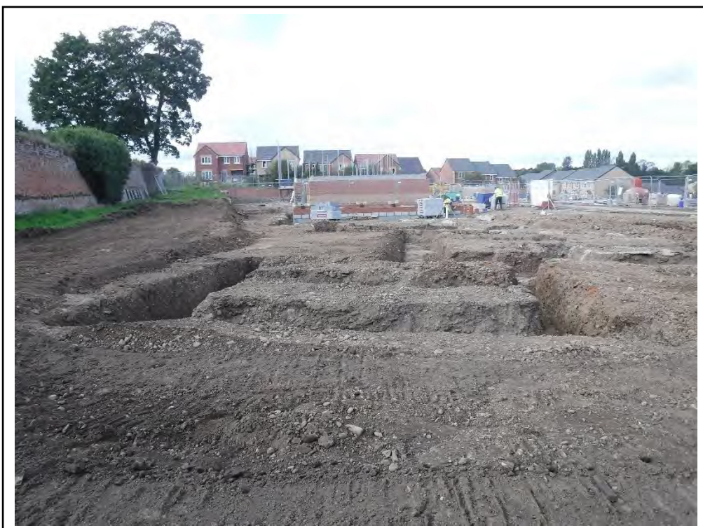
Plate 30 (2016): Layout of Plot 270 with house and garage footings in Area B after excavation; View facing W
