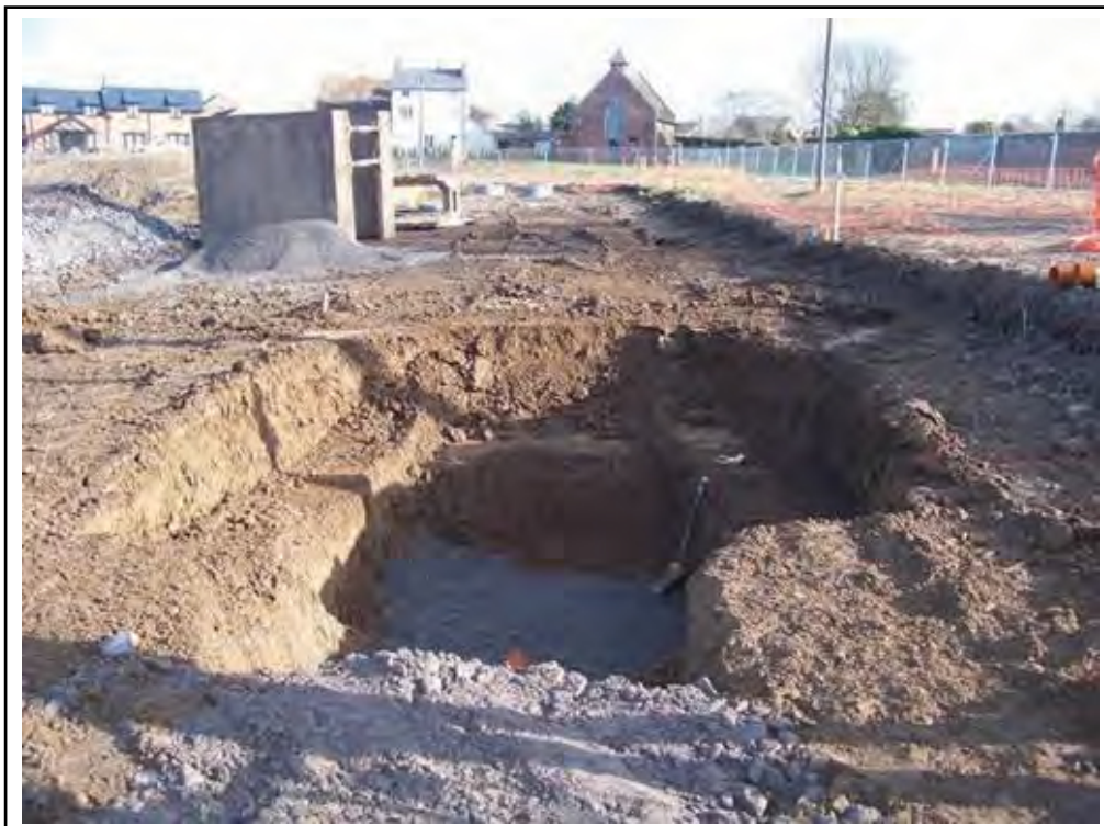
Plate 27 (Intervention 2014): Excavation of Manhole Pit for drainage during Watching Brief; View facing E
