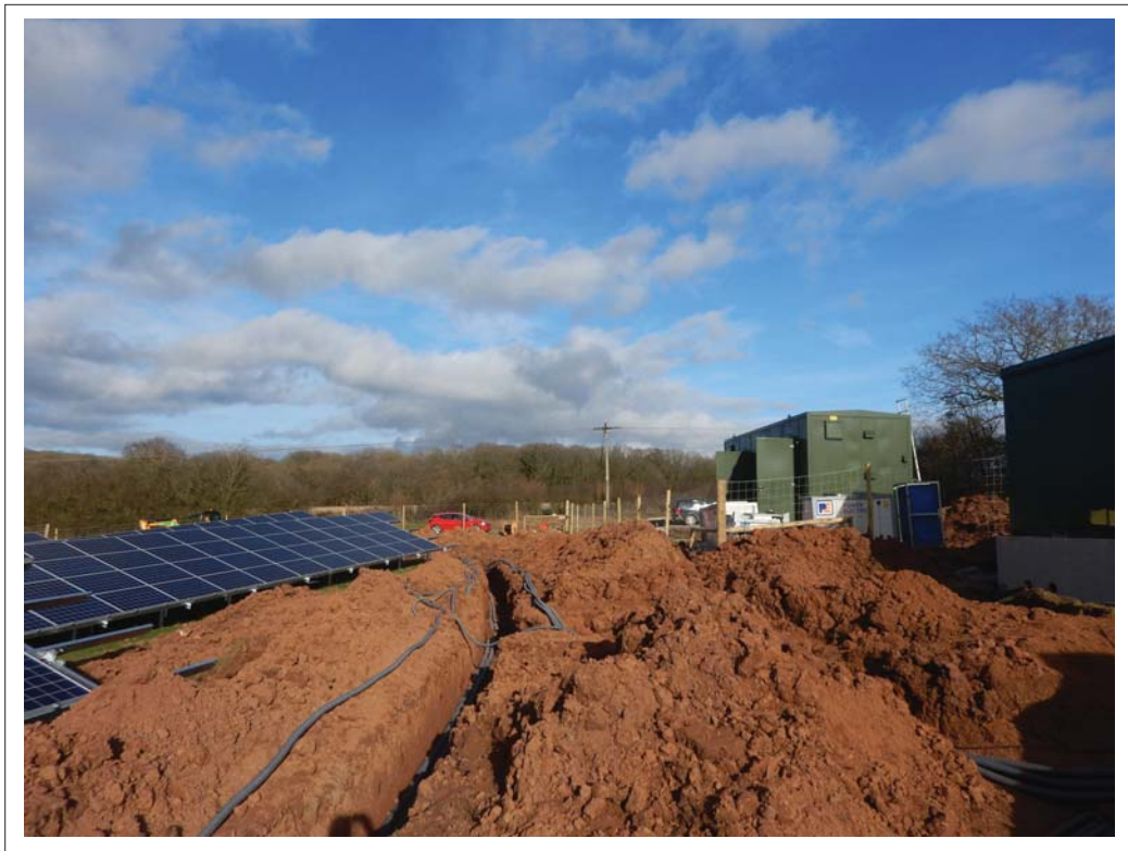
Plate 11. General shot of cable trenches within Field 2. Looking east
