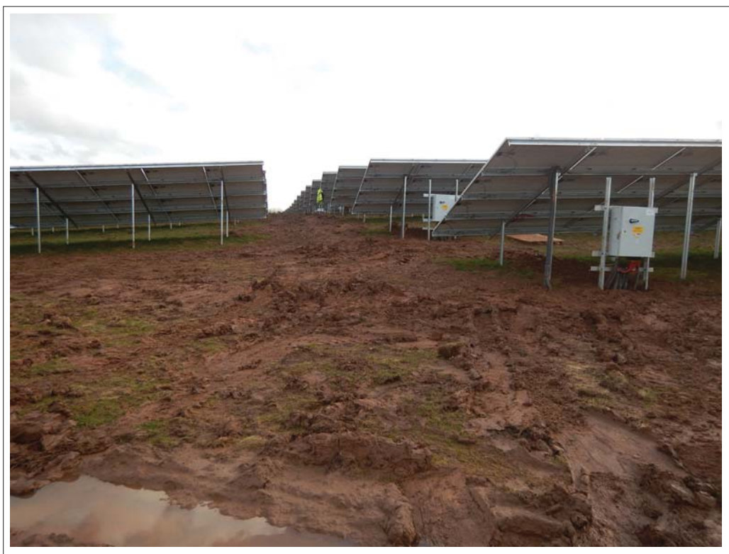
Plate 4. General view of backfilled cable trenches within Field 1. Looking south
