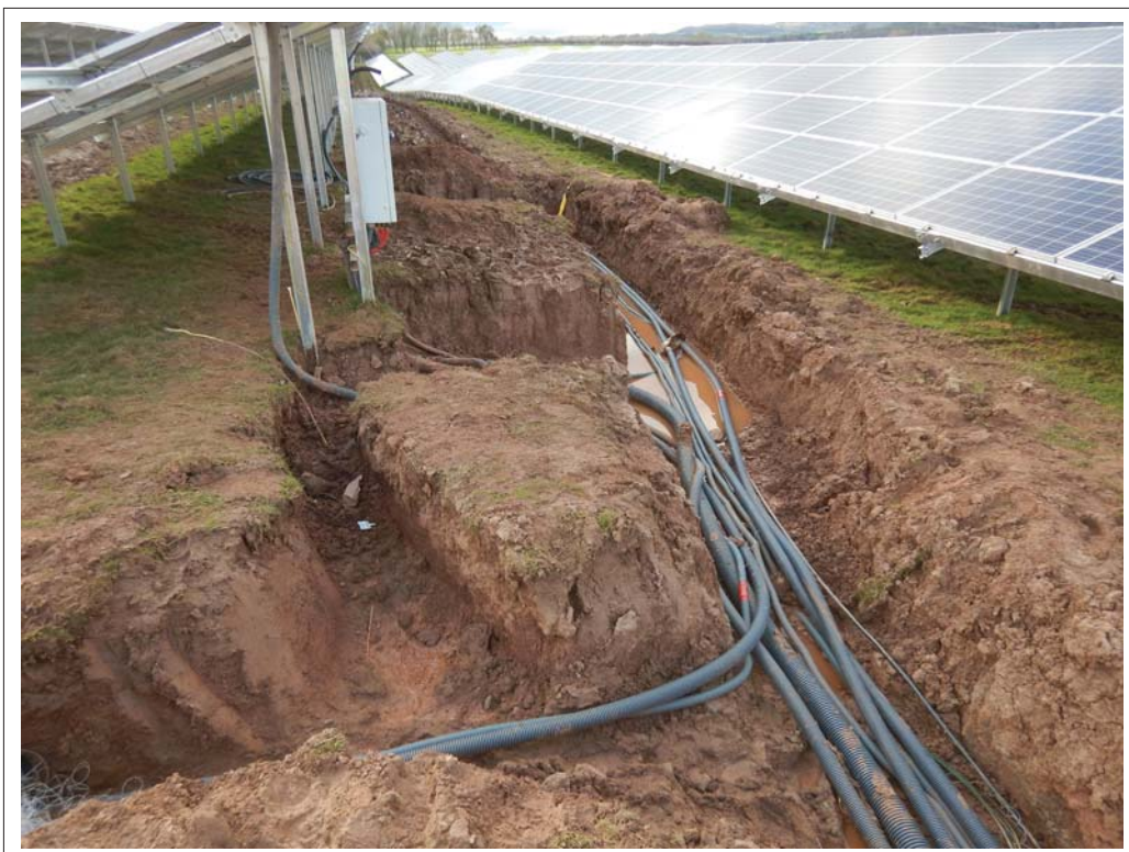
Plate 3. General view of cable trenches within Field 1. Looking west
