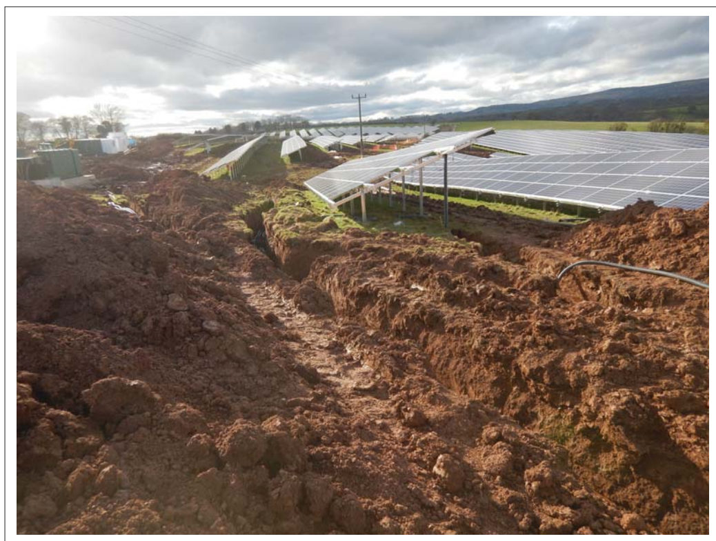
Plate 10. General shot of cable trenches within Field 2. Looking west
