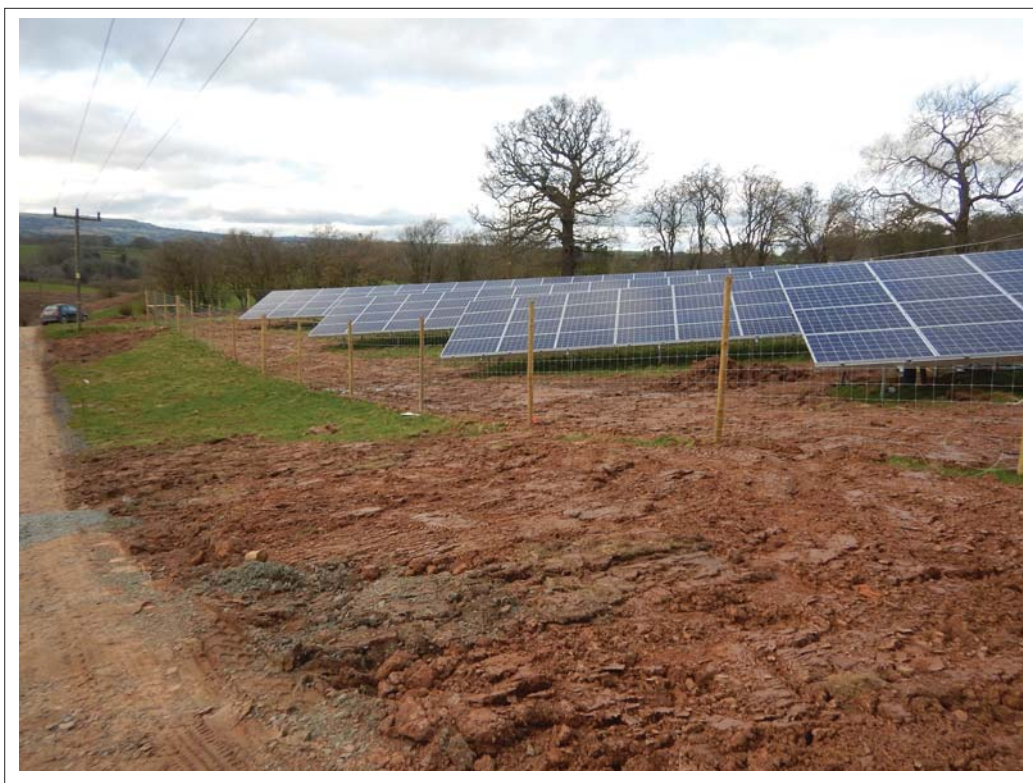
Plate 9. Shot of backfilled cable trenches within Field 2. Looking north
