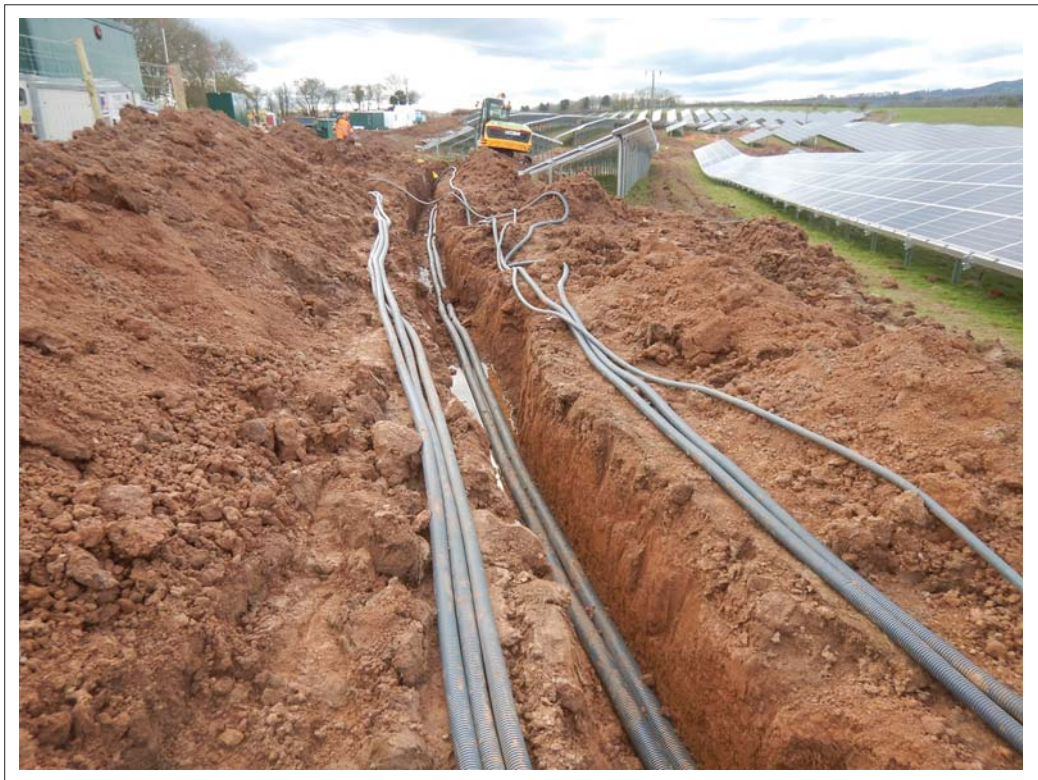
Plate 12. General shot of cable trenches within Field 2. Looking west
