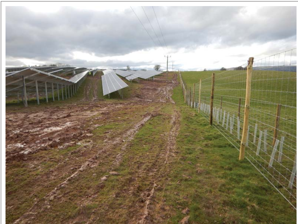
Plate 1. General shot of backfilled cable trenches within Field 1. Looking west
