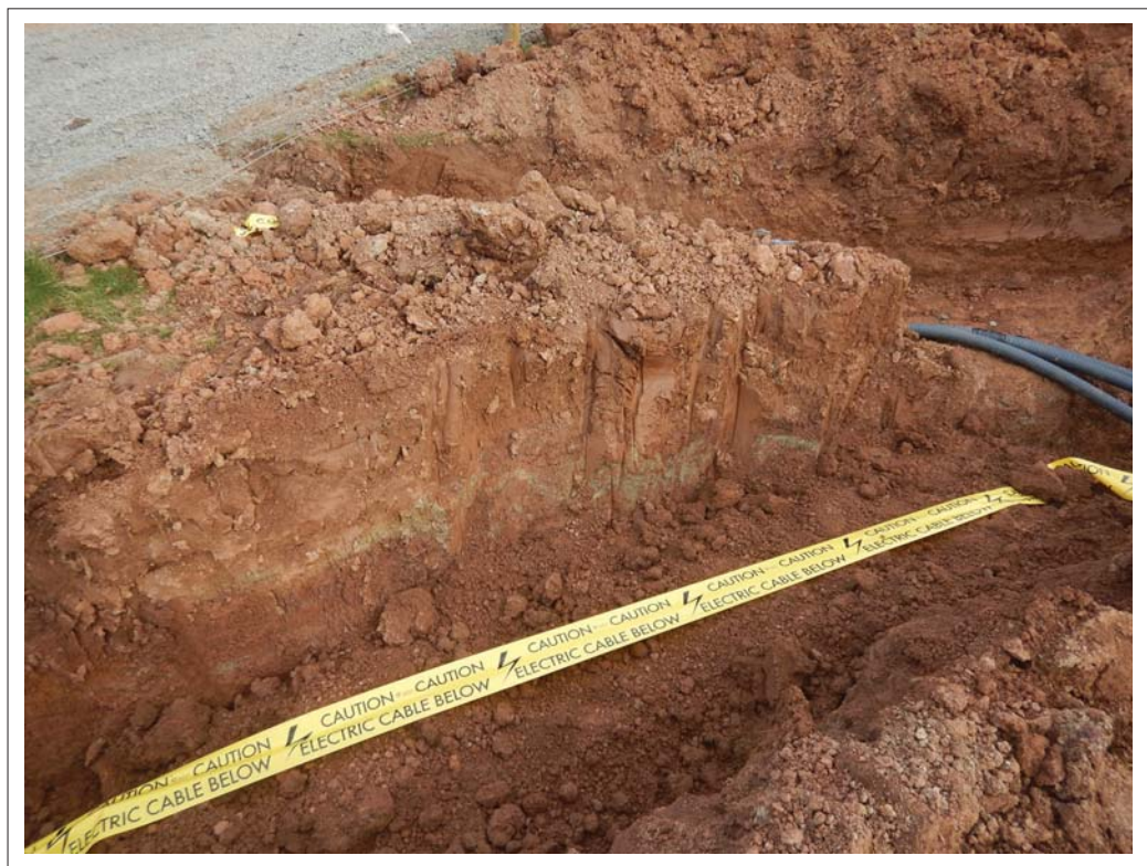
Plate14. Close up of partly backfilled cable trench within Field 2.
