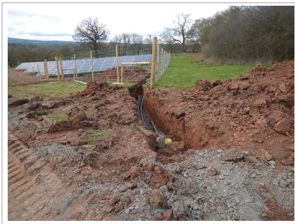
Plate 8. Shot of cable trenches within Field 2. Looking north
