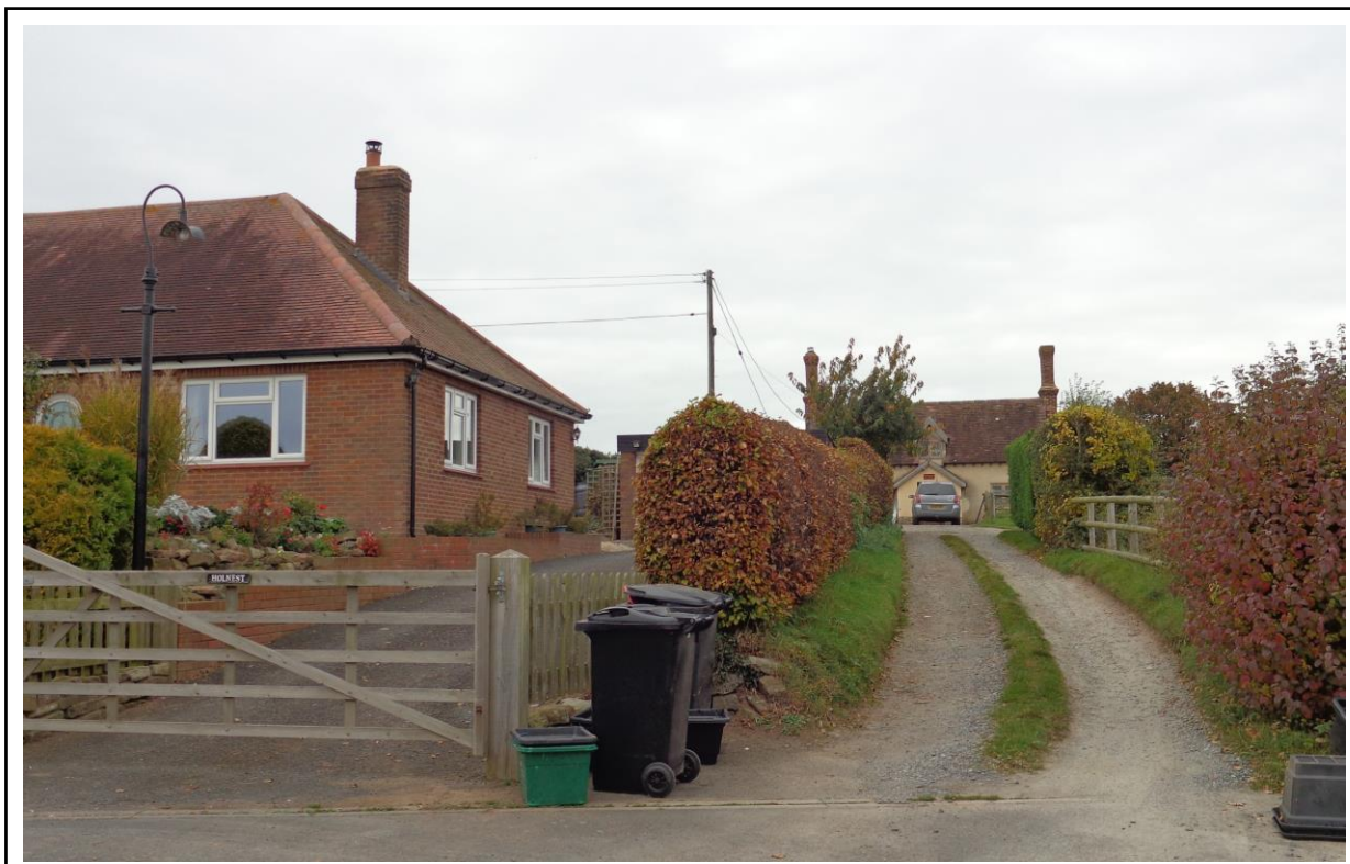
Plate 70: Dodmore Cottage, MSA 15780 at the background. Shot facing northwest.
