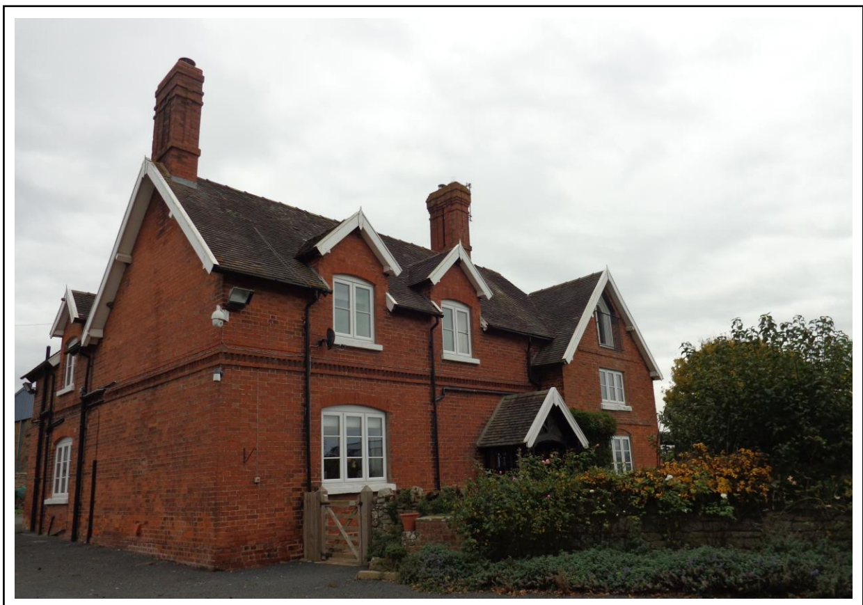
Plate 68: Rock Farm farmhouse, MSA 15497. Shot facing southeast.
