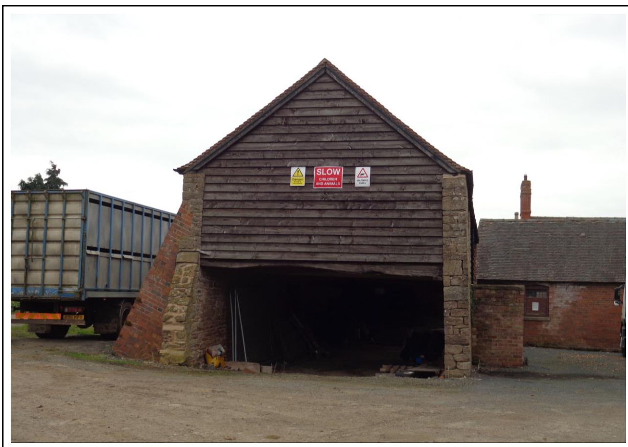
Plate 60: MSA 15495, 26541, agricultural building and house. Shot facing southeast.
