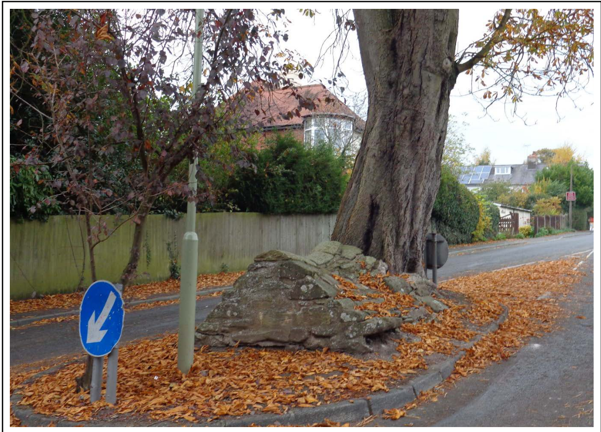
Plate 25: St Julian's Well, details of stone pitched roof. Shot facing north.
