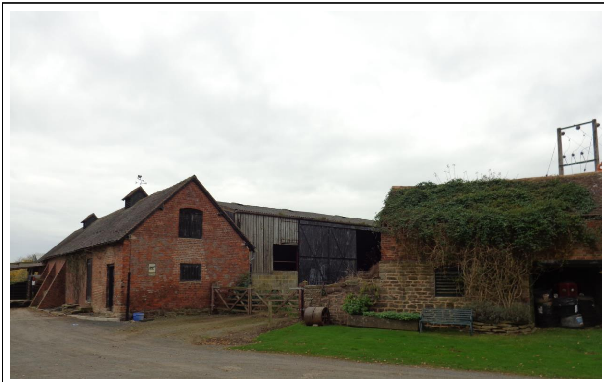
Plate 69: Rock Farm group, MSA 26541, agricultural building. Shot facing west.
