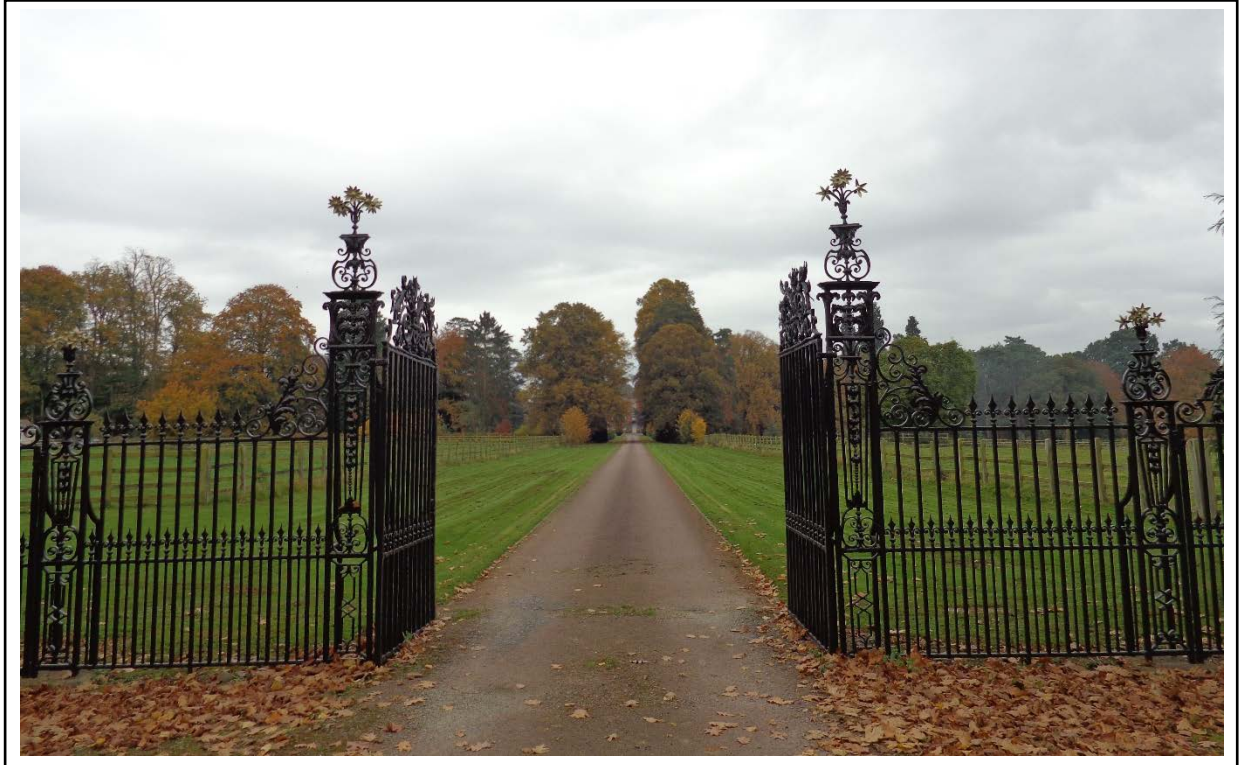
Plate 33: Henley Park entrance, with Henley Hall at the background. Shot facing south
