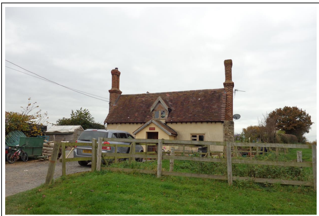
Plate 72: Dodmore Cottage MSA 15780, oblique view. Shot facing west.
