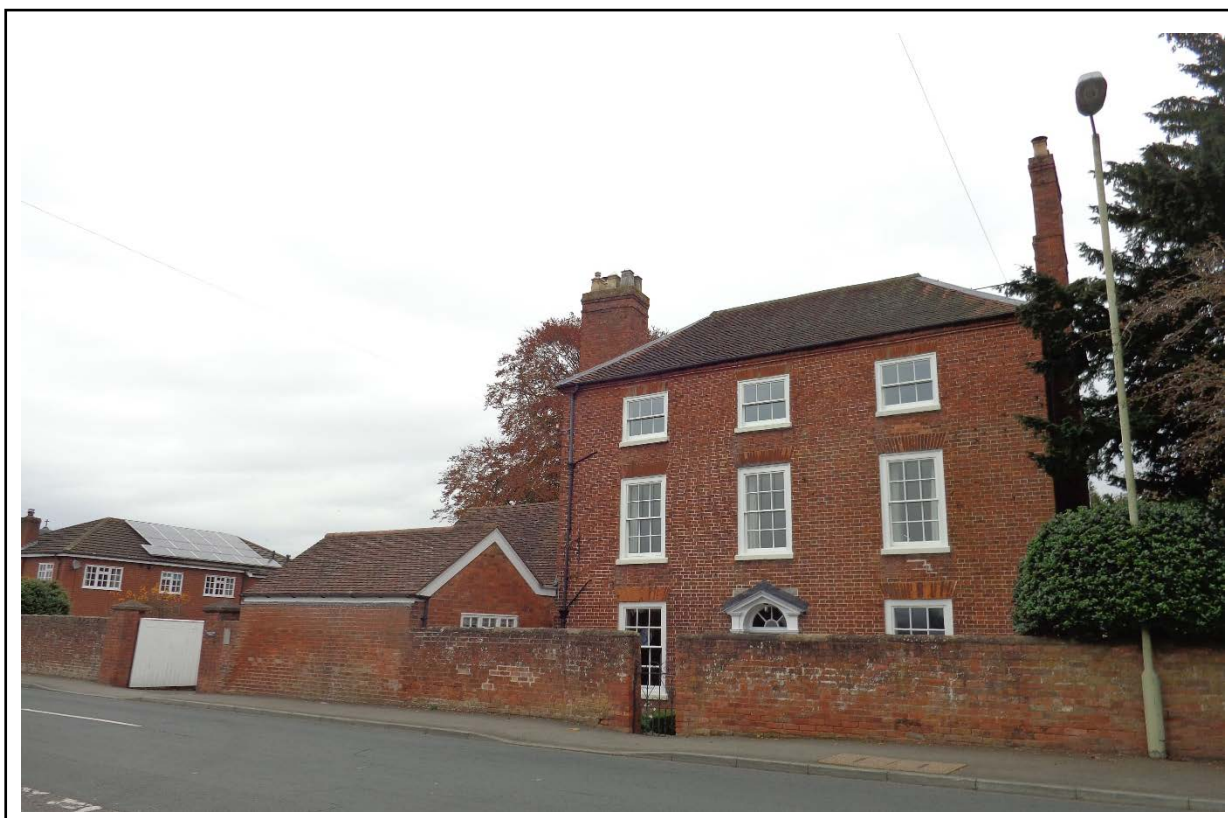
Plate 30: Gravel Hill House, frontal view. Shot facing northeast.
