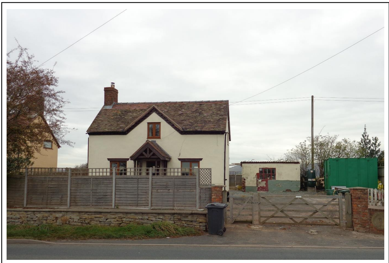
Plate 56: MSA 15491 Suncrest, traditional house. Shot facing northwest.
