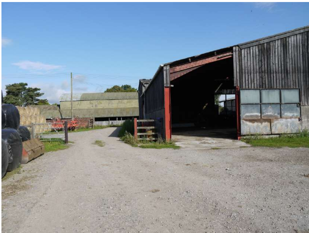
Plate 2: Site looking north.
