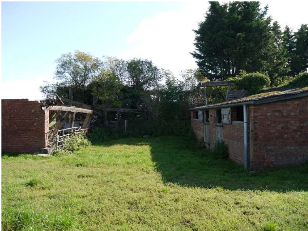
Plate 16: Barn (centre) and adjoining buildings, stables (right) looking east.
