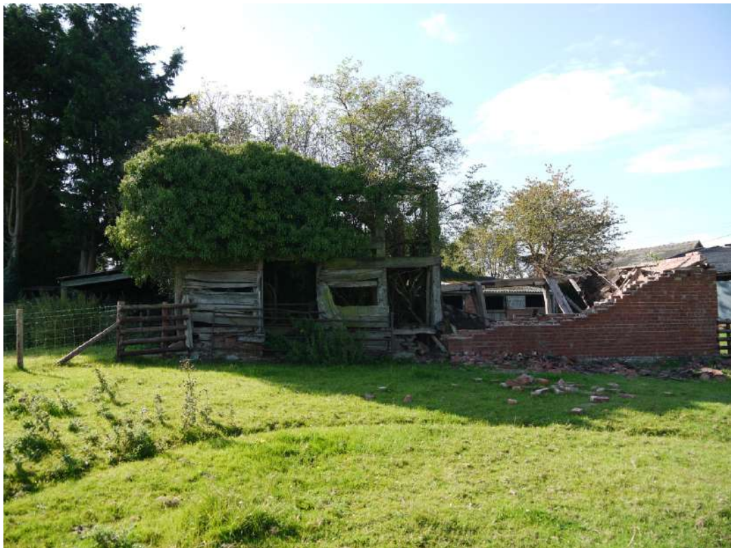
Plate 14: 15 th century timber frame of barn (LB 1383792 / HER 17368); shot facing south.
