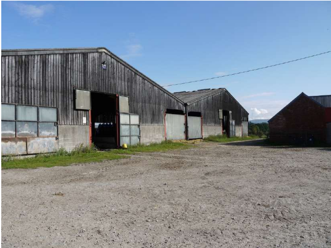
Plate 3: Modern barns on site, shot facing northeast.
