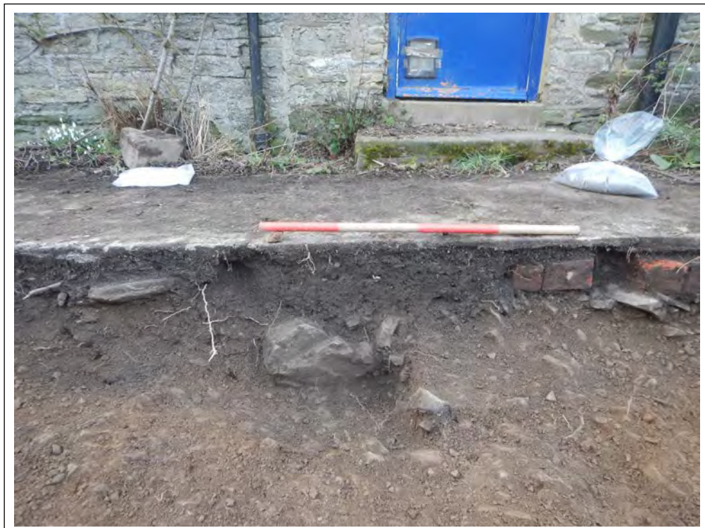
Plate 8. View of widening of foundation trench which runs parallel with the western side of the evaluation trench, looking west. Scale 1m
