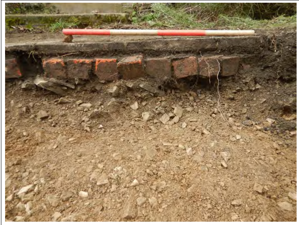
Plate 5. View of brick underpinning (011), looking west. Scale 1m
