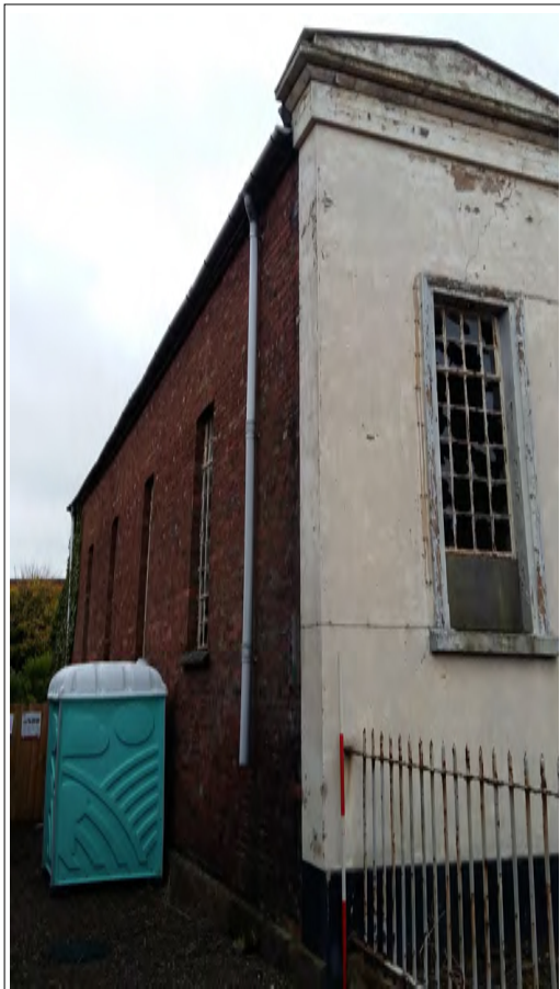
Plate 2. West elevation, looking northwest. Scale 2m
