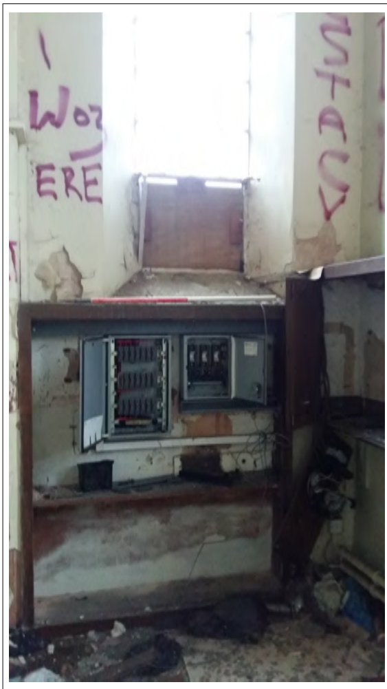
Plate 8. Utility room, looking north. Scale 1m
