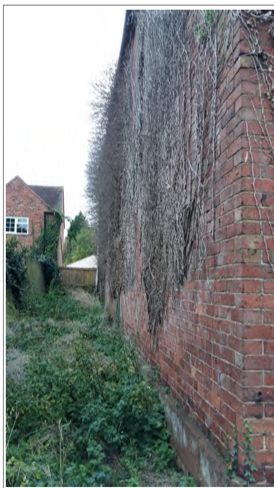
Plate 6. East elevation, looking southeast.
