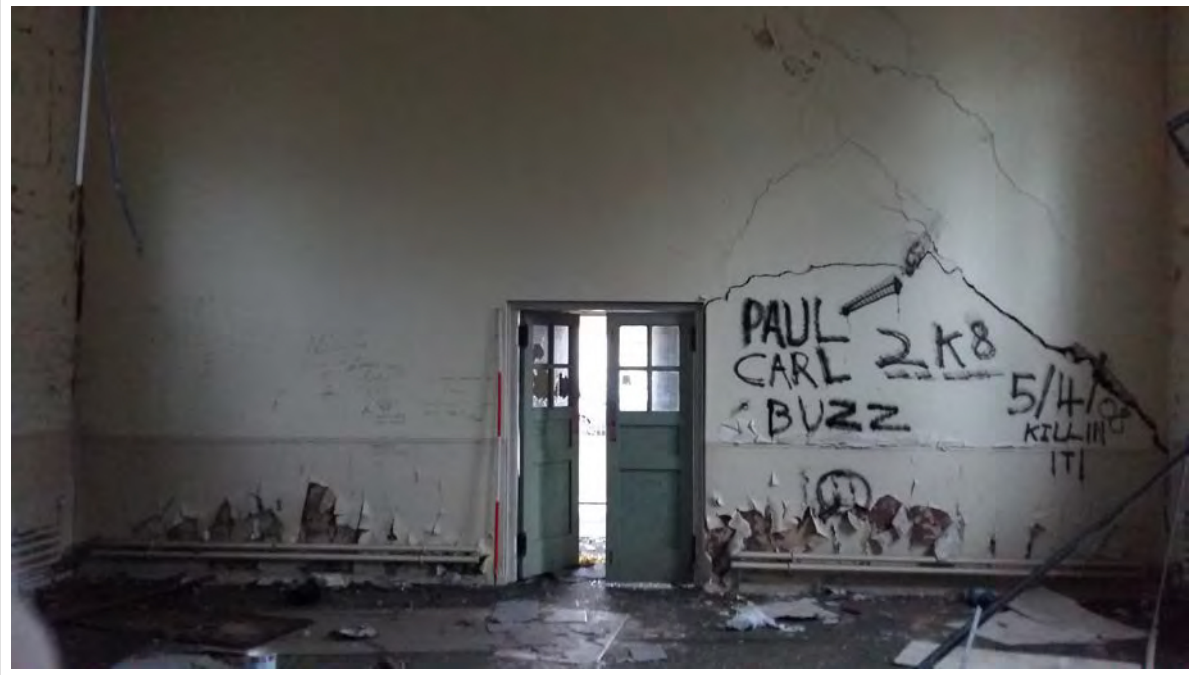
Plate 7. Building interior, north elevation. Scale 2m
