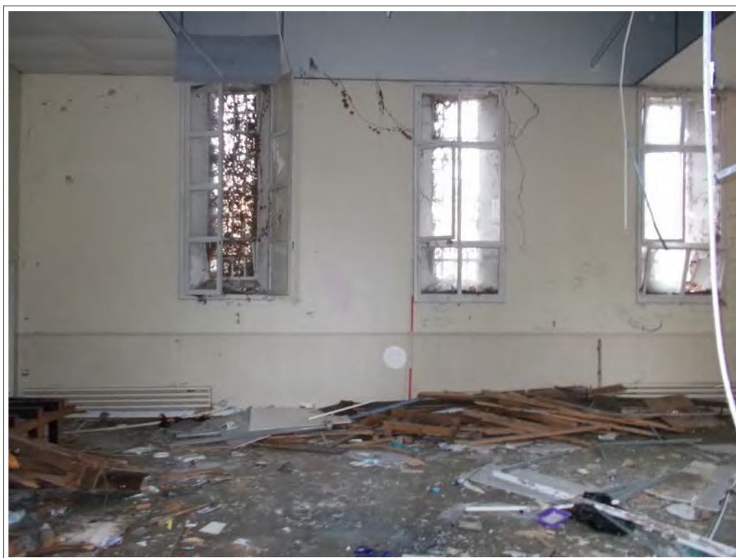
Plate 14. Interior, west elevation, looking west. Scale 2m
