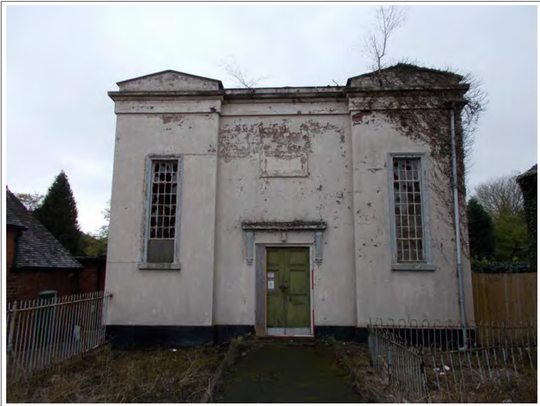
Plate 1. Front elevation Old Baptist Chapel, looking south. Scale 2m
