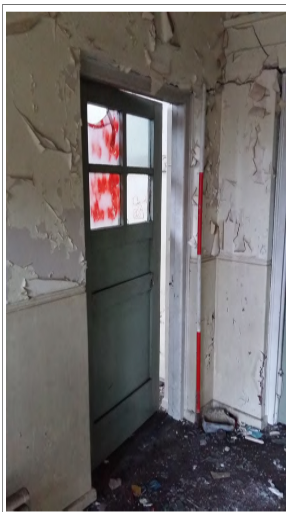
Plate 16. Bathroom door, looking west. Scale 2m
