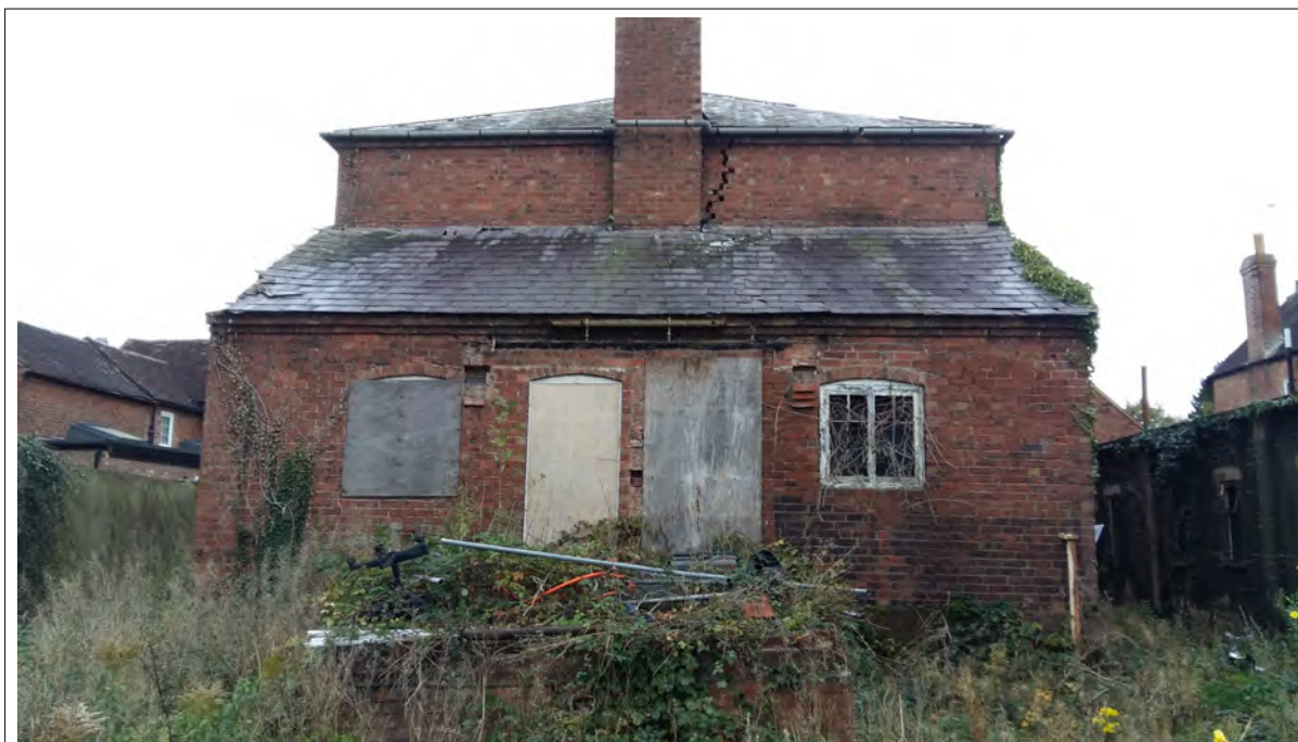
Plate 5. South elevation, looking north.
