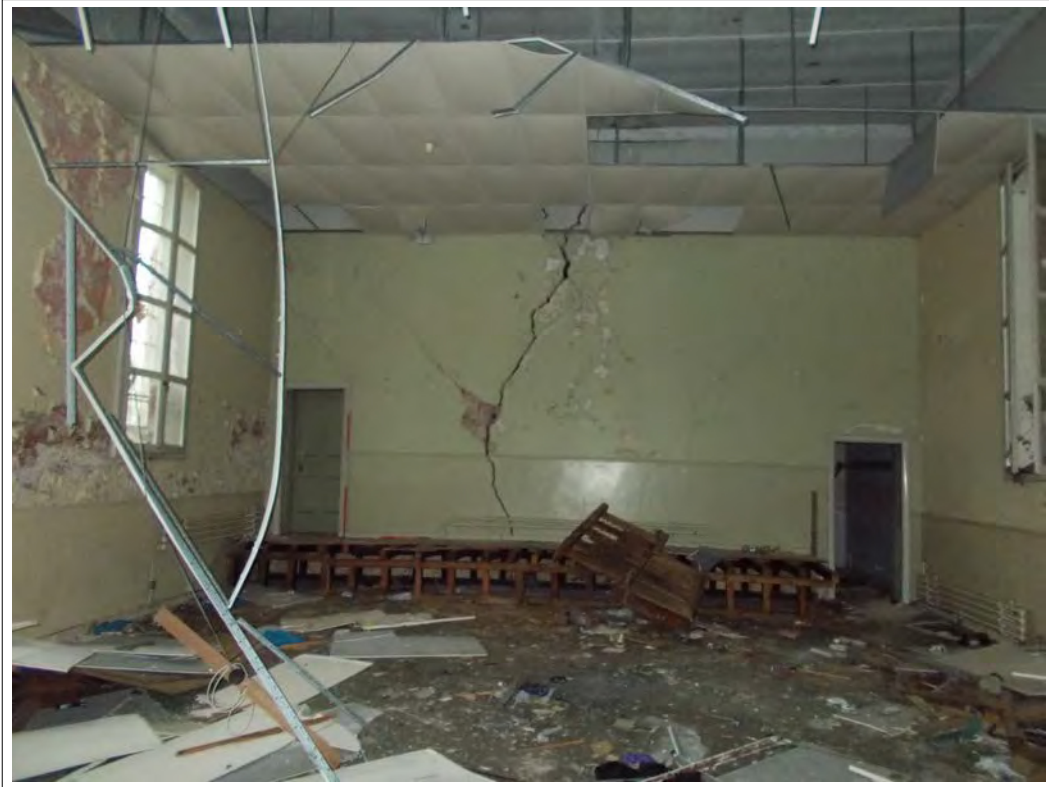
Plate 11. Interior, south elevation. Scale 2m
