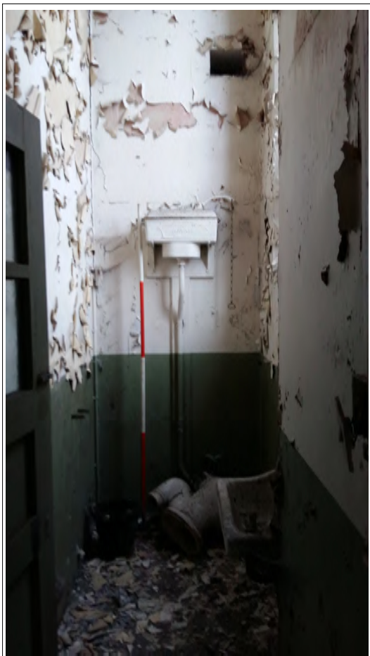
Plate 13. Bathroom area, looking west. Scale 2m
