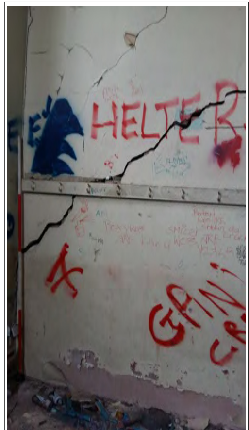
Plate 10. Utility room, looking south. Scale 2m
