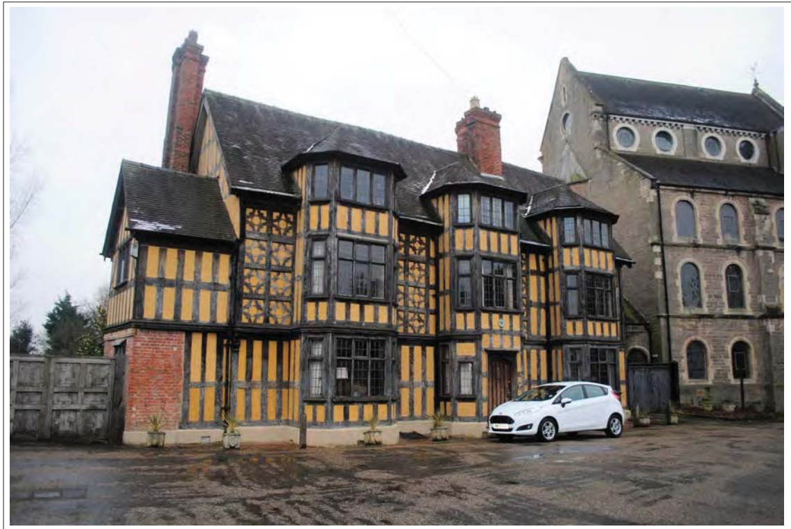
Plate 13. Castle Gates House (LB 1246555) at the main entrance to the castle. Looking southeast.
