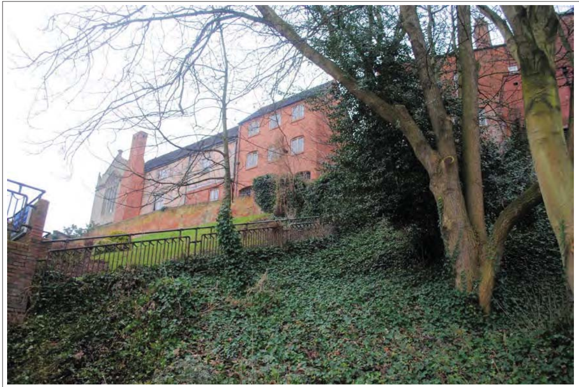
Plate 17. West elevations of the Library (LBs 1271155 & 1271288) and Riggs Hall (LB 1246750). Looking east.
