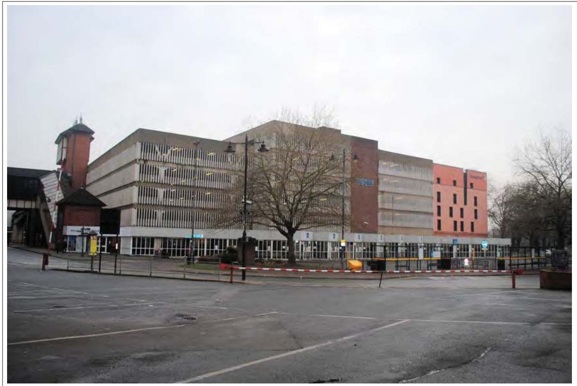
Plate 25. View of Raven Meadows Multi-storey Car Park from the site. Looking west.
