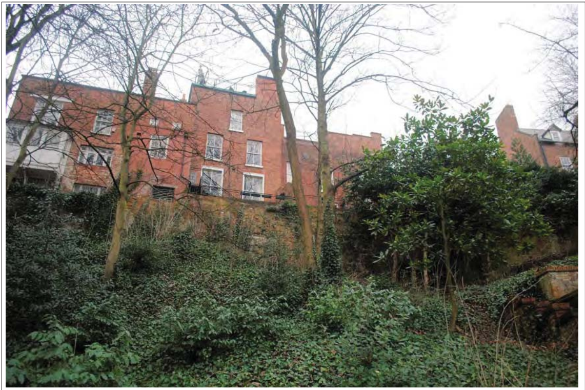
Plate 18. West elevations of the Old School House (LBs 1254868 & 1254870). Looking southeast.
