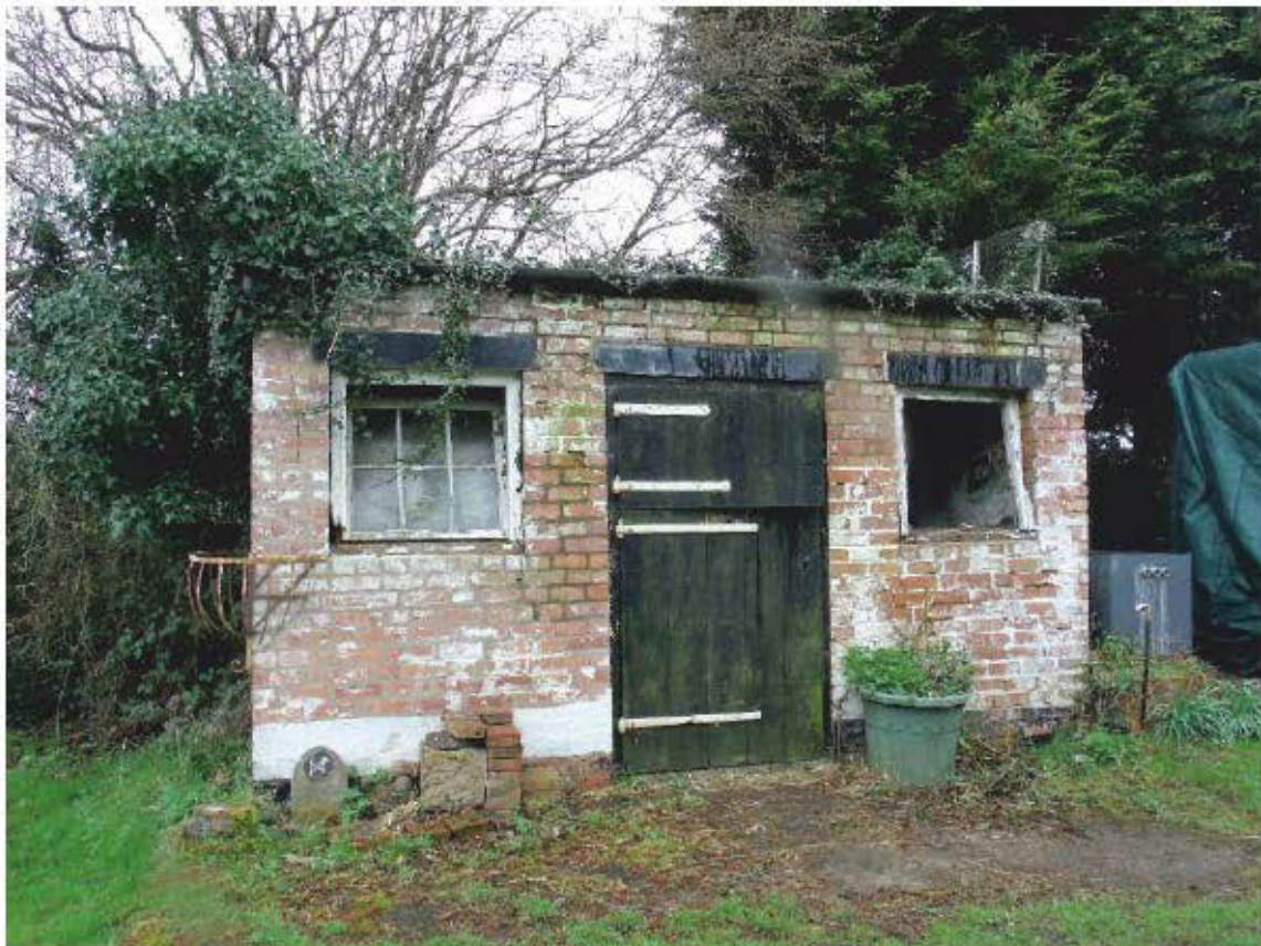
Plate 8: View of old stables at Spring Cottage; shot facing W
