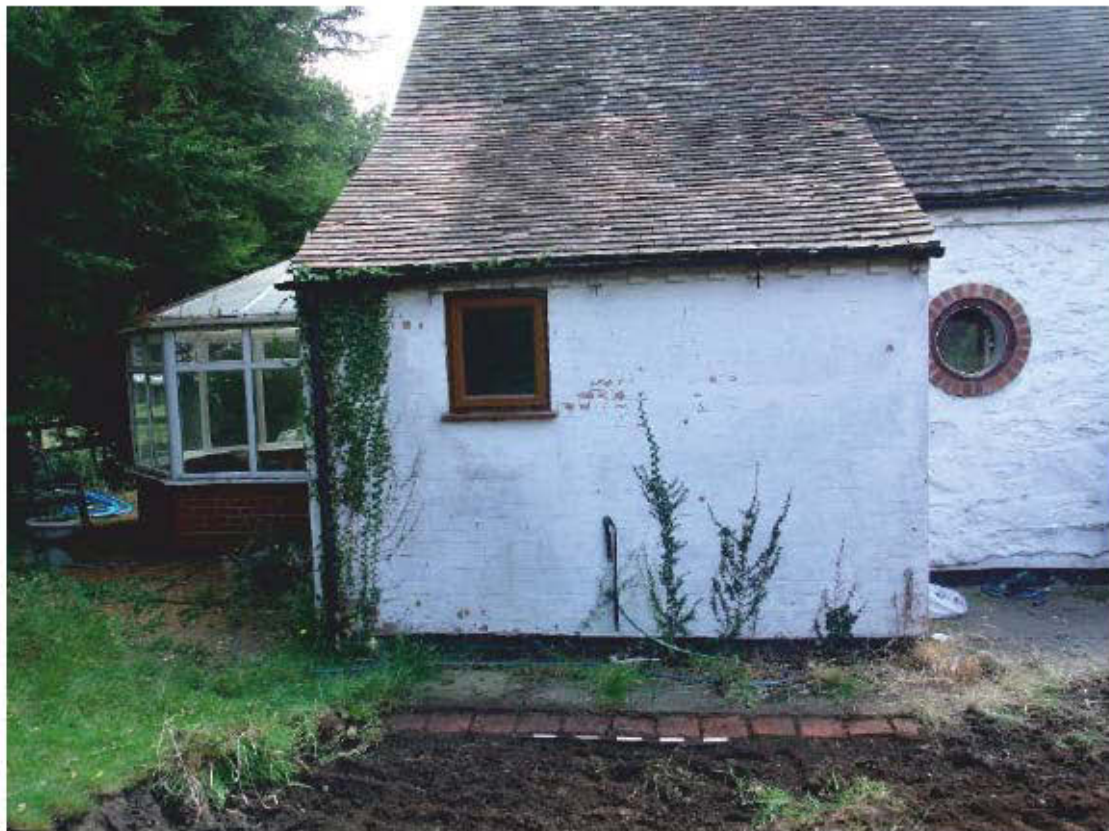
Plate 20: View of alignment of reused ceramic tiles [206], in Trench 2 at the rear of the house; shot facing SE
