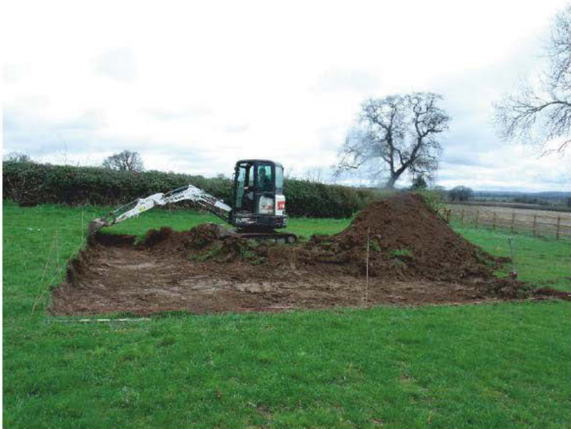
Plate 11: View of works at Trench 1, for new stables; shot facing NW
