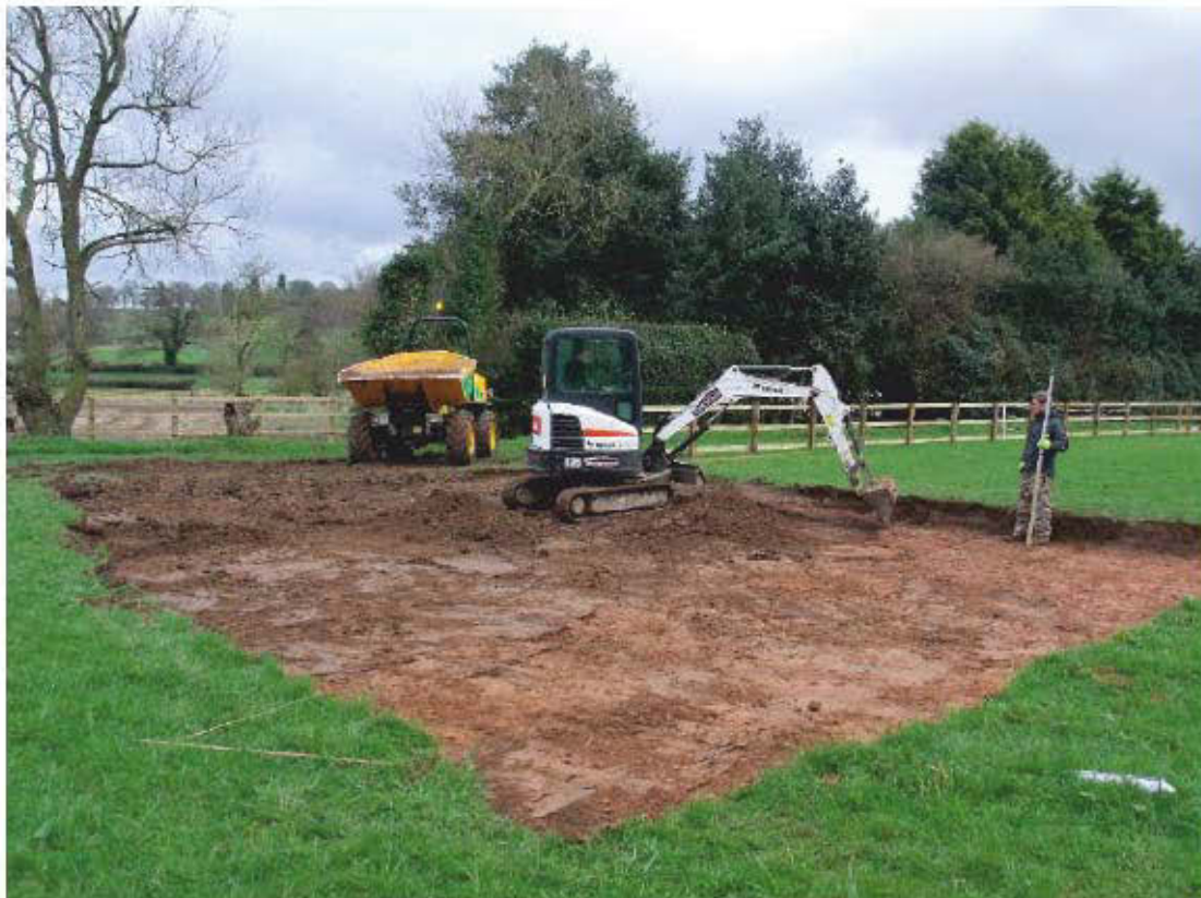
Plate 12: View of works at Trench 1, for new stables; shot facing E
