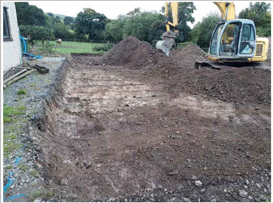
Plate 11. Eastern end of excavations. View S.
