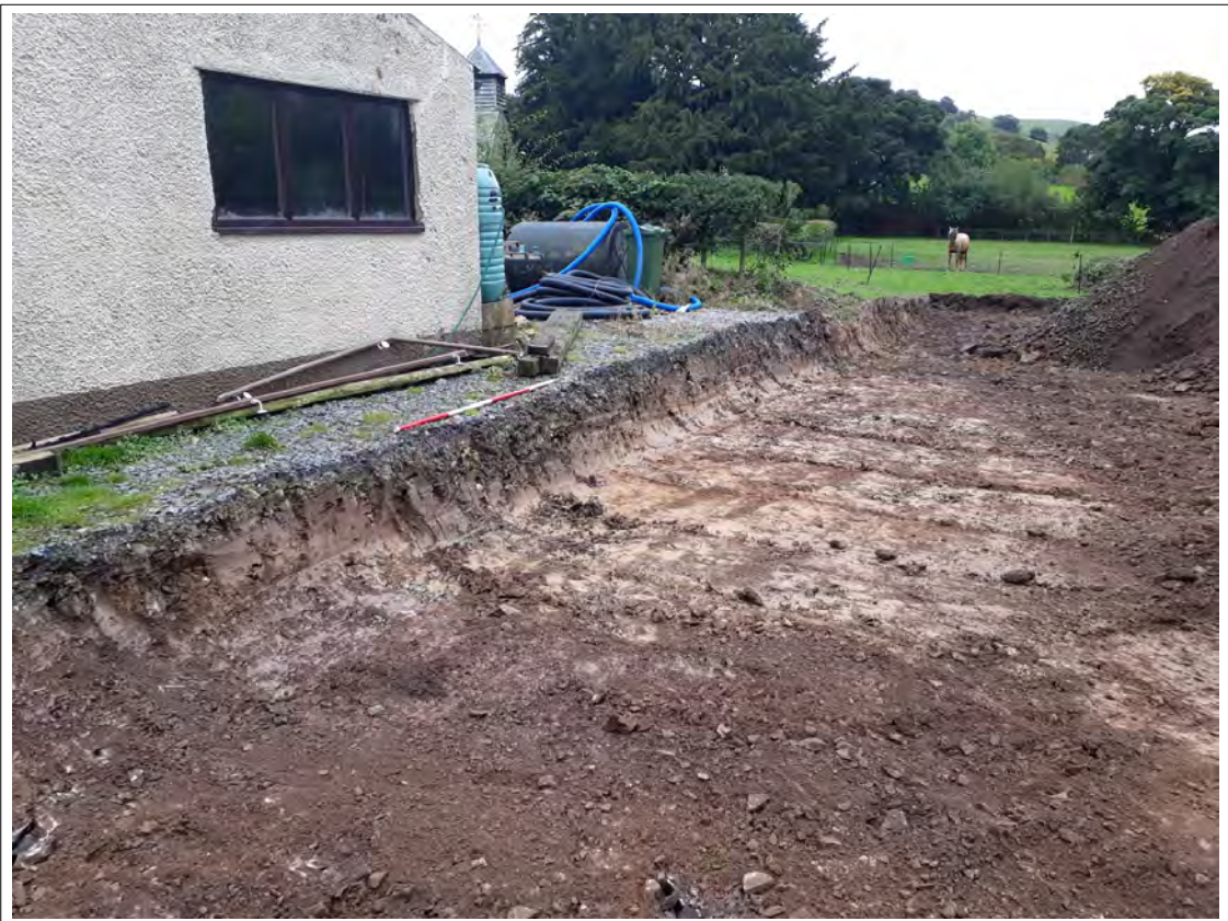
Plate 8. Eastern end of excavations showing natural clay. View S. 2m scale
