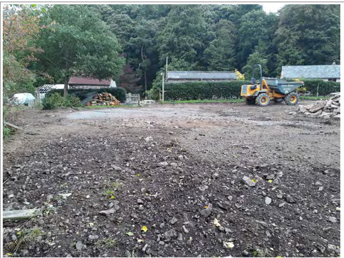
Plate 16. Western end of excavations, topsoil strip onto mixed made-ground. View N
