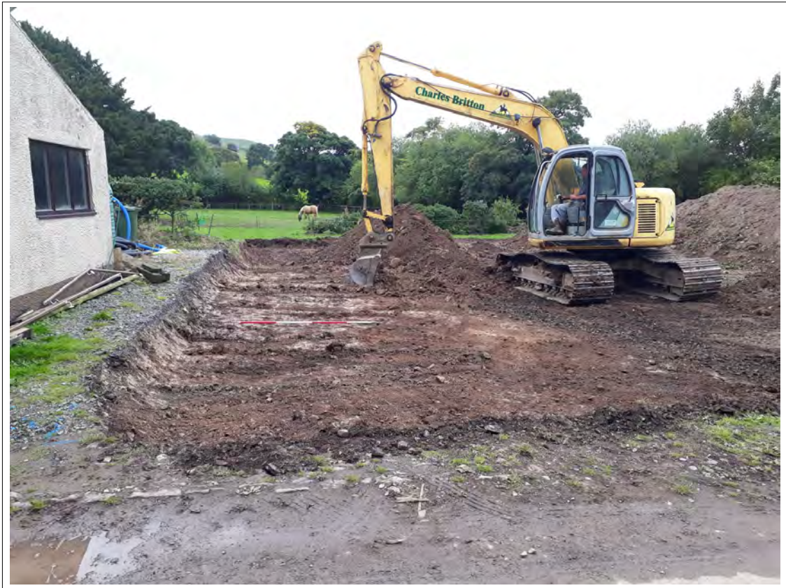
Plate 7. Eastern end of excavations. View S. 2m scale
