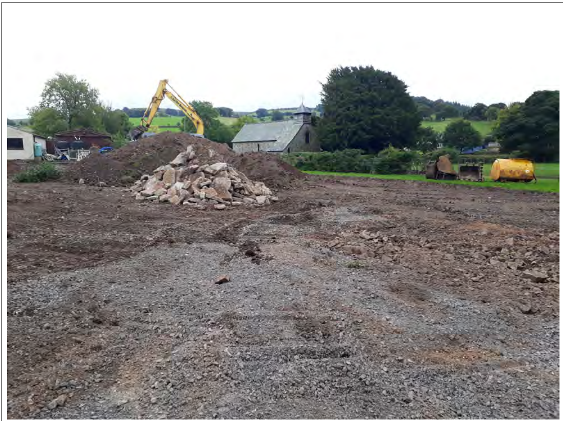
Plate 15. Western end of excavations, topsoil strip onto mixed made-ground. View SE
