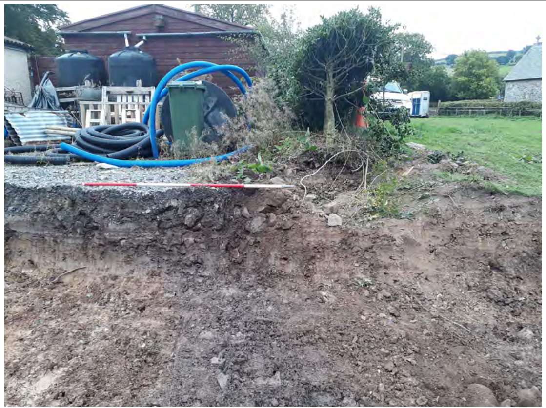
Plate 9. Eastern end of excavations, section of bank with holly hedge. View E. 2m scale
