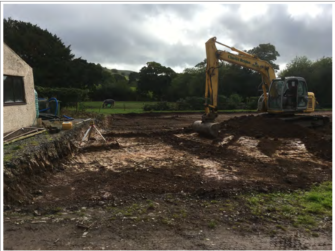
Plate 14. Eastern end of excavations. View S.
