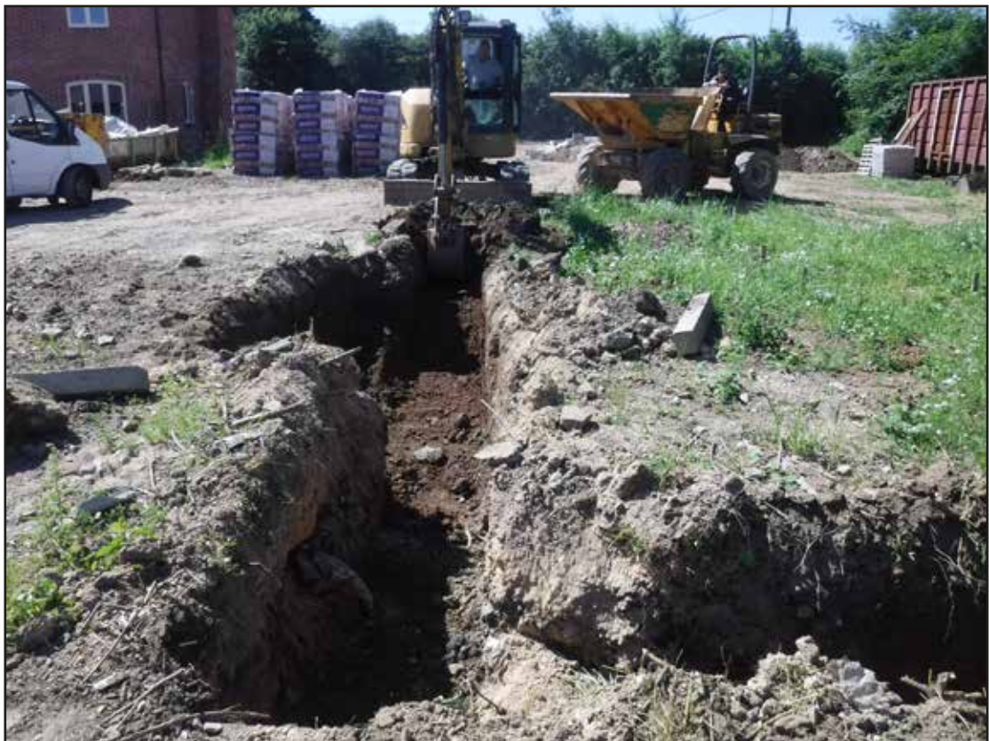
Plate 11. Plot 2, working shot, looking SSE.
