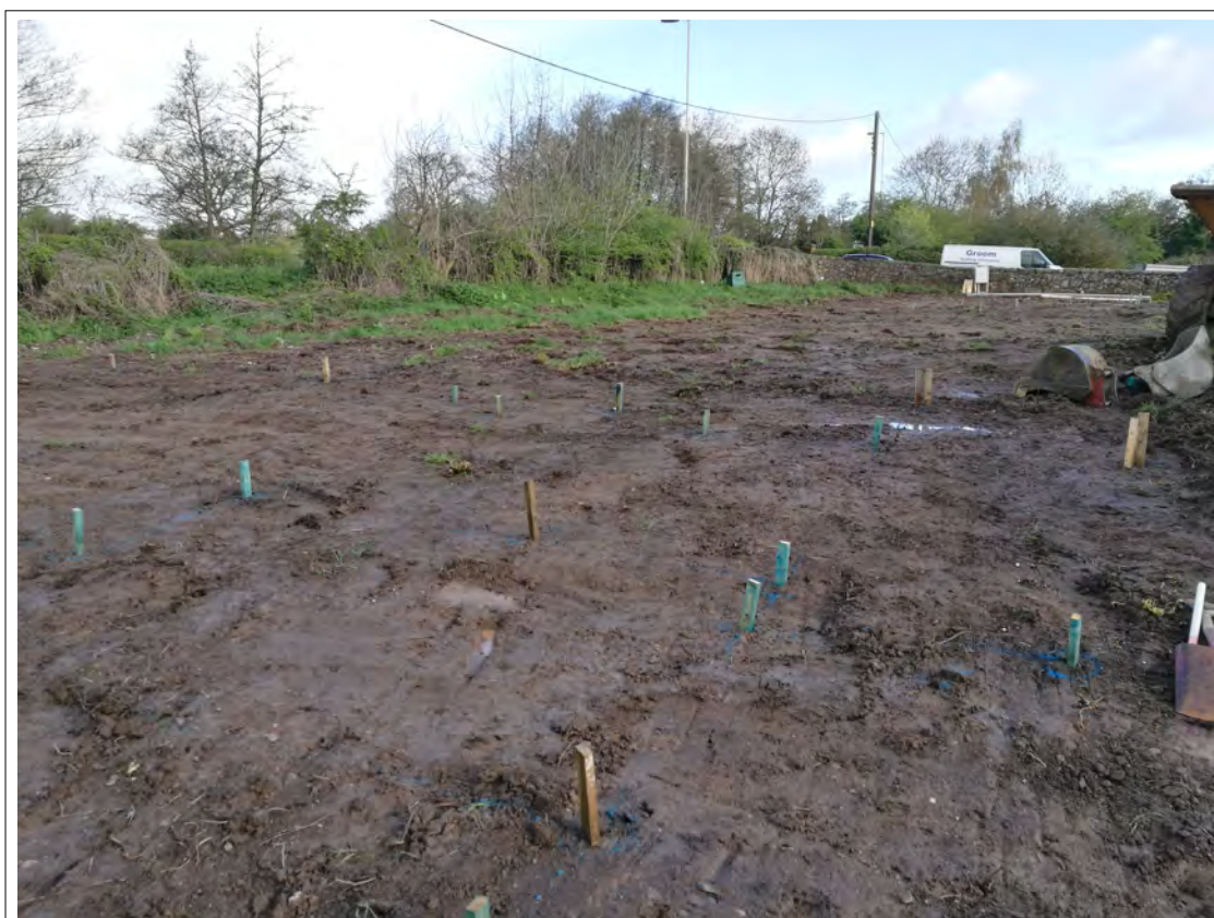
Plate 2. The site prior to excavation. View NW
