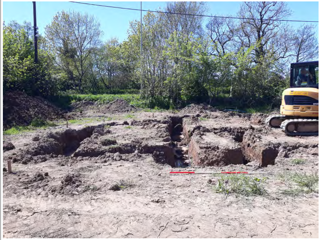
Plate 9. Excavated footings. View W. 2m scale. Plot 1
