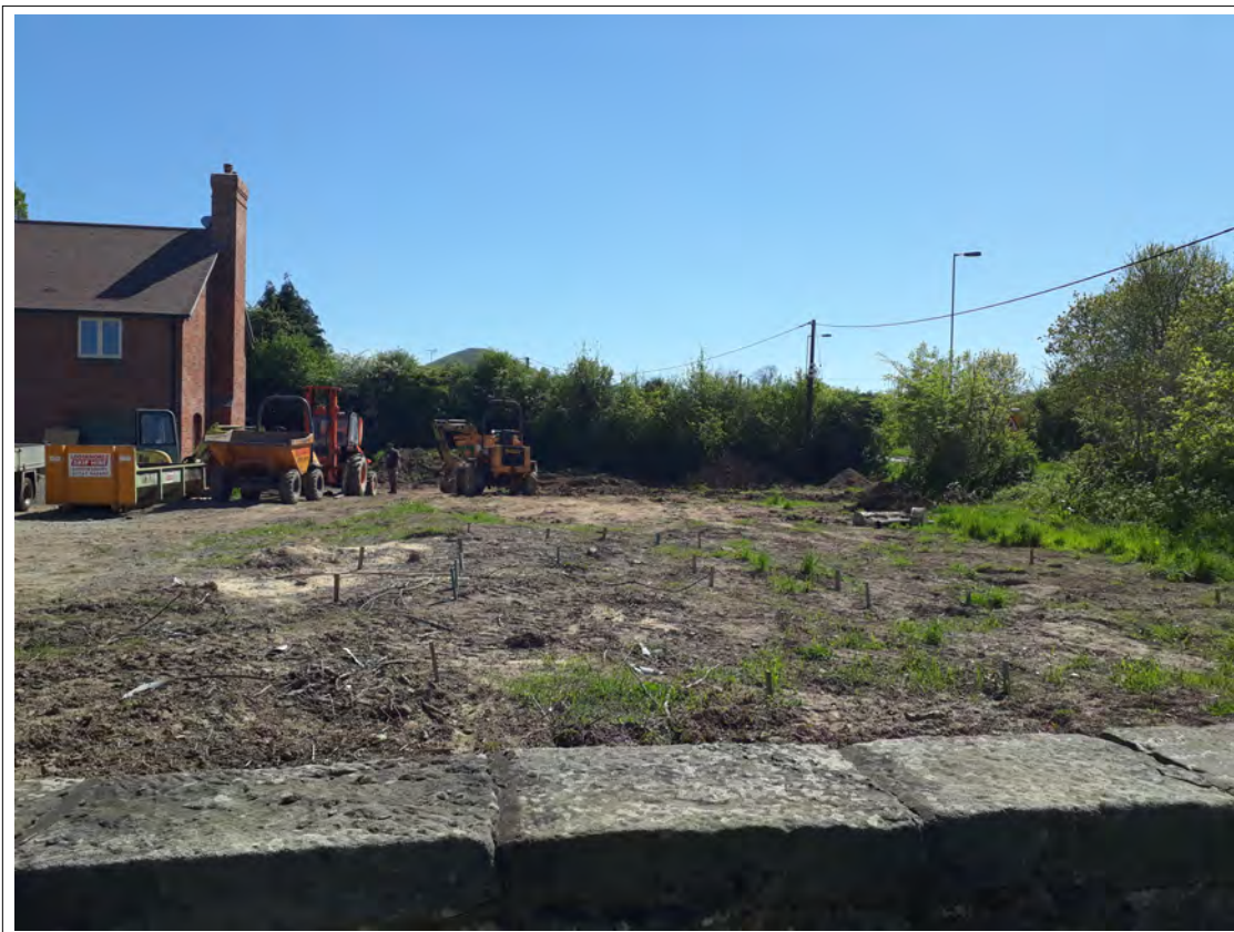
Plate 1. Plot 1 prior excavation. View S
