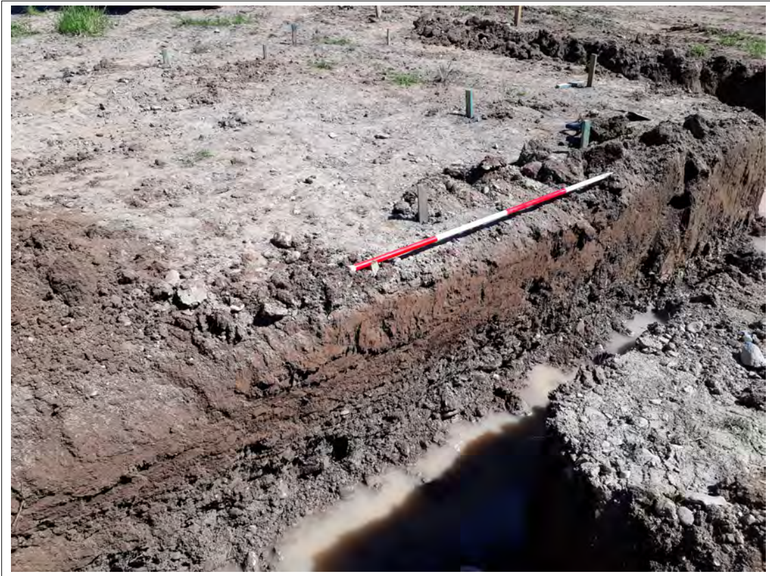
Plate 7. Excavation of footings. View NE. 2m scale. Plot 1
