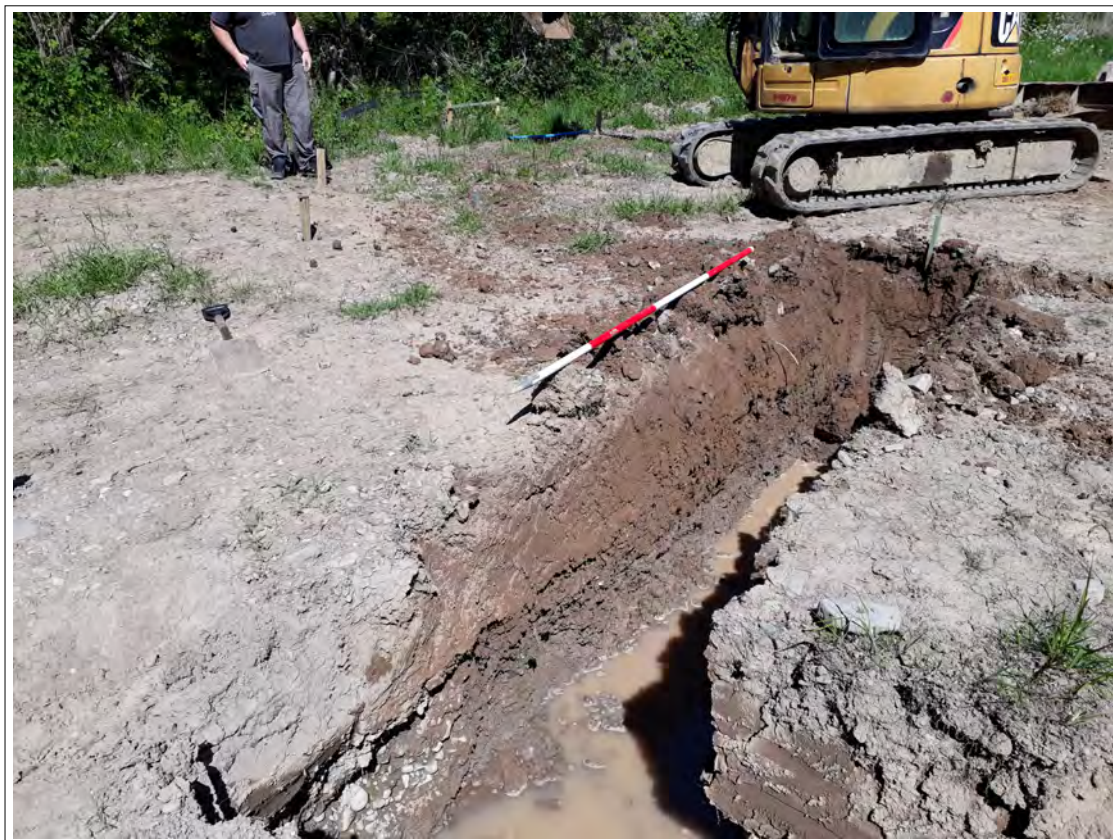
Plate 6. Excavation of footings. View NW. 2m scale. Plot 1
