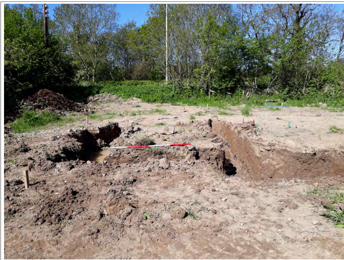
Plate 3. Excavation of footings. View W. 2m scale - Plot 1.
