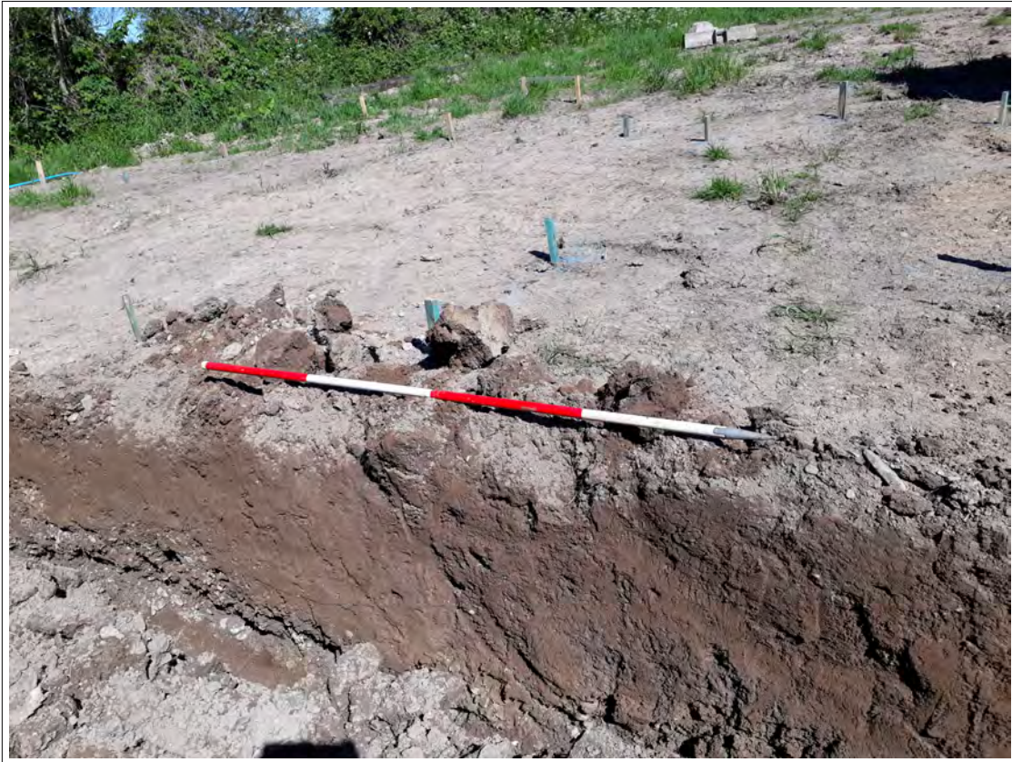
Plate 5. Excavation of footings. View NW. 2m scale. Plot 1
