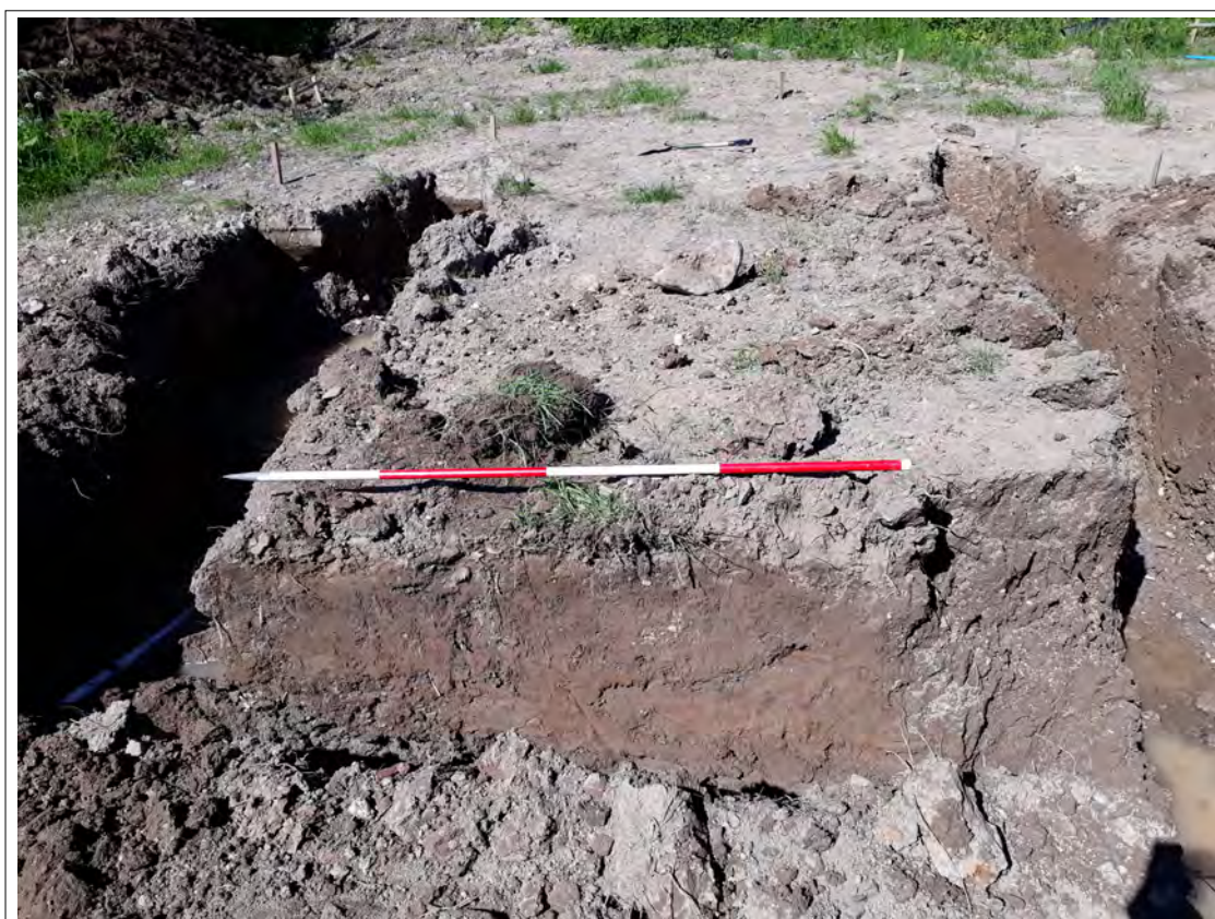
Plate 4. Excavation of footings. View W. 2m scale. Plot 1
