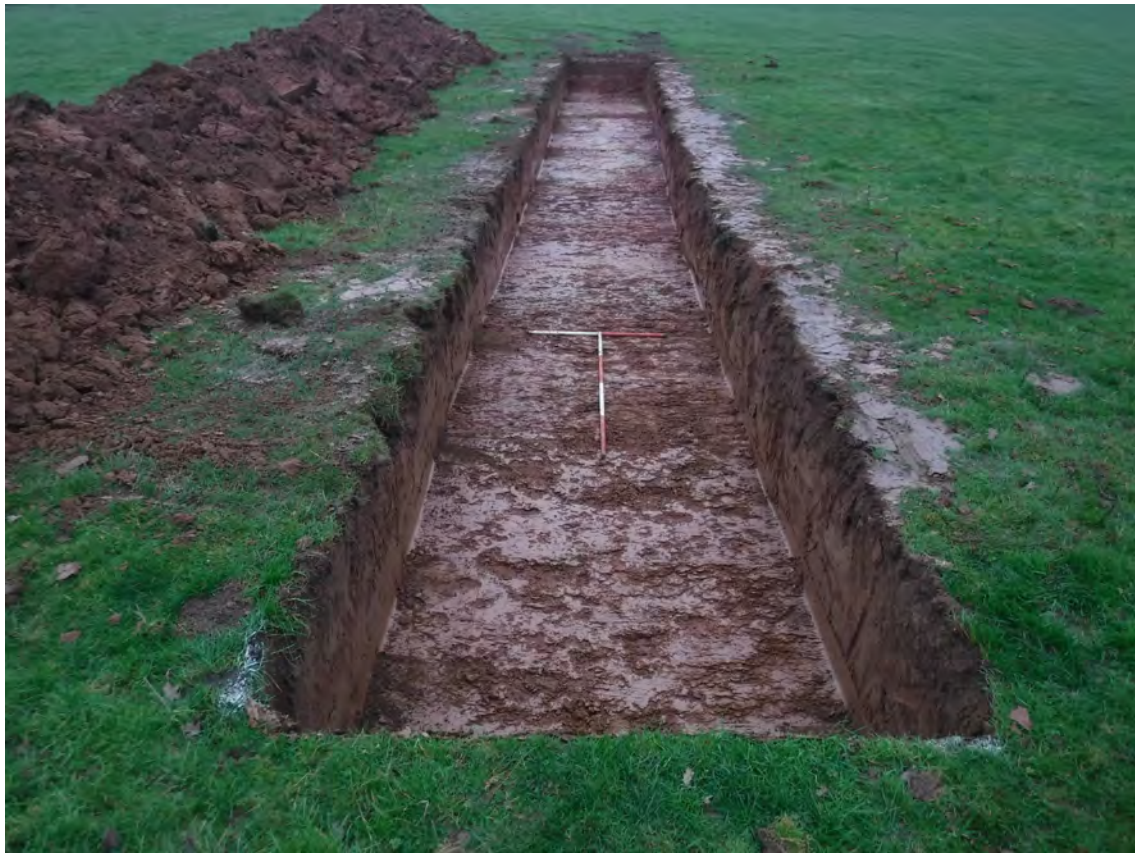
Plate 45. Trench 22, looking east. Scales 1m & 2m
