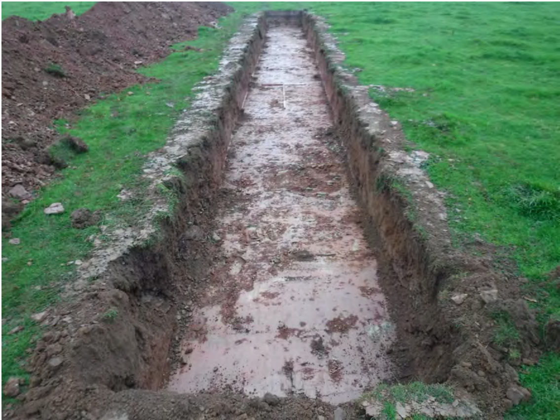
Plate 3. Trench 2, looking east. Scales 1m & 2m
