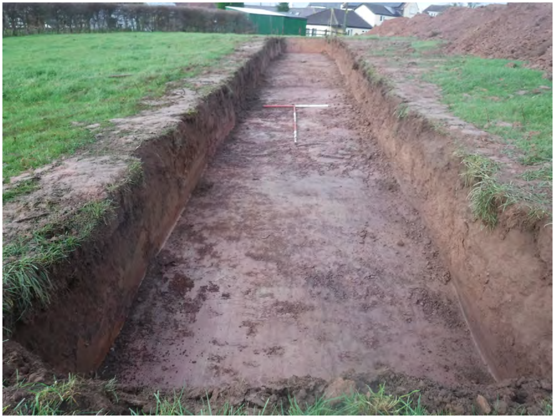
Plate 55. Trench 27, looking north. Scales 1m & 2m
