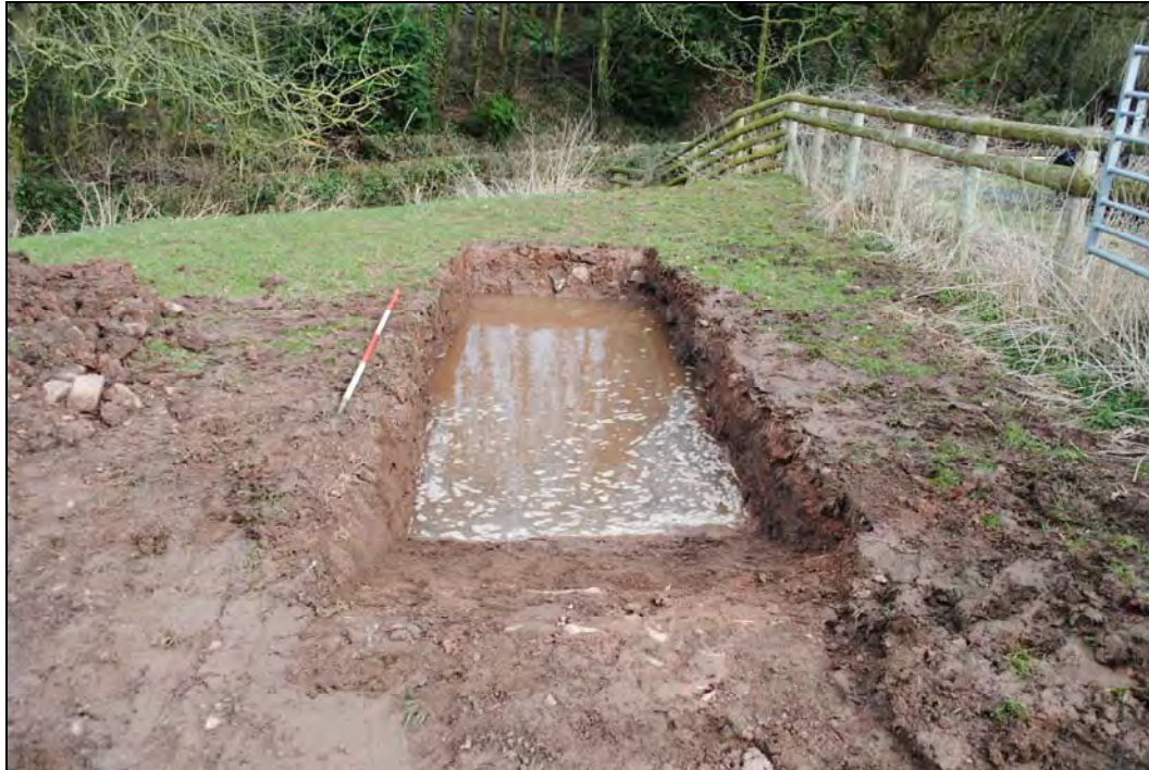
Plate 13. Trench 3. Looking north.
