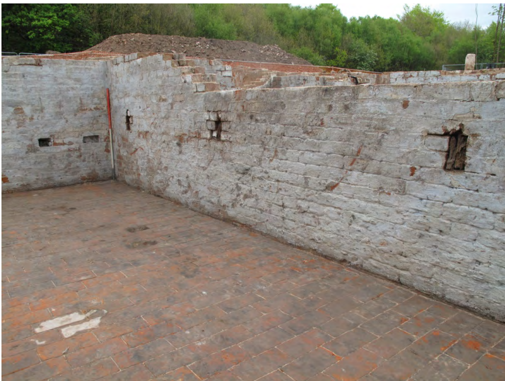
Figure 22: The remains of three voids containing timber remains within the eastern wall (070) within Room B5.
