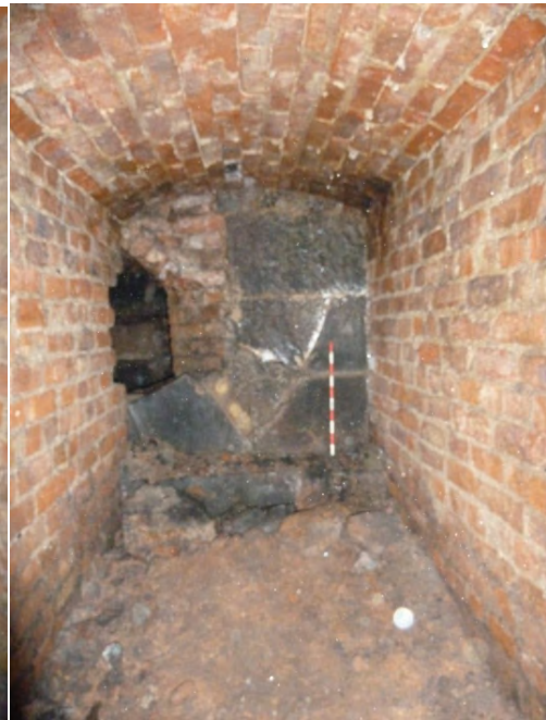
Figure 98: southern wall of Room C13. Looking south.
