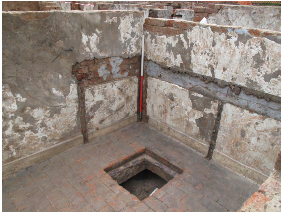
Figure 52: north-west quadrant of Room B12, sub-basement access hatch (252)
