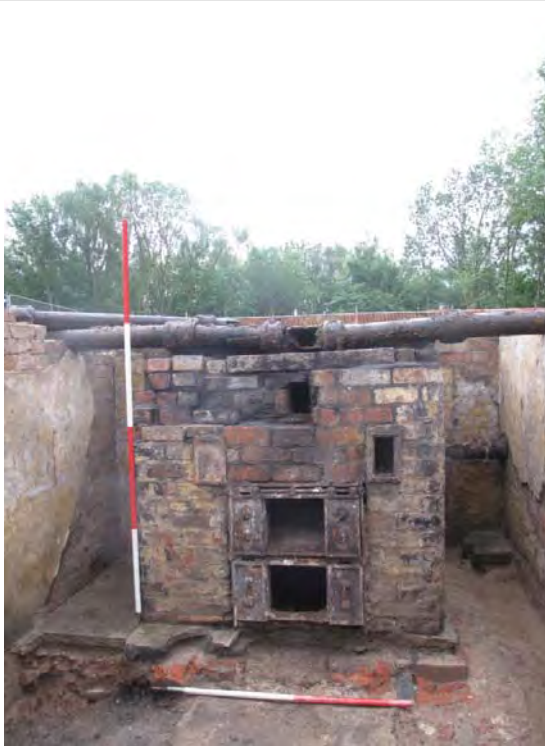
Figure 62: Closeup of Boiler (240 ) Within Room B14.
