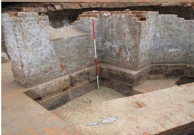
Figure 39: View of south end of B9 western wall (061), showing the walls window sill and plinth (141), looking south-east.
