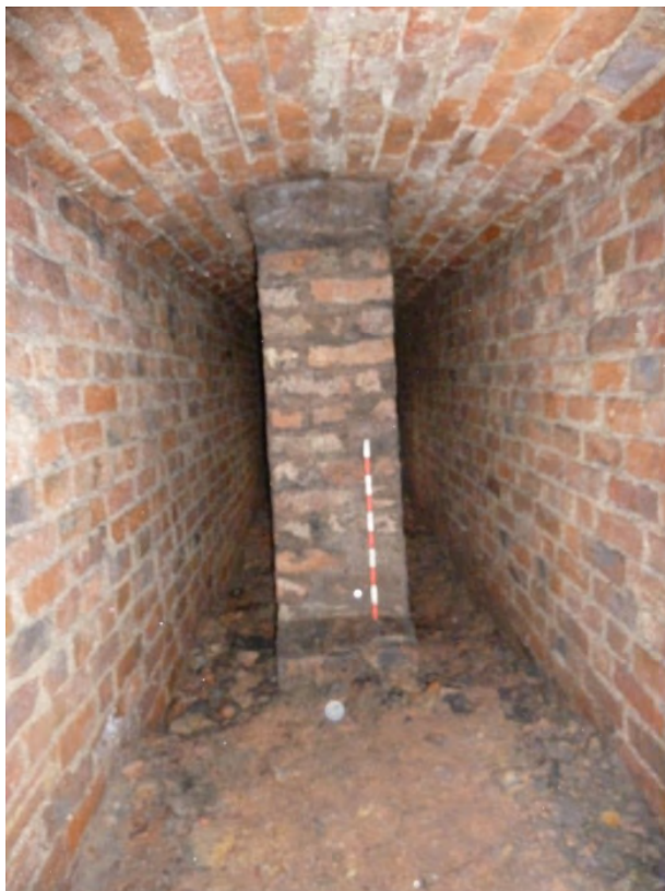
Figure 93: Brick column in Room C10. Looking south.
