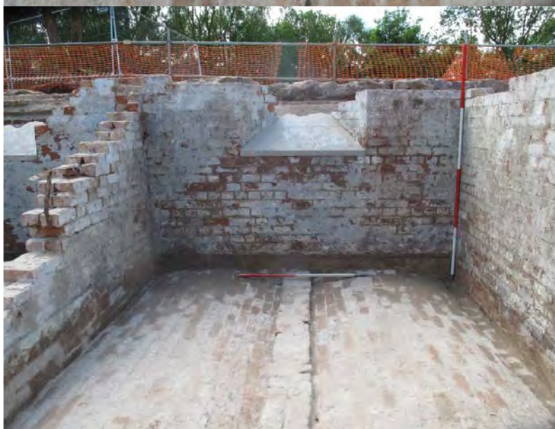
Figure 33: View of window sill in southern wall (004) of B7a, looking south.
