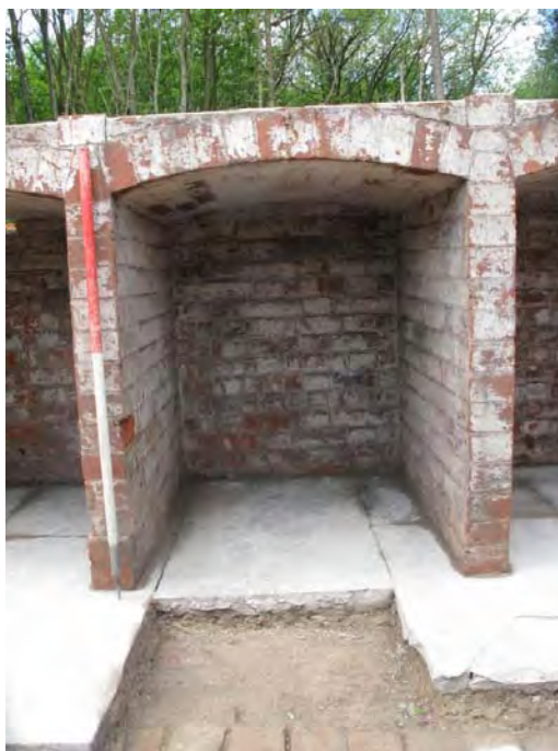
Figure 19: Brick built storage bays (015) within Room B4.
