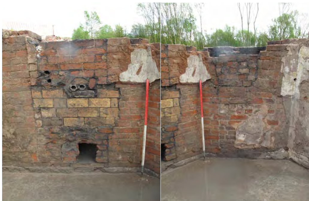
Figure 74: Blocked up doorway Within Room B18.
