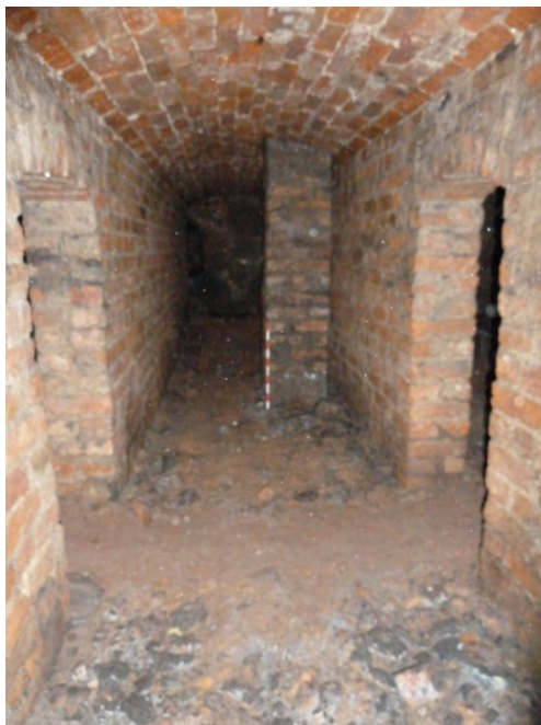
Figure 97: Room C13 with brick column. Looking south.
