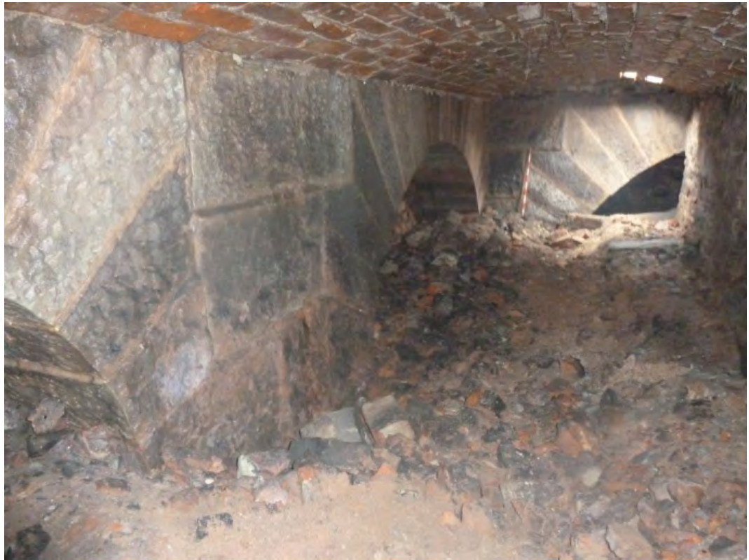
Figure 107: Room C27. Looking northwest.
