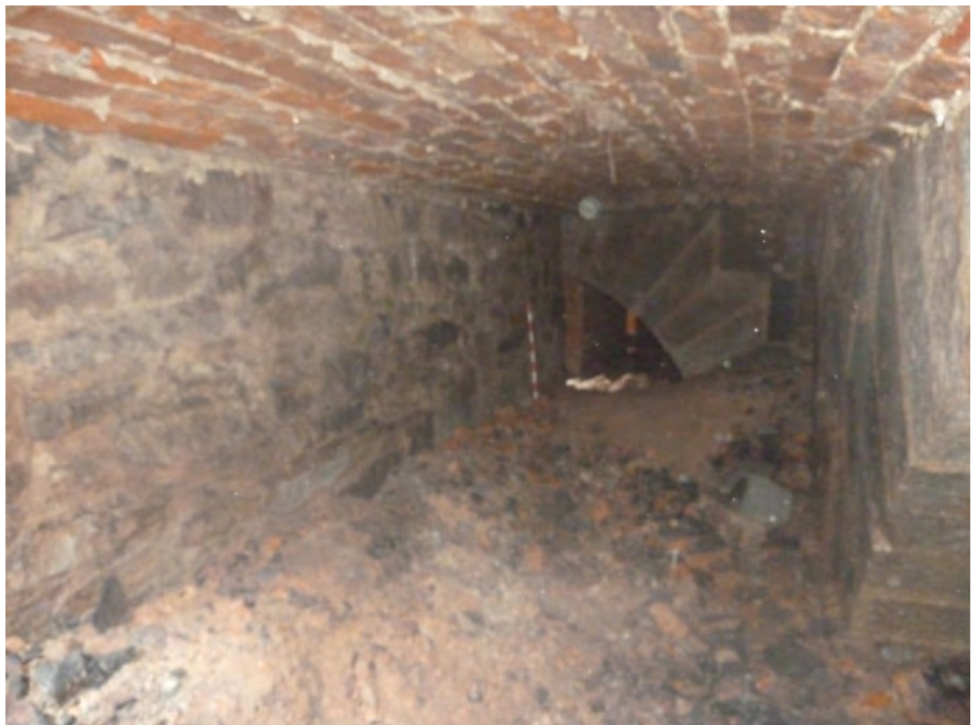
Figure 108: Room C27. Looking south.
