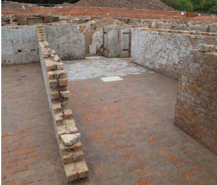
Figure 26: Detail of doorways in the northern (002) and eastern (073) walls of B6, looking north-east.
