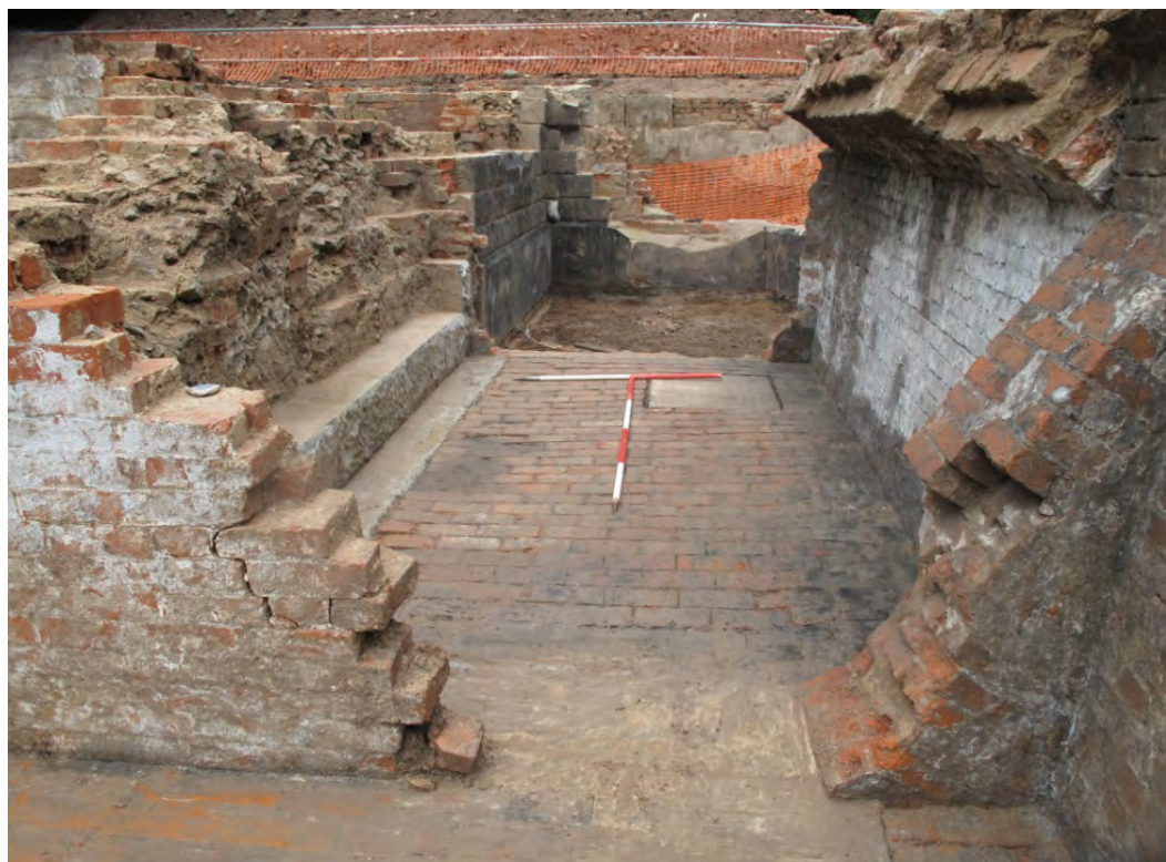
Figure 9: View of north/south wing of Corridor 5, looking north.
