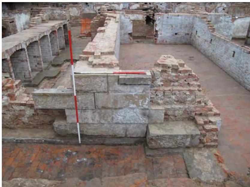
Figure 10: Detail of ashlar facing stones (144) on northern wall (004) of Corridor 6, looking north
