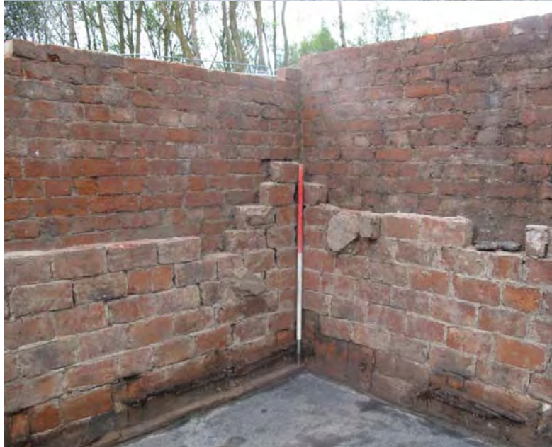
Figure 72: Inserted brick skin (275) on the internal face of Room B16.
