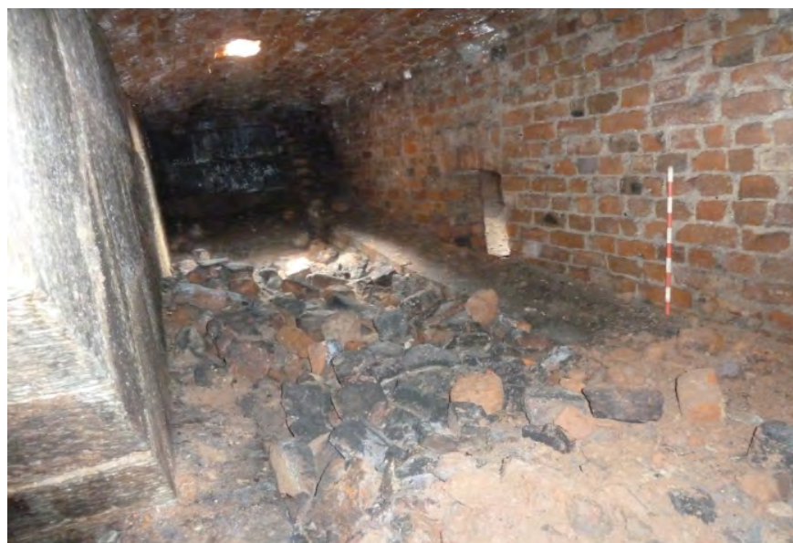
Figure 86: Room C3 Looking southwest
