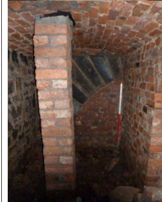
Figure 106: Northern end of Room C26. Looking north.
