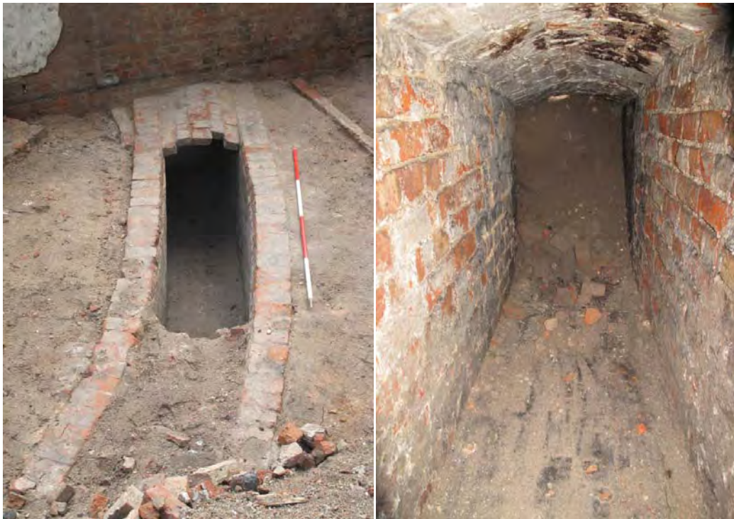
Figure 44: Detail of brick tunnel (166) in B10, looking east.
