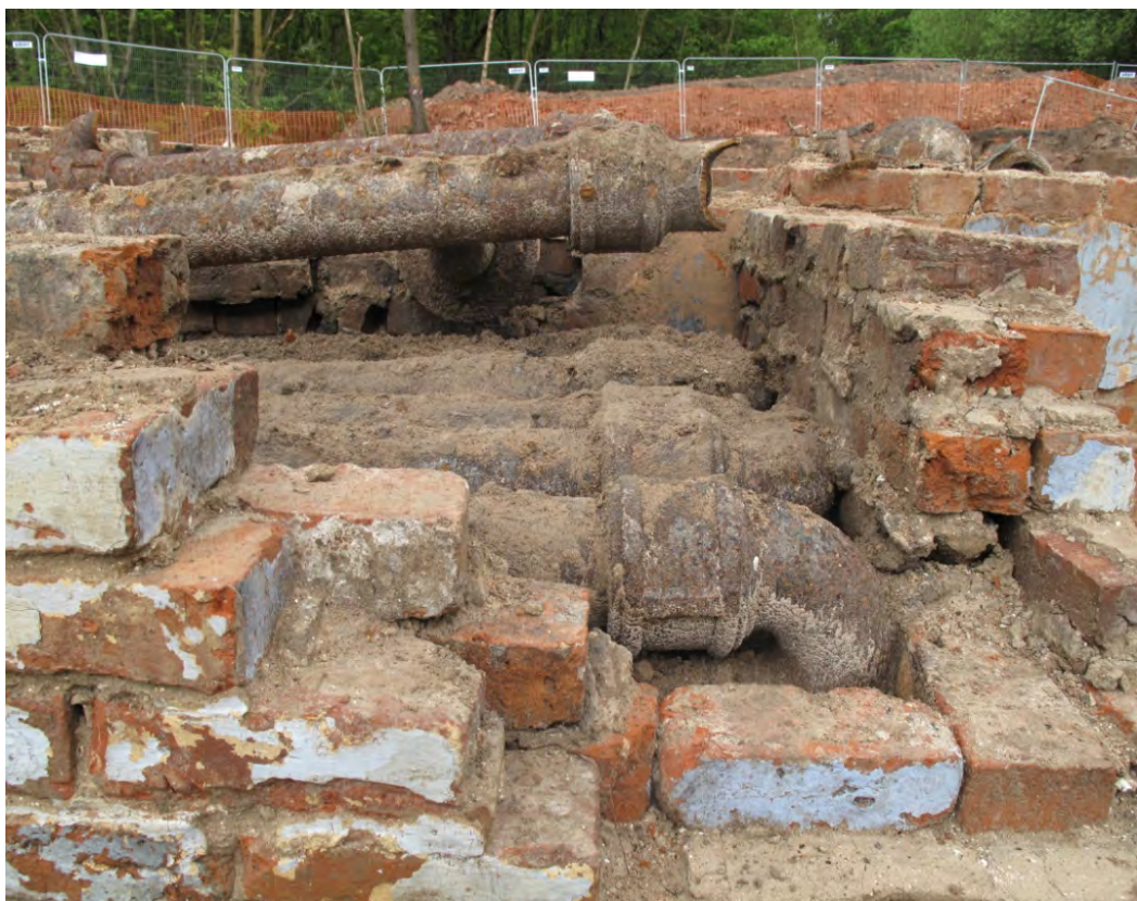
Figure 50: Cast iron pipes within the heat exchanger (231) in Room B12.
