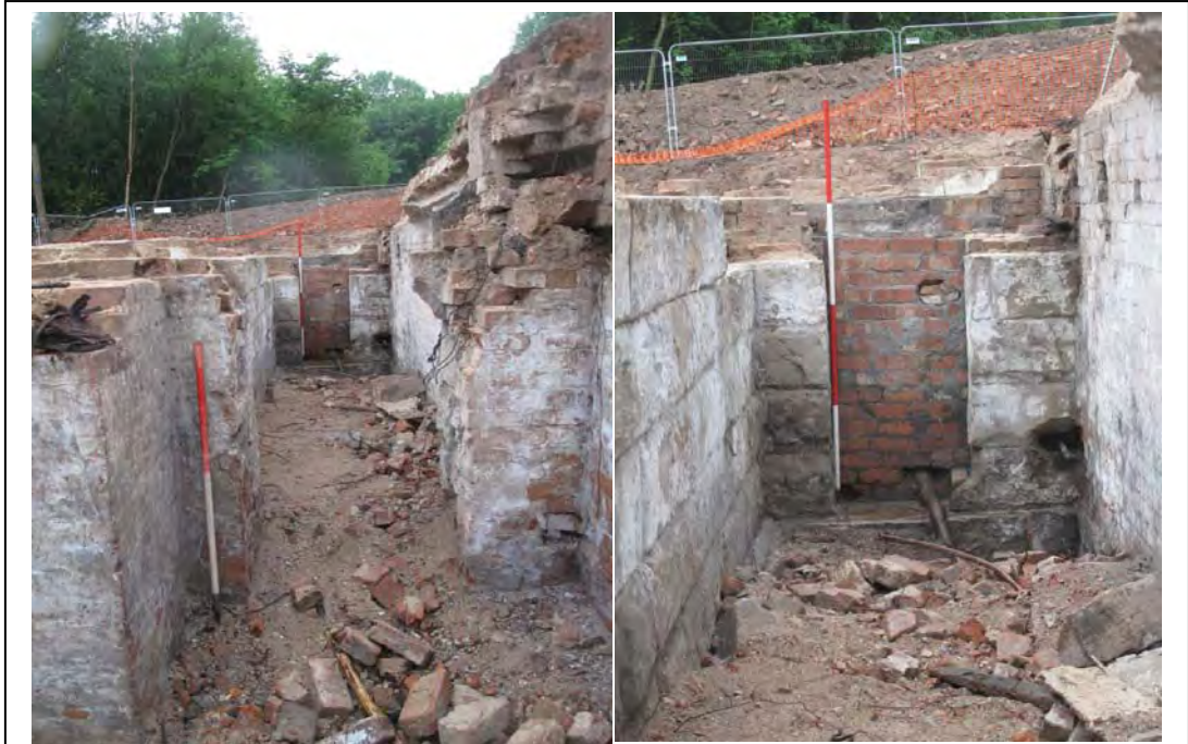
Figure 77: Room B20 looking west.
