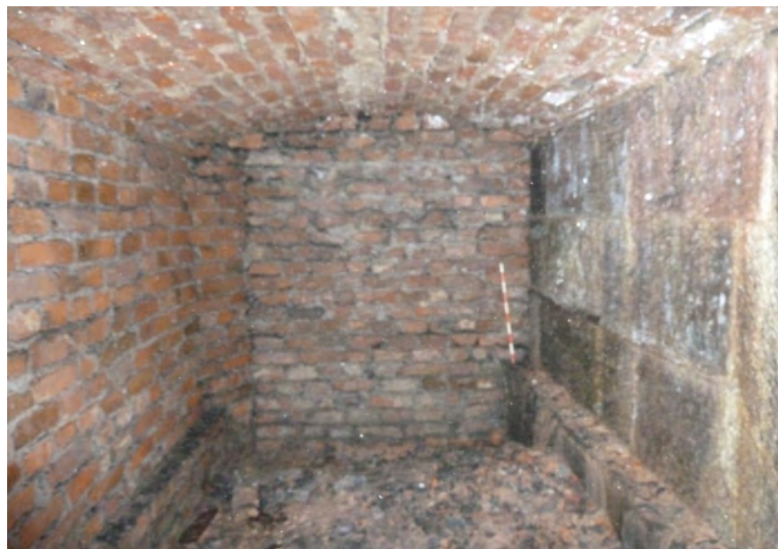
Figure 85: Blocking at southern end of Room C2. Looking south.
