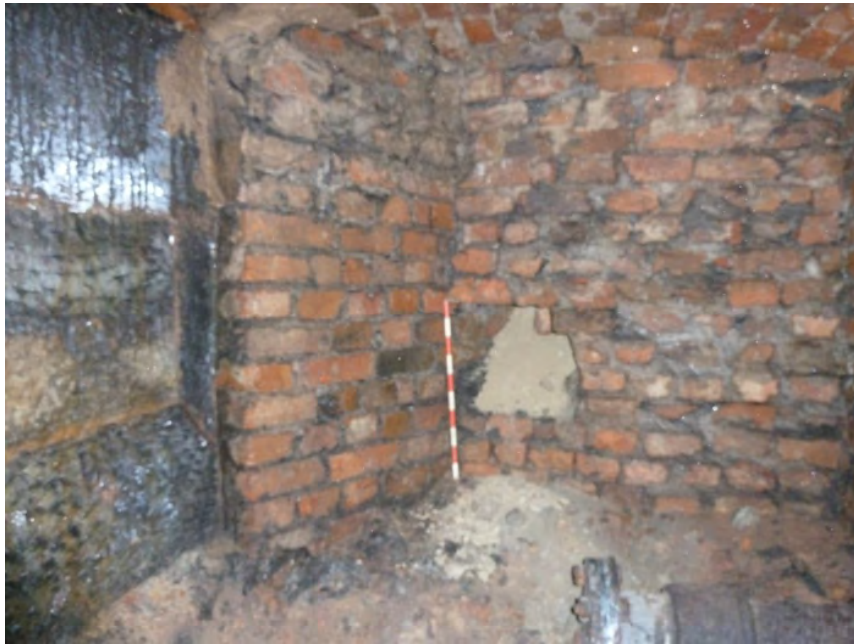
Figure 83: Southern and eastern walls in Room C1. Looking southeast.
