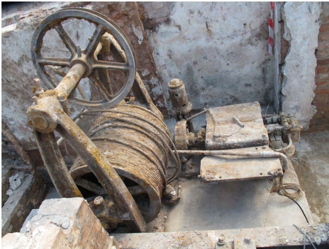
Figure 67: Mechanical remains of lift within lift shaft, Room B15.
