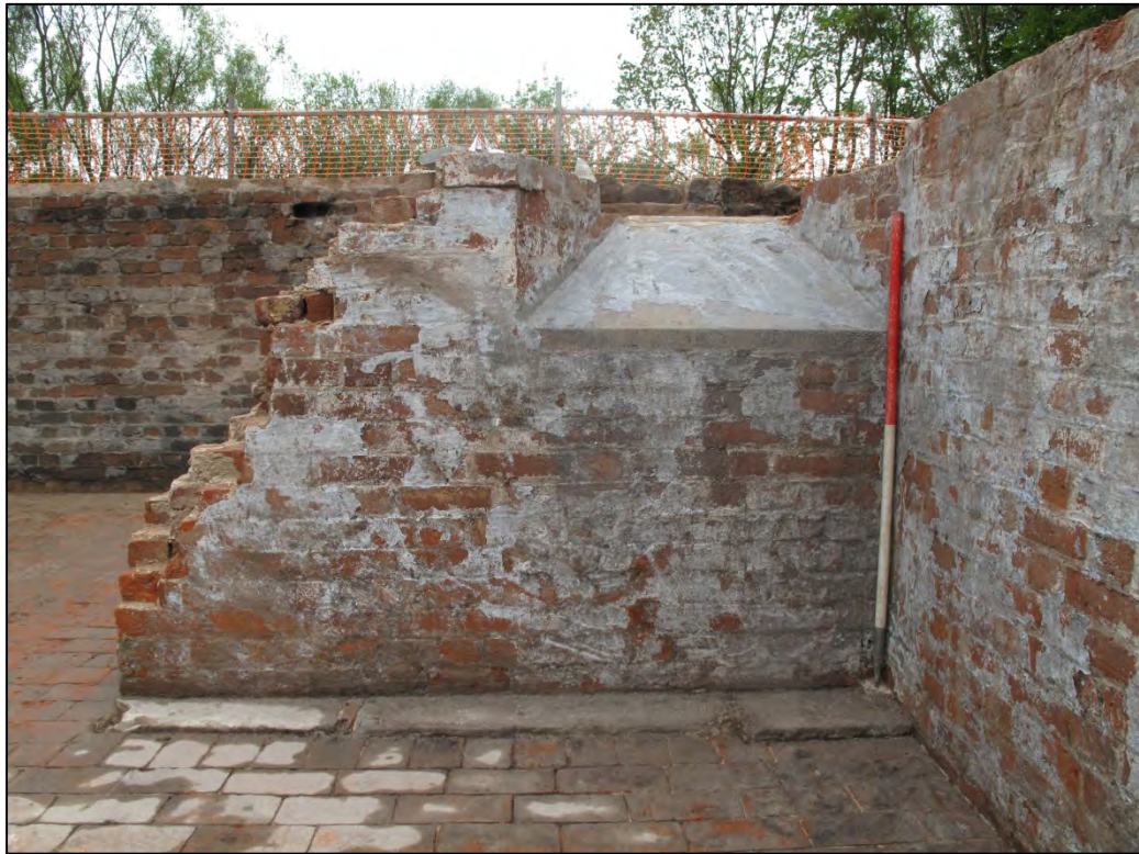
Figure 23: Detail of tapered sandstone window sill in southern wall (004) of Room B5, looking south.
