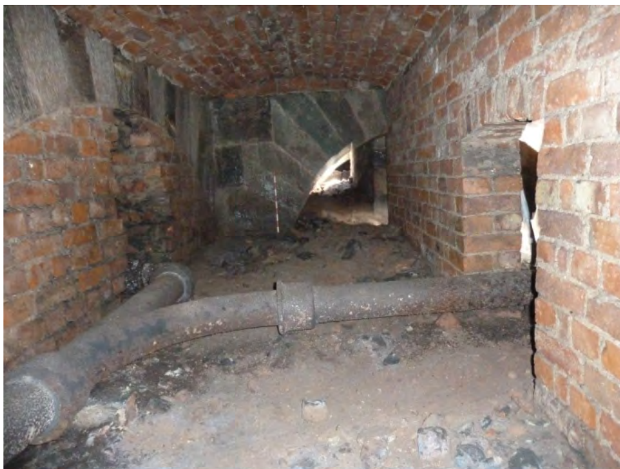
Figure 88: Room C4 looking north.
