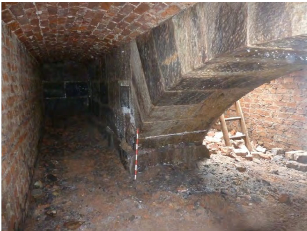
Figure 99: Stone archway in Room C16. Looking southwest.
