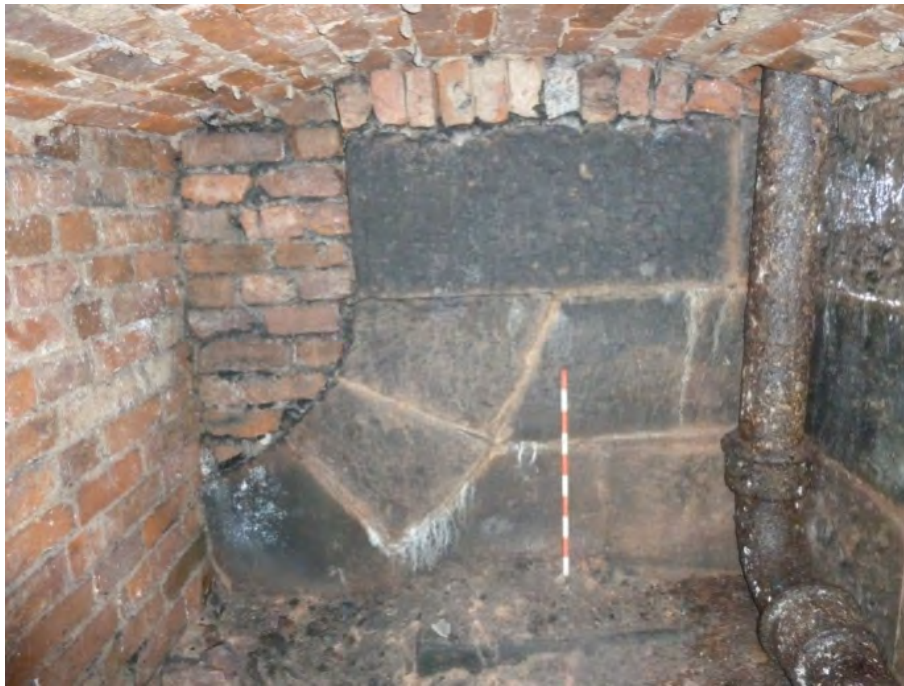
Figure 87: Southern wall in Room C4.
