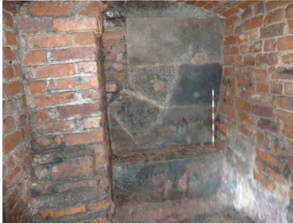
Figure 103: Southern end of Room C22. Looking east.
