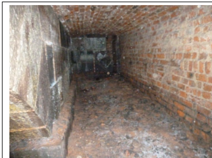
Figure 100: Southern end of Room C19. Looking south.
