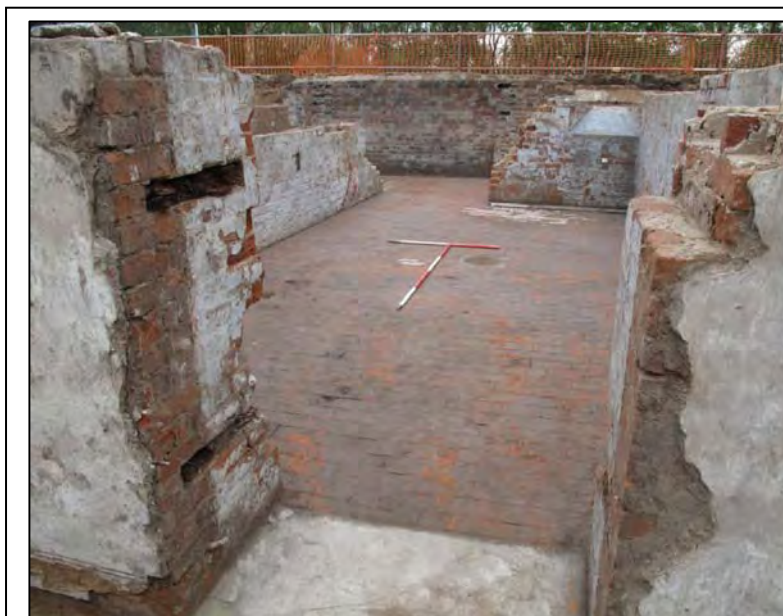
Figure 20: Room B5, looking south.
