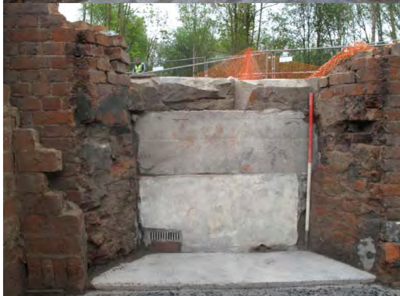
Figure 73: Blocked up cellar light (276) within wall (277), Room B16.
