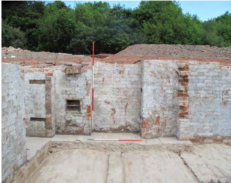
Figure 31: Detail of drain pipe (079) within floor of B7a, looking north.
