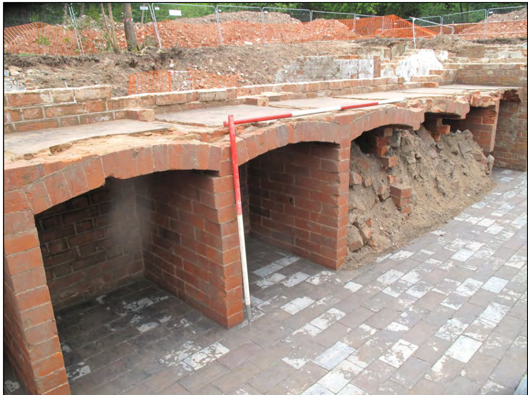
Figure 13: Storage bays (006) within Room 3, looking northwest.
