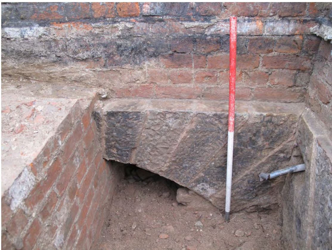
Figure 64: Ashlar stone archway (242 ) within the sub-basement beneath Room B14.
