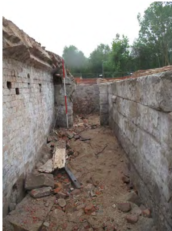
Figure 79: Room B22 looking west.
