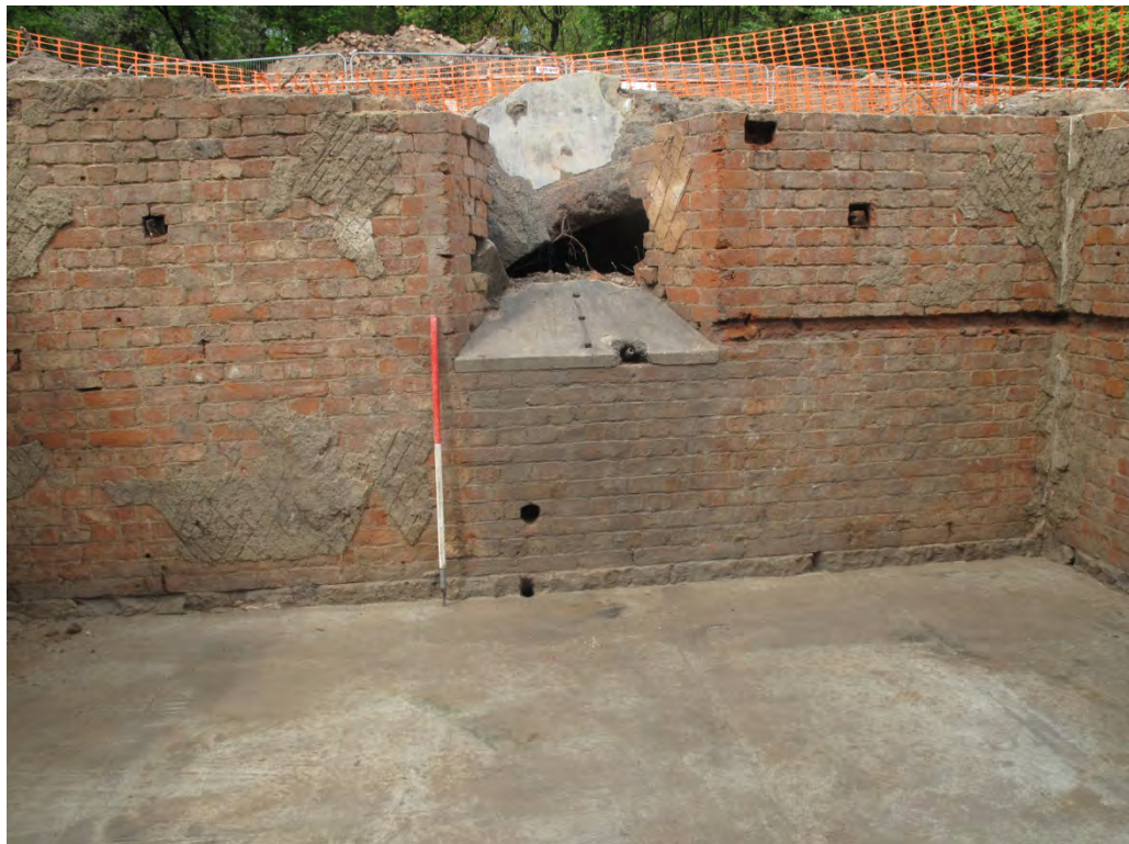
Figure 76: Blocked up cellar light within room B18.
