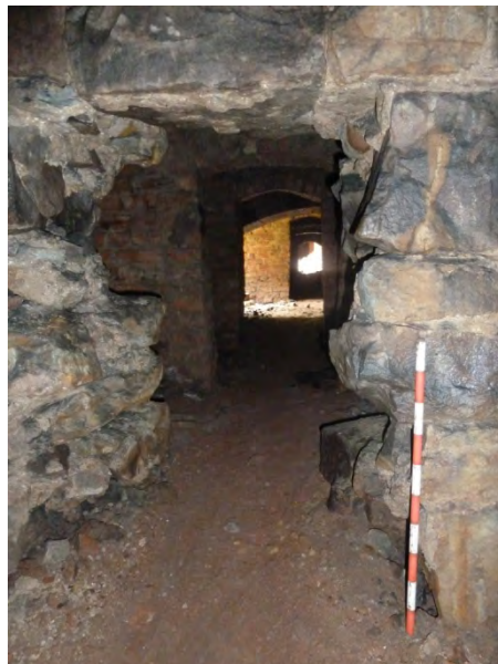
Figure 94: Western stone wall in Room C11. Looking west.
