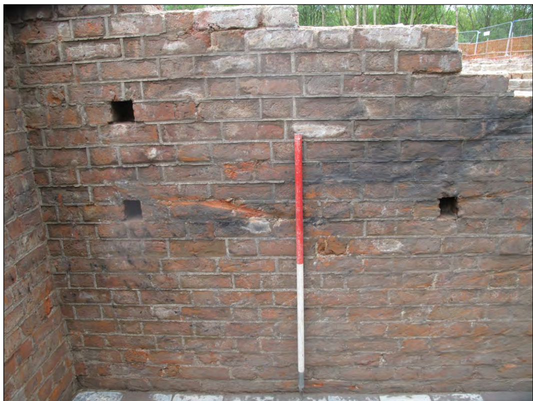
Figure 14: Voids within the eastern wall (005) within Room 3, looking east.
