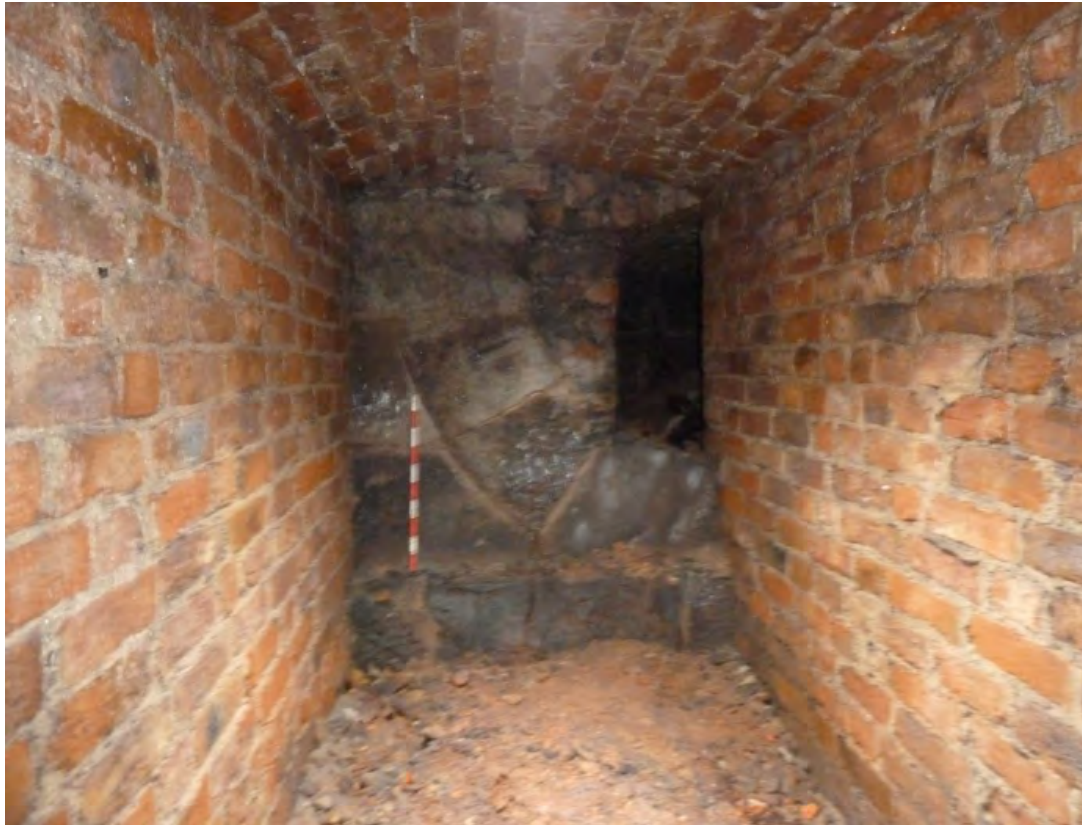
Figure 92: Shot of southern wall in Room C10. Looking south.
