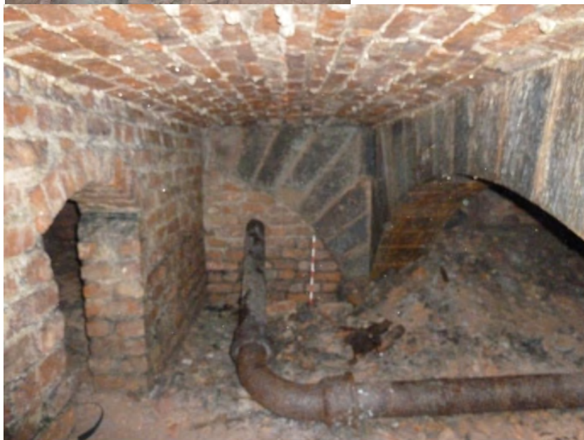
Figure 91: Pipe running into brick blocking in Room C7. Looking north.
