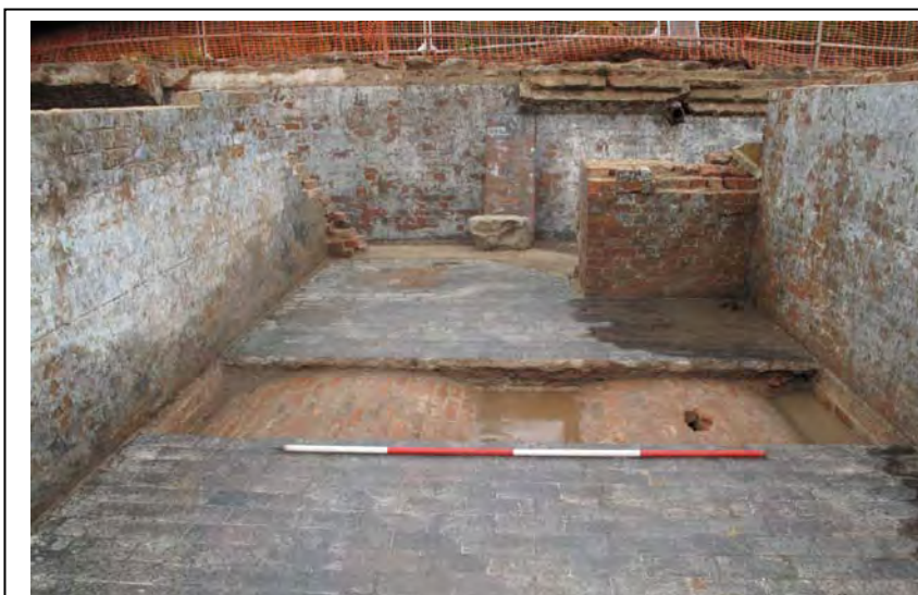
Figure 36: Detail of brick vaulted ceilings (150) below the floor (149) of B8, looking south.
