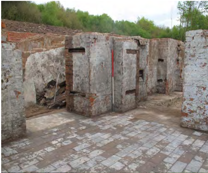
Figure 25: View of B6, looking north-east.
