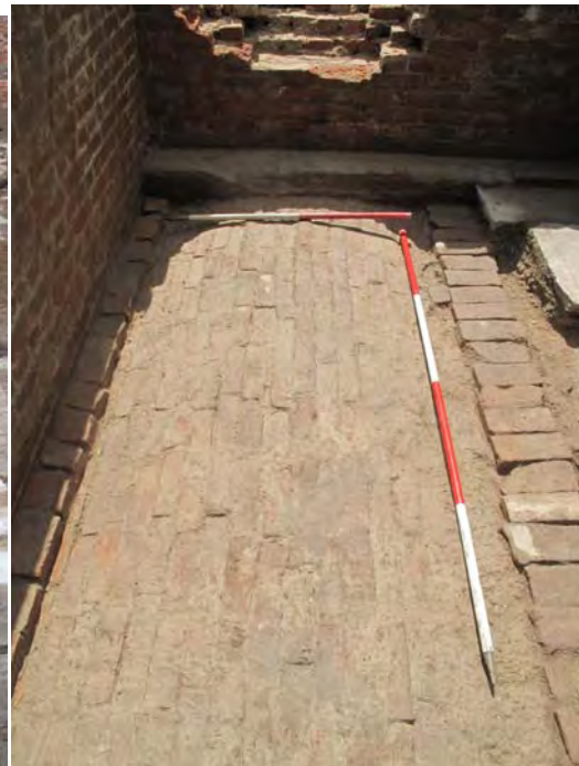
Figure 18: Vaulted ceiling of the sub basements (009) within Room B4.
