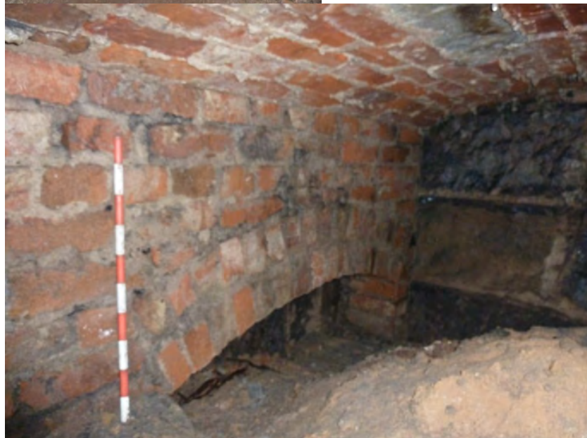
Figure 95: Small brick archway at southern end of Room C11.
