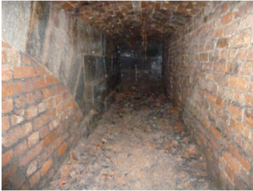
Figure 89: Southern end of Room C5. Looking south.
