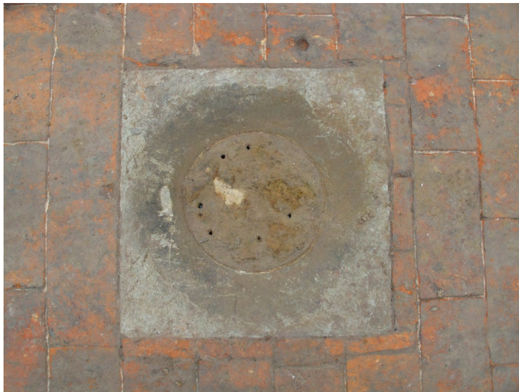
Figure 24: Detail of floor drain (072) in floor of Room B5 looking north.
