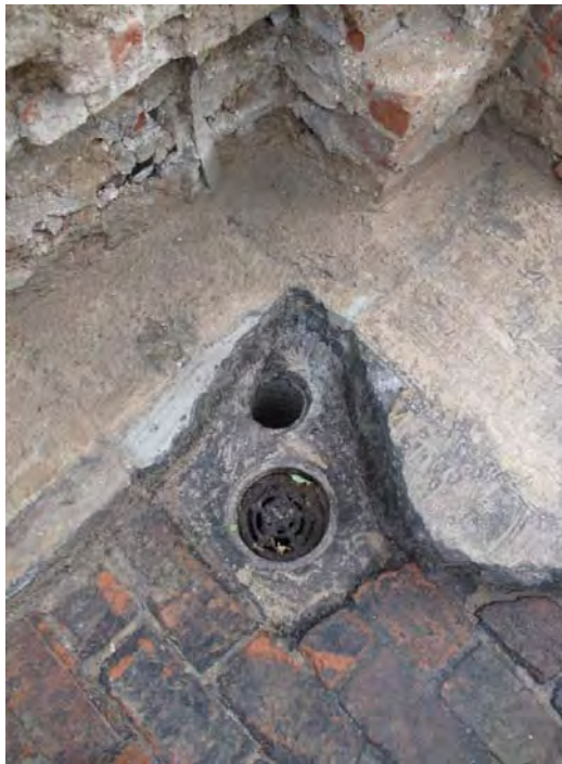
Figure 5: Detail of drain (146) within the east/west wing of Corridor 5, looking north-east.
