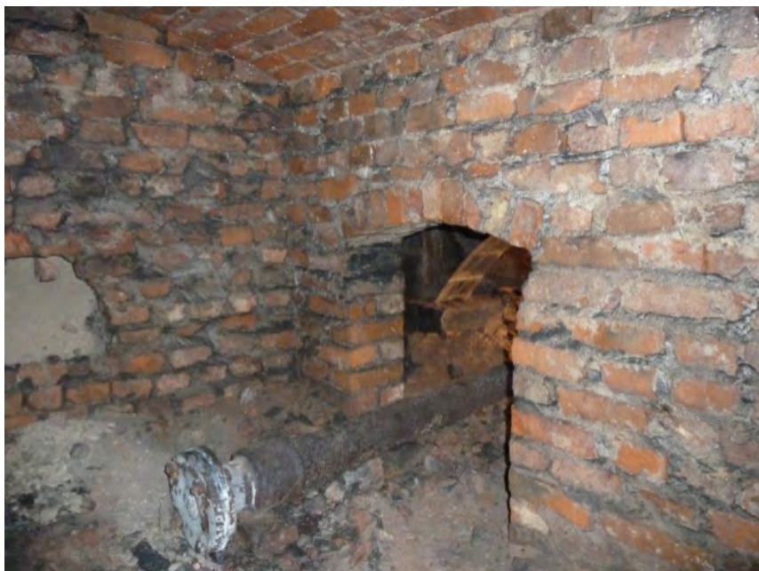
Figure 84: Shot of southern and southwestern walls in Room C1. Looking southwest.
