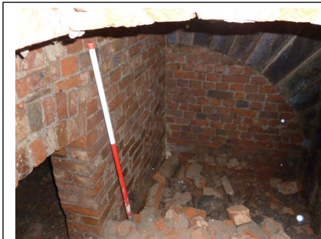
Figure 105: Room C25. Looking north.
