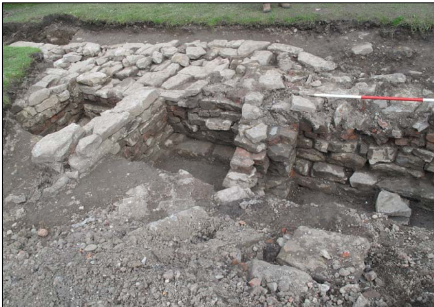
Fig. 10: Wall (099) showing abutting walls (107), (106), (105). Looking south.
